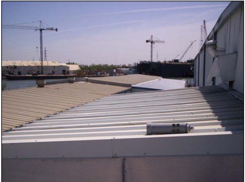
7. Overview of roof (area B).
