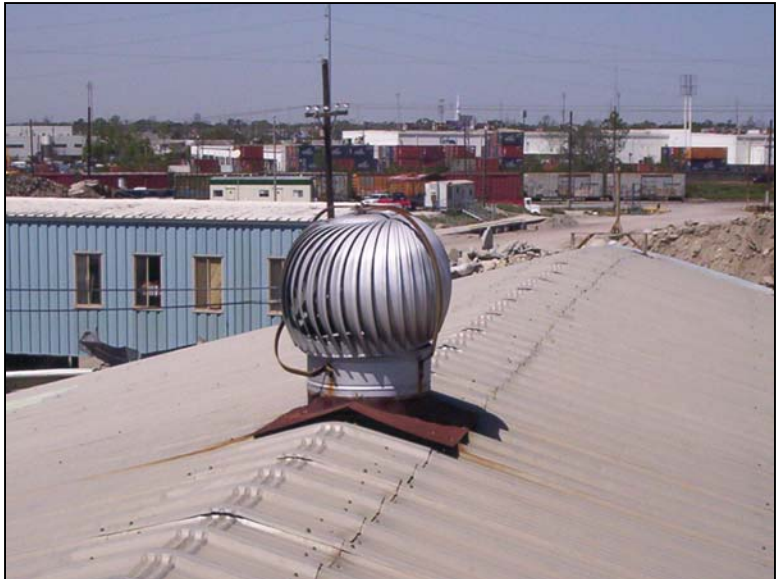
1. Overview of roof (area A).
