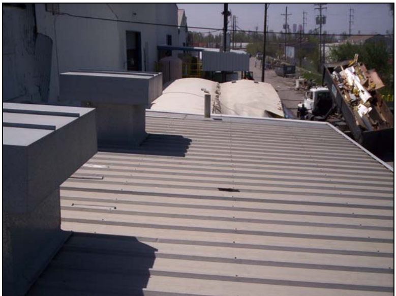
8. Overview of roof (area C).
