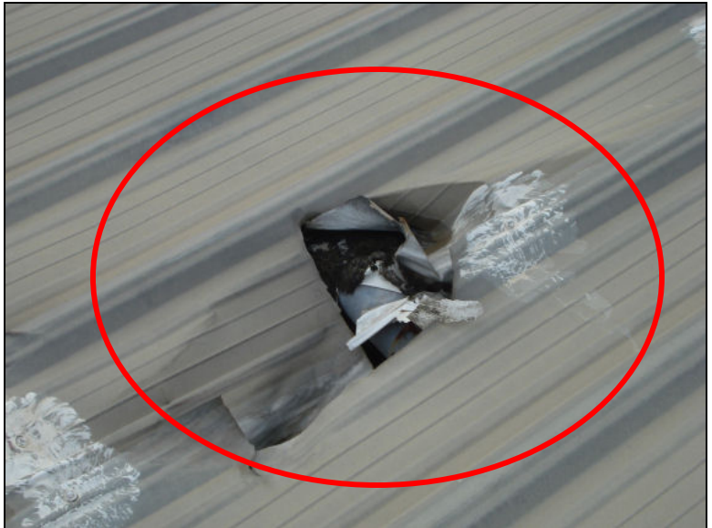
7. Hole from flying debris.
