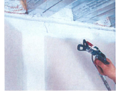
The head-of-wall construction joint is sprayed with fire resistive sealant.
