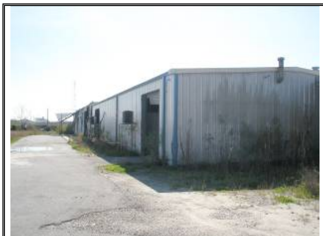
Photograph No. 059: north side of bldg 5
