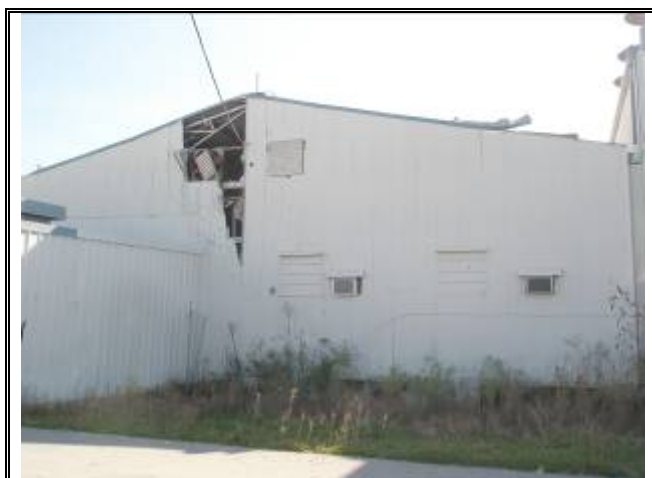
Photograph No. 048: west side of bldg 4
