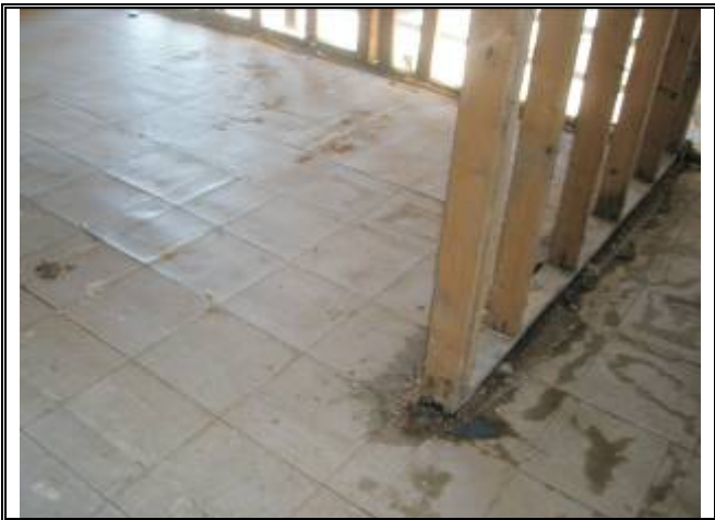
Photograph No. 008: inside downstairs of bldg 1
