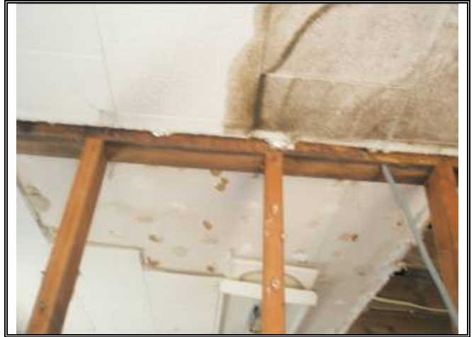
Photograph No. 010: inside downstairs of bldg 1
