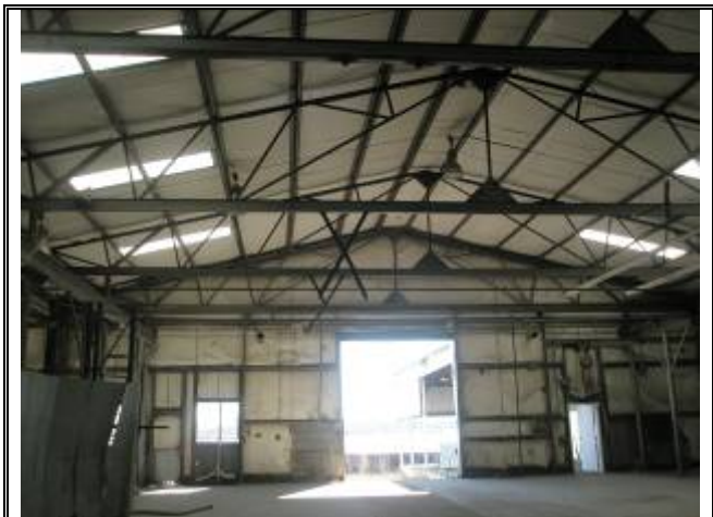
Photograph No. 055: inside of bldg 4
