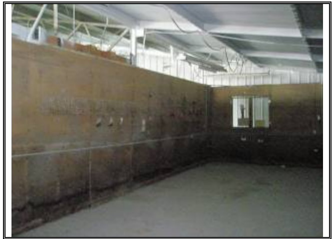
Photograph No. 029: inside storage shed of bldg 2
