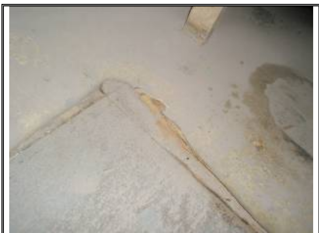
Photograph No. 057: inside bathroom of bldg 4
