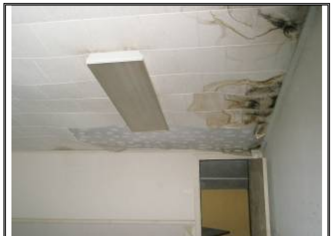
Photograph No. 012: inside upstairs of bldg 1
