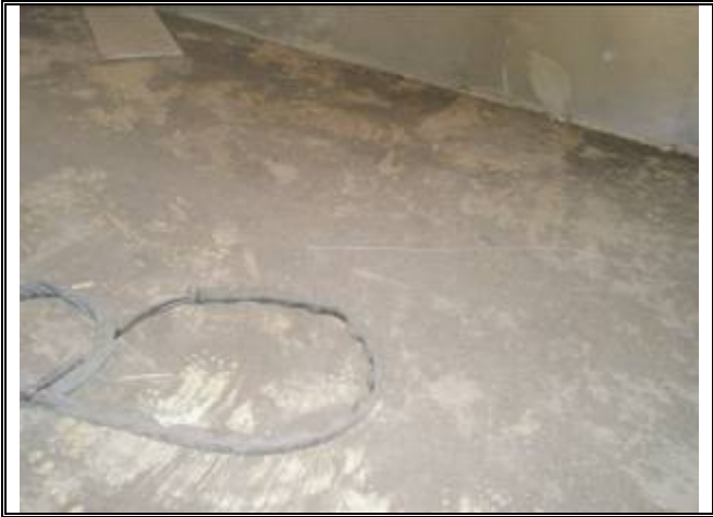
Photograph No. 025: inside upstairs offices of bldg 2
