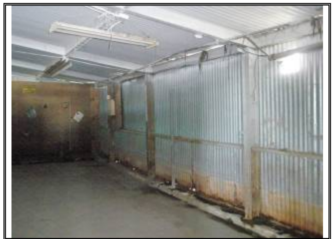
Photograph No. 030: inside storage shed of bldg 2
