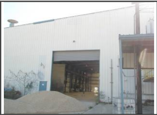
Photograph No. 032: west side of bldg 3
