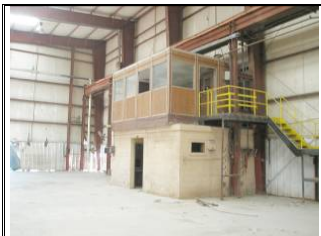
Photograph No. 042: inside of bldg 3
