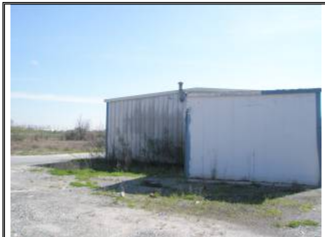
Photograph No. 058: west side of bldg 5
