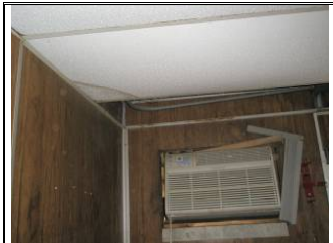
Photograph No. 046: inside upstairs office of bldg 3
