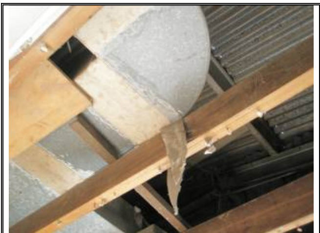
Photograph No. 009: inside downstairs of bldg 1
