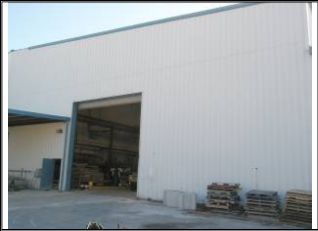
Photograph No. 031: west side of bldg 3
