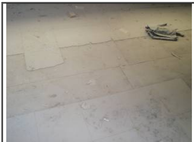
Photograph No. 047: inside upstairs office of bldg 3
