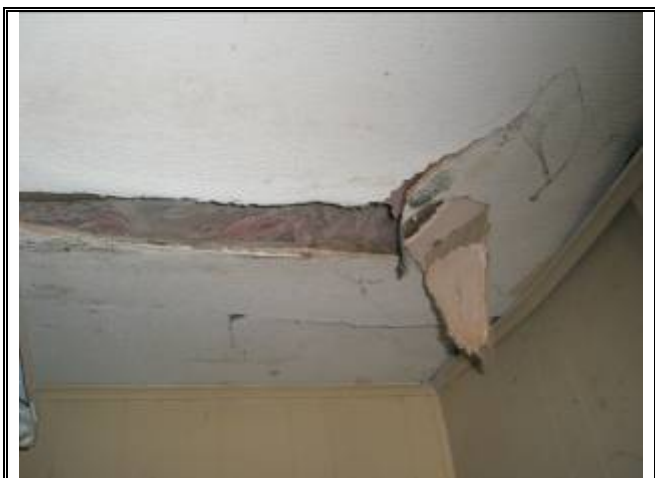
Photograph No. 056: inside bathroom of bldg 4
