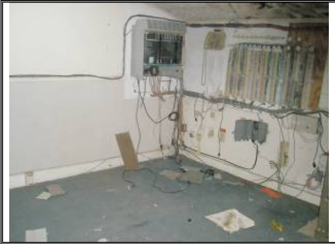
Photograph No. 013: inside upstairs of bldg 1
