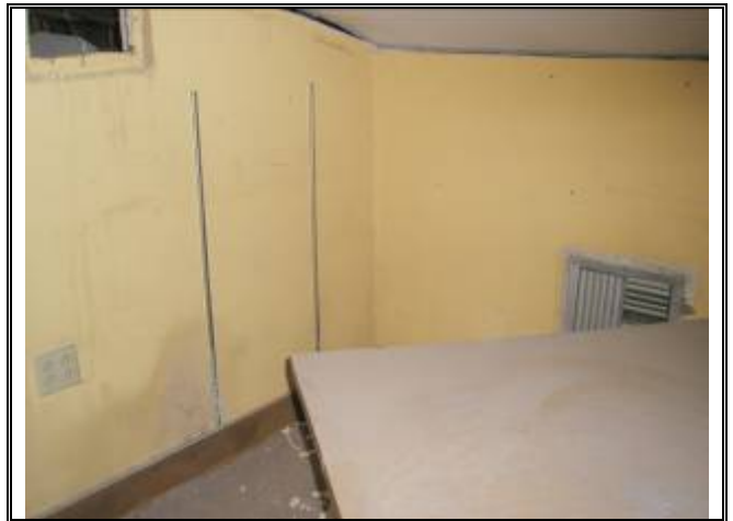
Photograph No. 011: inside upstairs of bldg 1
