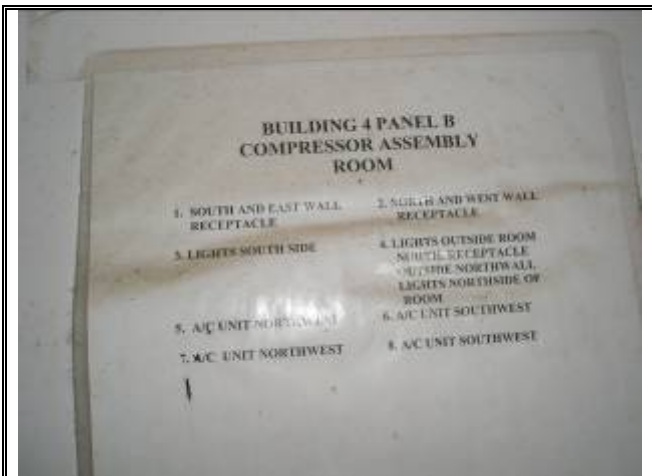
Photograph No. 050: inside compressor room of bldg 4
