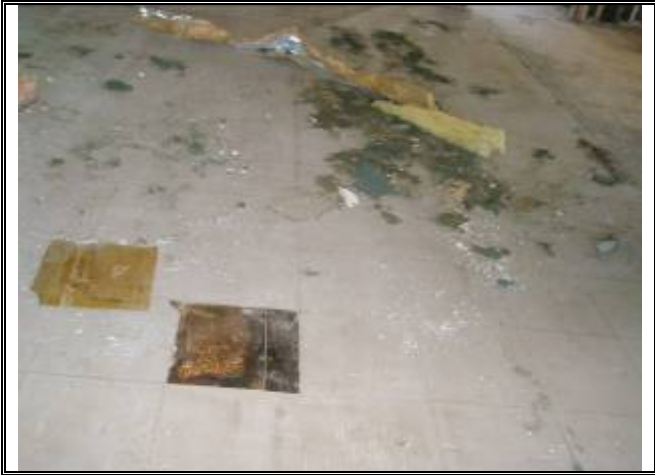
Photograph No. 007: inside downstairs of bldg 1
