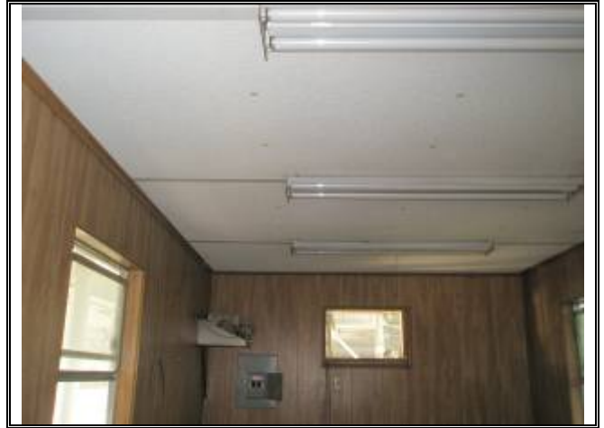
Photograph No. 022: inside upstairs offices of bldg 2
