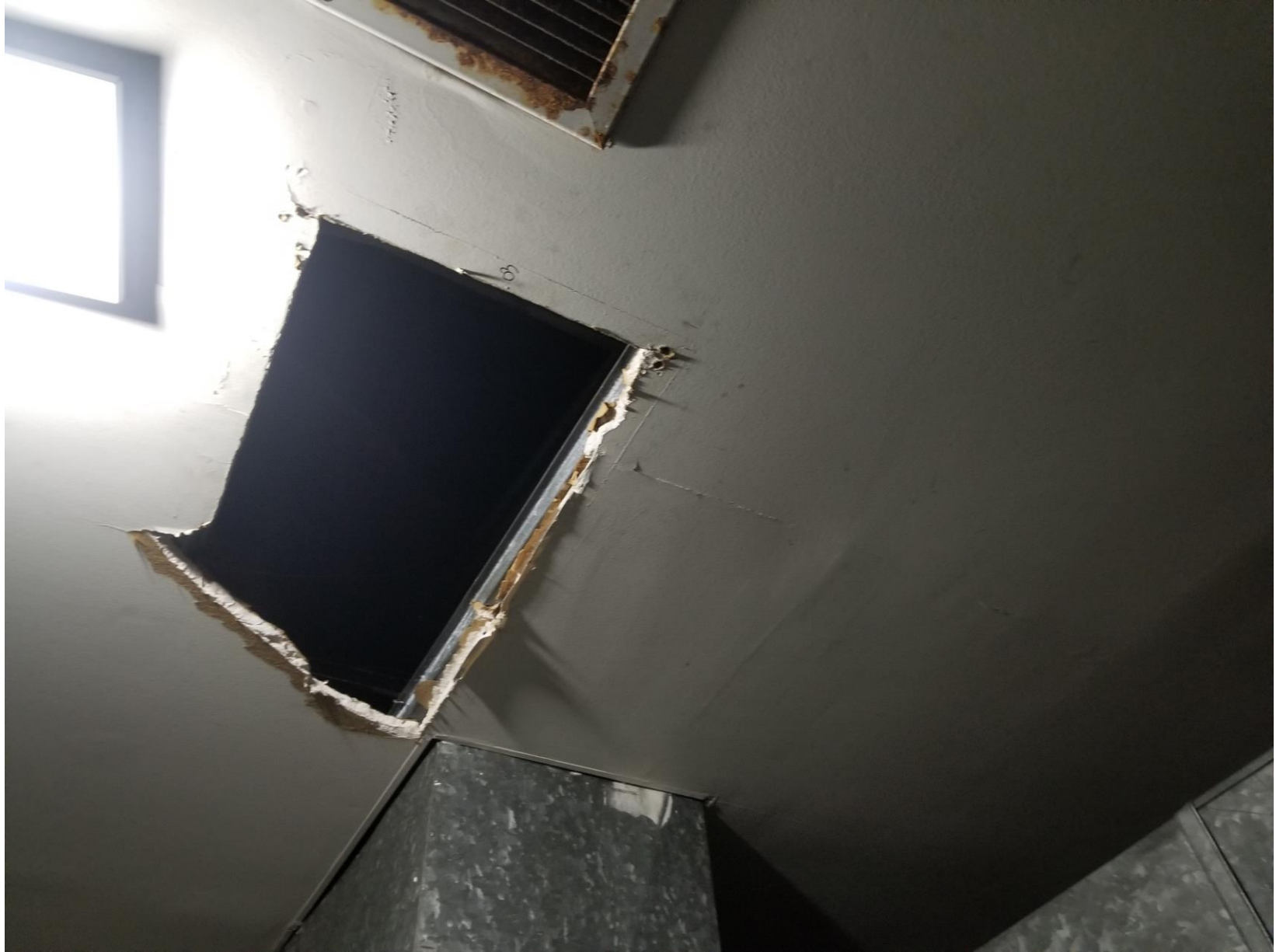
View of HA-02: White drywall and joint compound.
