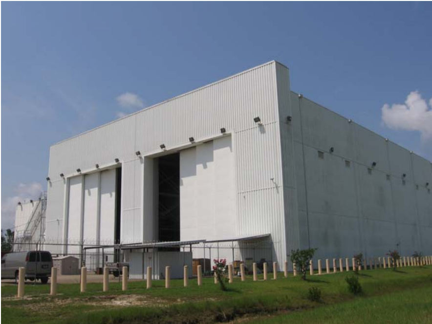
Building B3202 – North and East side
