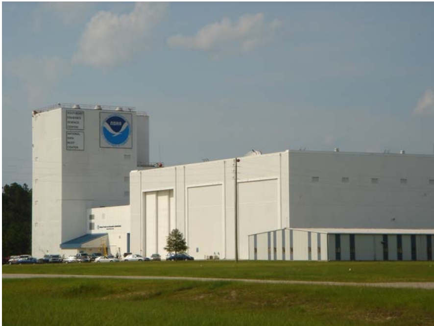
Building B3203 – West side
