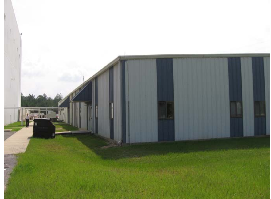
Building B3205 – North and West side
