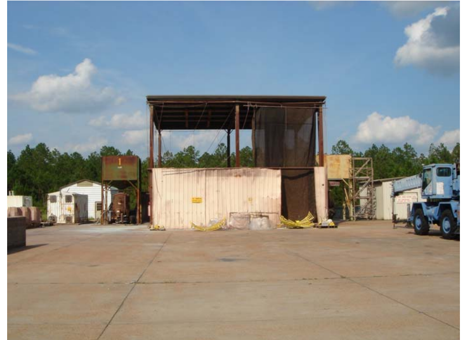
Building B3209 – West side
