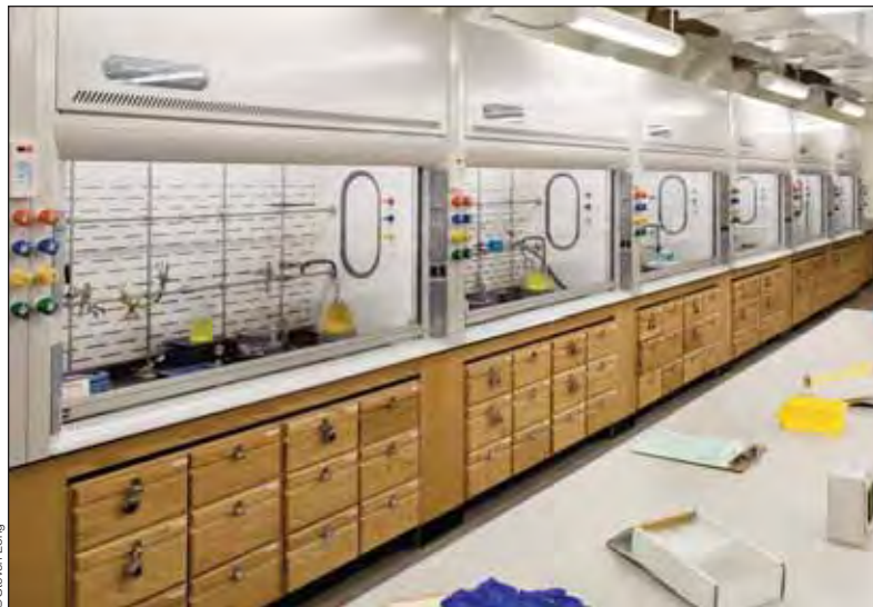
At the Rochester Institute of Technology, each Protector XStream Laboratory Hoods is outfitted with eight service fixtures, including a gooseneck faucet.
