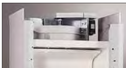
The built-in blower in this Protector Premier Laboratory Hood is visible when the front panel is removed.
