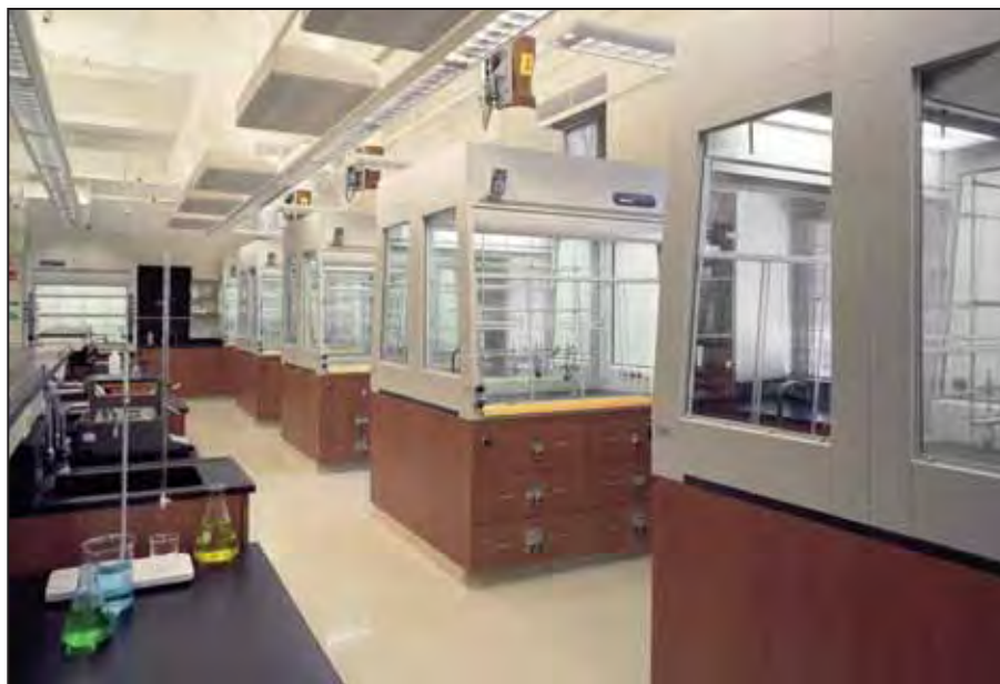
Transparent glass backs and baffles provide a clear view through these Protector ClassMate Combination Sash Laboratory Hoods mounted back-to-back on peninsular casework at this university laboratory.
