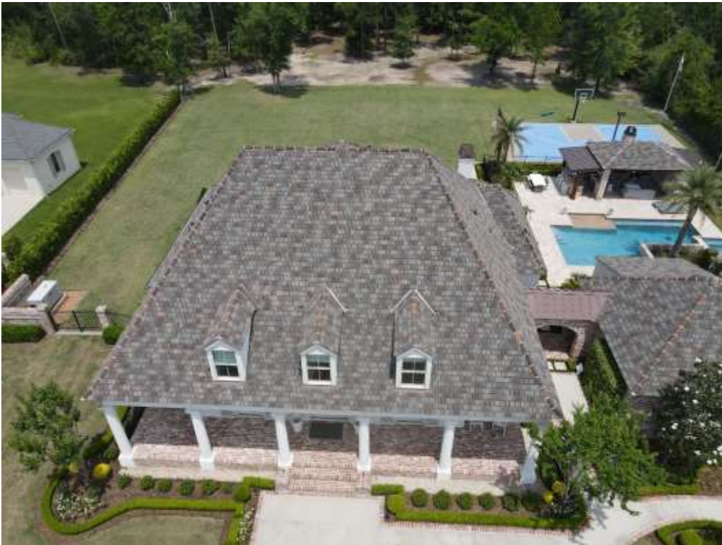
Photograph #5 – Drone view of the various roof slopes over the residence.
