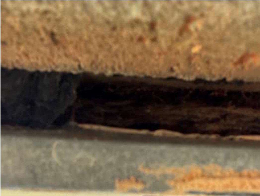
Photograph #4 – View of the exterior building material behind the stucco-finished walls.
