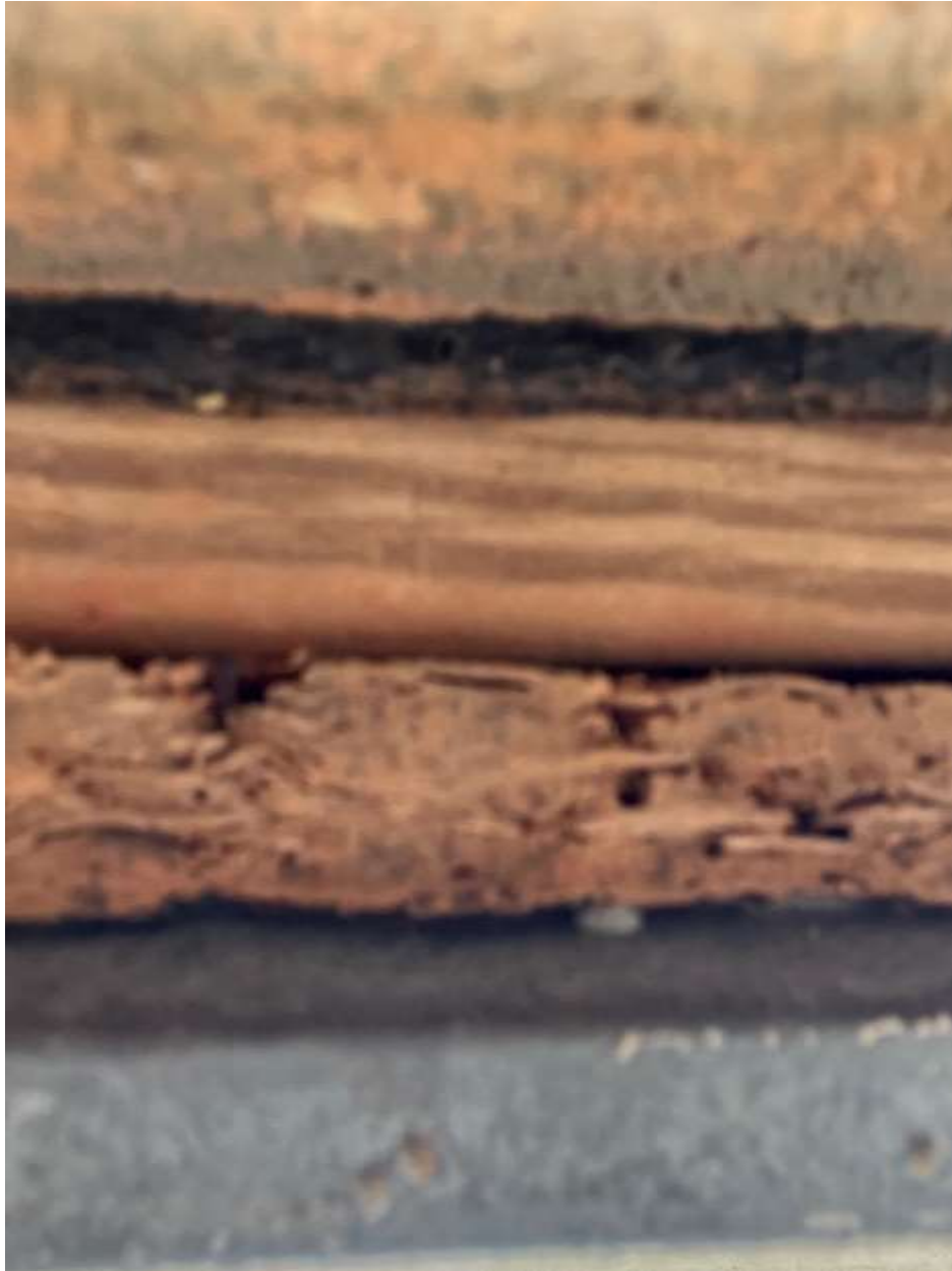
Photograph #3 – View of the exterior building material behind the stucco-finished walls.
