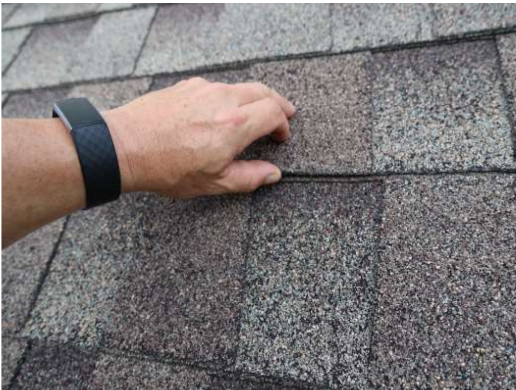
Photograph #7 – View of the asphalt shingles (original inspection).
