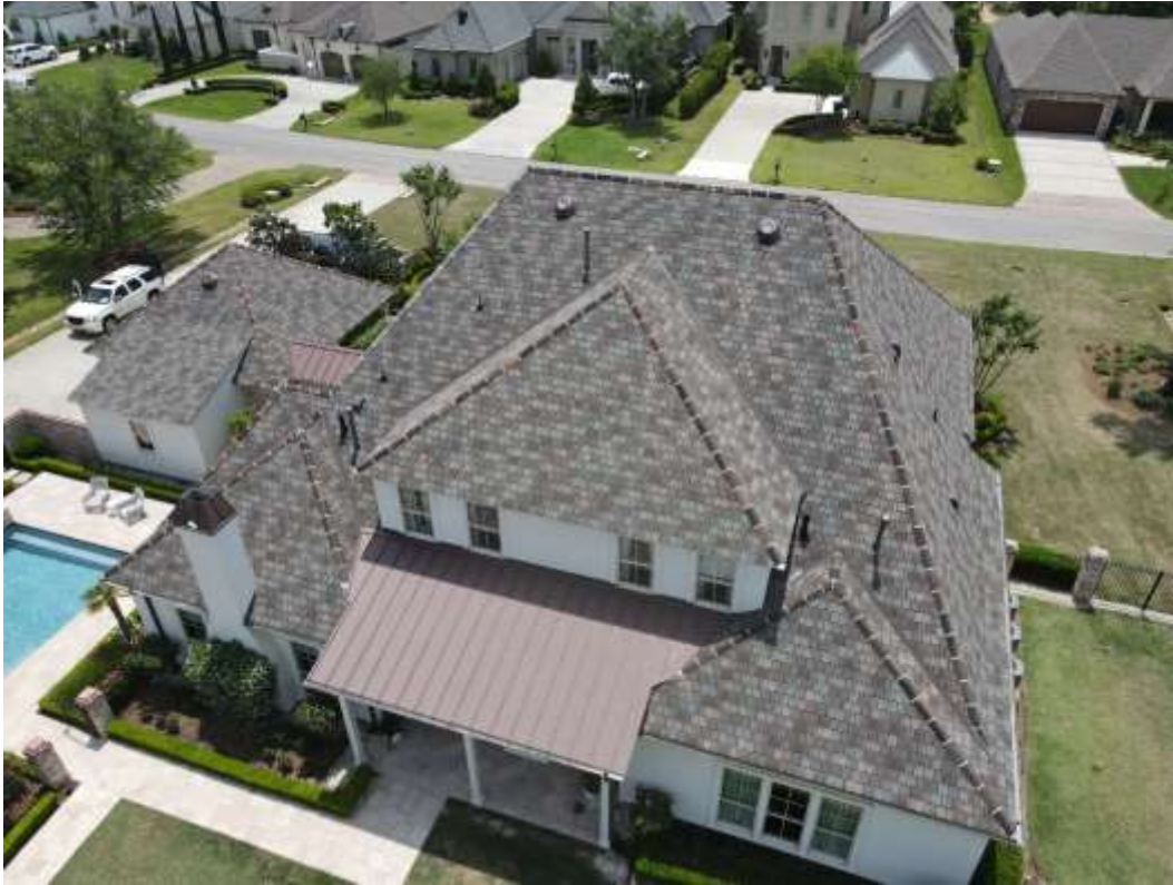
Photograph #6 – Drone view of the various roof slopes over the residence.
