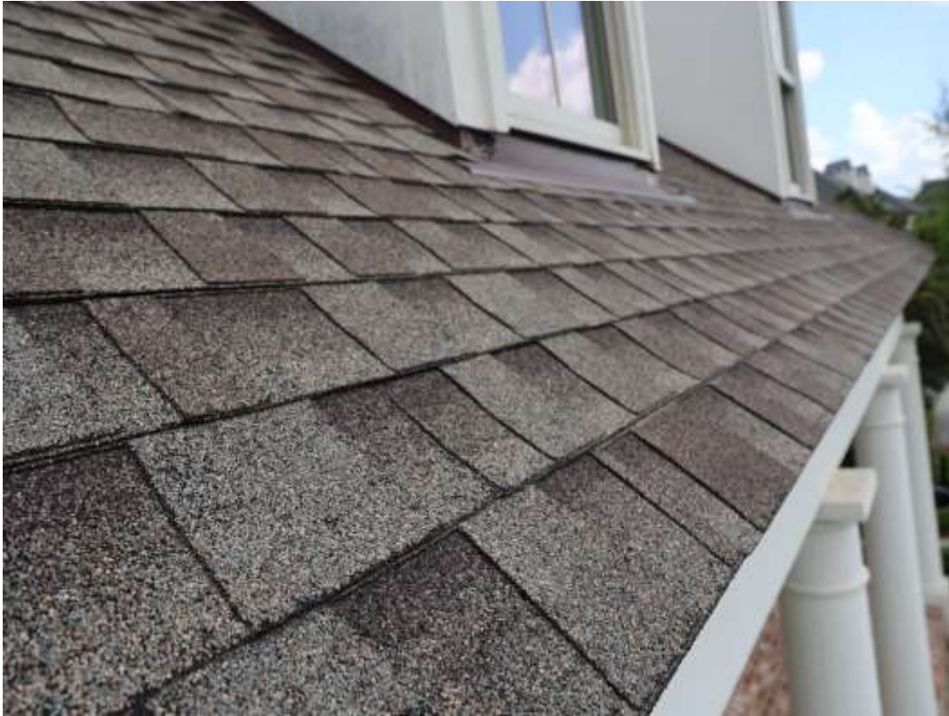
Photograph #8 – View of the asphalt shingles (original inspection).
