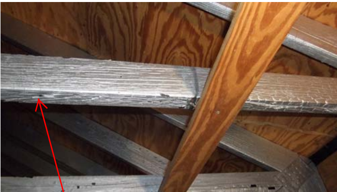
Roof framing member that has been painted.
