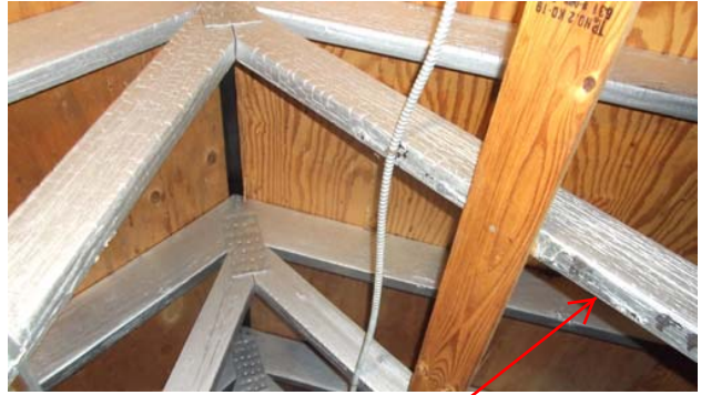
Roof framing members that have been painted.
