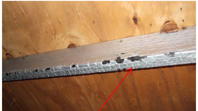
Roof framing member that has been painted.
