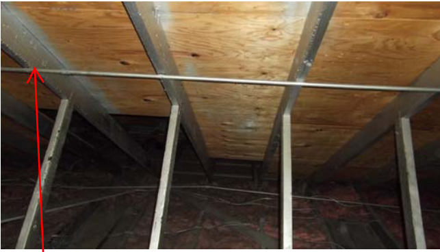
Roof framing members that have been painted.
