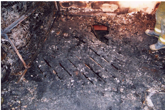
Figure 1 Hole burned through hardwood floor and subfloor underneath a mattress fire (Courtesy Lew Kingman)
