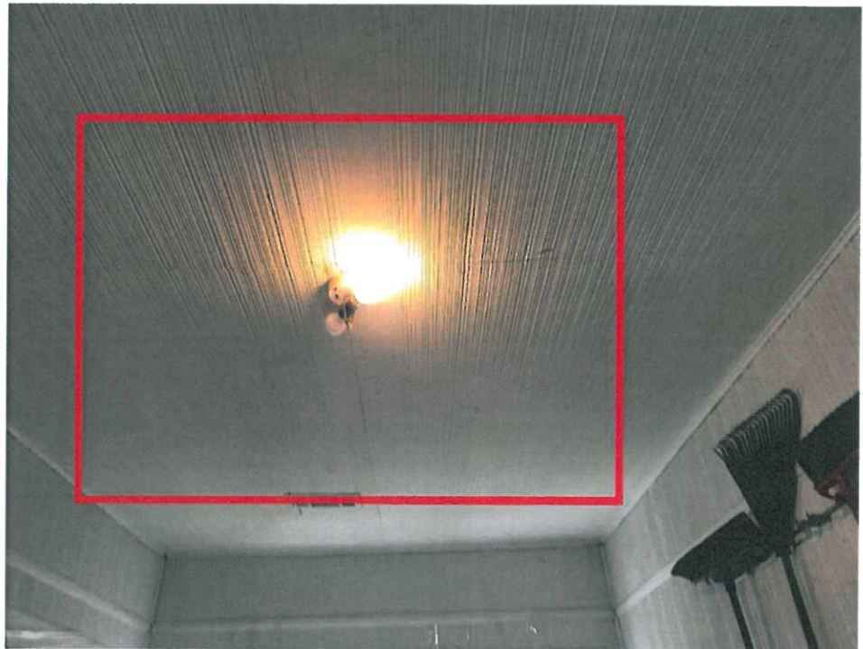
231 Main Level/Sun room - 214-214- Jan 31 2022 04_25pm-k7Cd Date Taken: 1/31/2022
