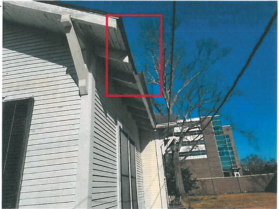
85 Dwelling Exterior/Right Elevation - 5-5-Jan 31 2022 03_41pm-zayW Date Taken: 1/31/2022
