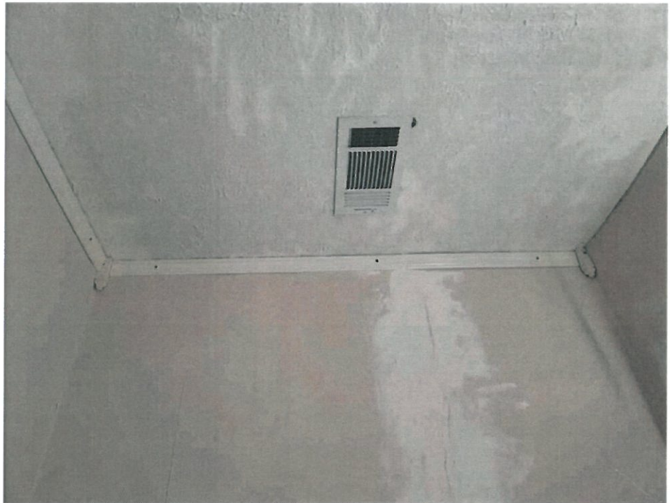
193 Main Level/Bathroom - 171-171- Jan 31 2022 04_22pm-5MHJ Date Taken: 1/31/2022
