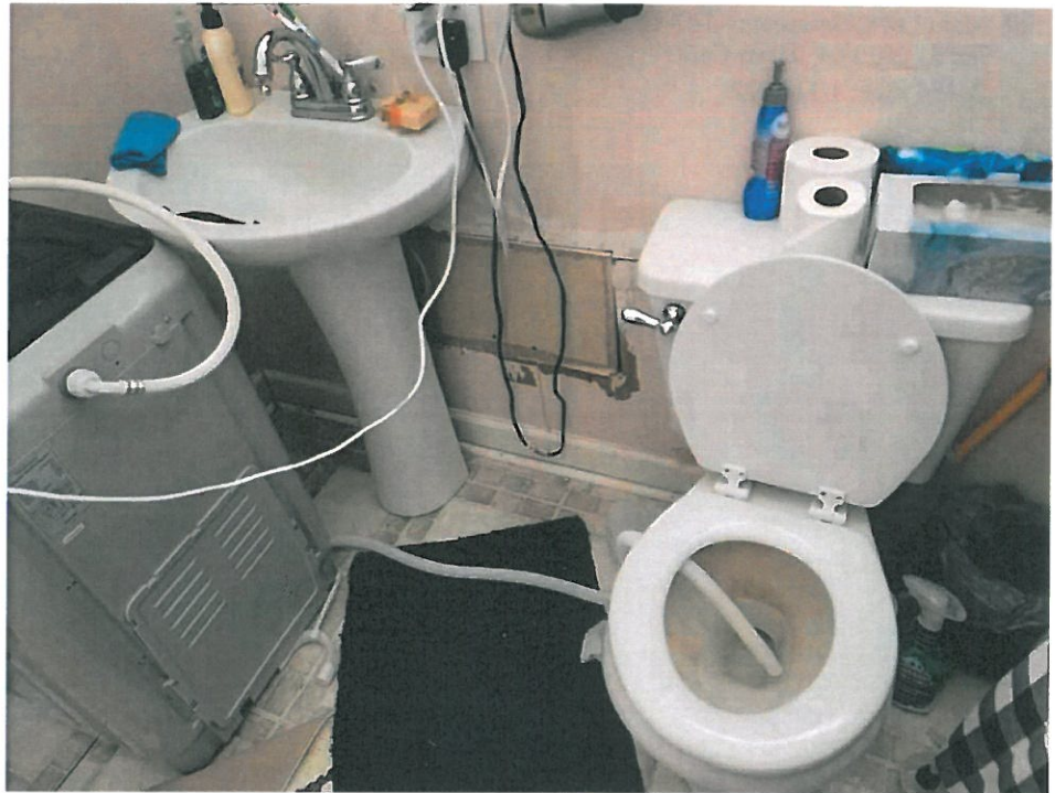
191 Main Level/Bathroom - 169-169- Jan 31 2022 04_22pm-p64a Date Taken: 1/31/2022
