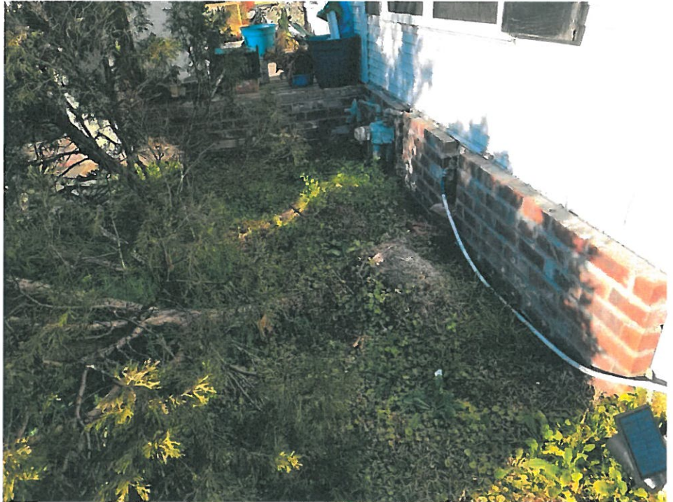
86 Main Level - 8-8-Jan 31 2022 03_ 41pm-RfwA Date Taken: 1/31/2022
