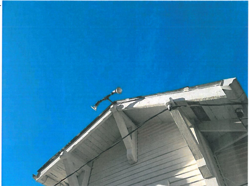
81 Dwelling Exterior/Right Elevation - 49-49-Jan 31 2022 03_47pm-52nb Date Taken: 1/31/2022
