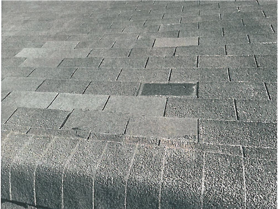
14 Roof/Roof - 66-66-Jan 31 2022 03_ 50pm-Cx1N Date Taken: 1/31/2022
