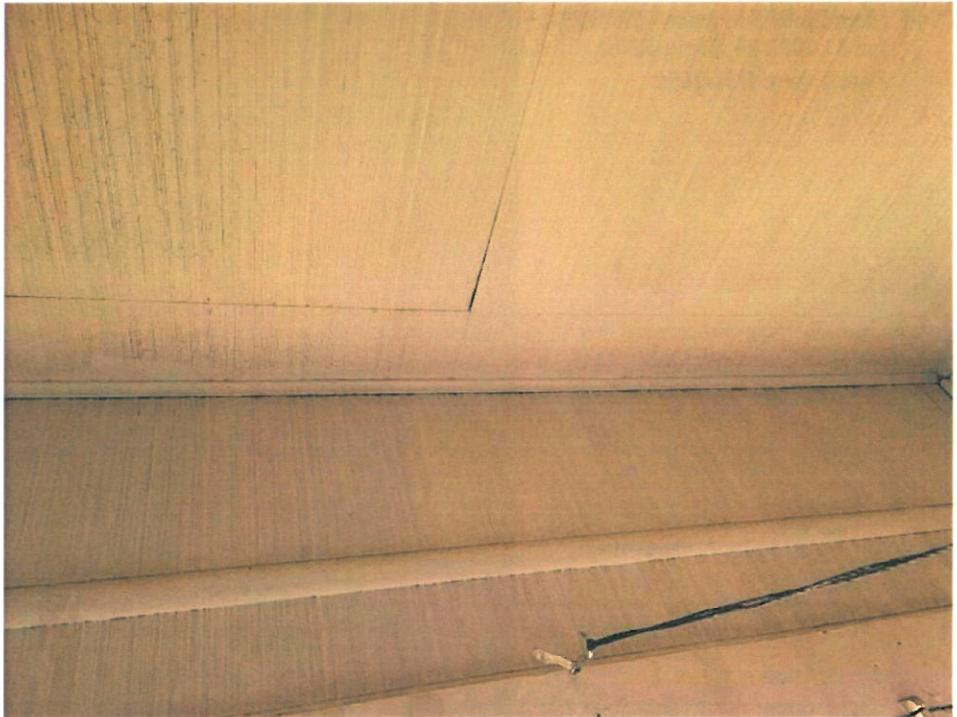
242 Main Level/Sun room - 225-225- Jan 31 2022 04_25pm-N8MZ Date Taken: 1/31/2022
