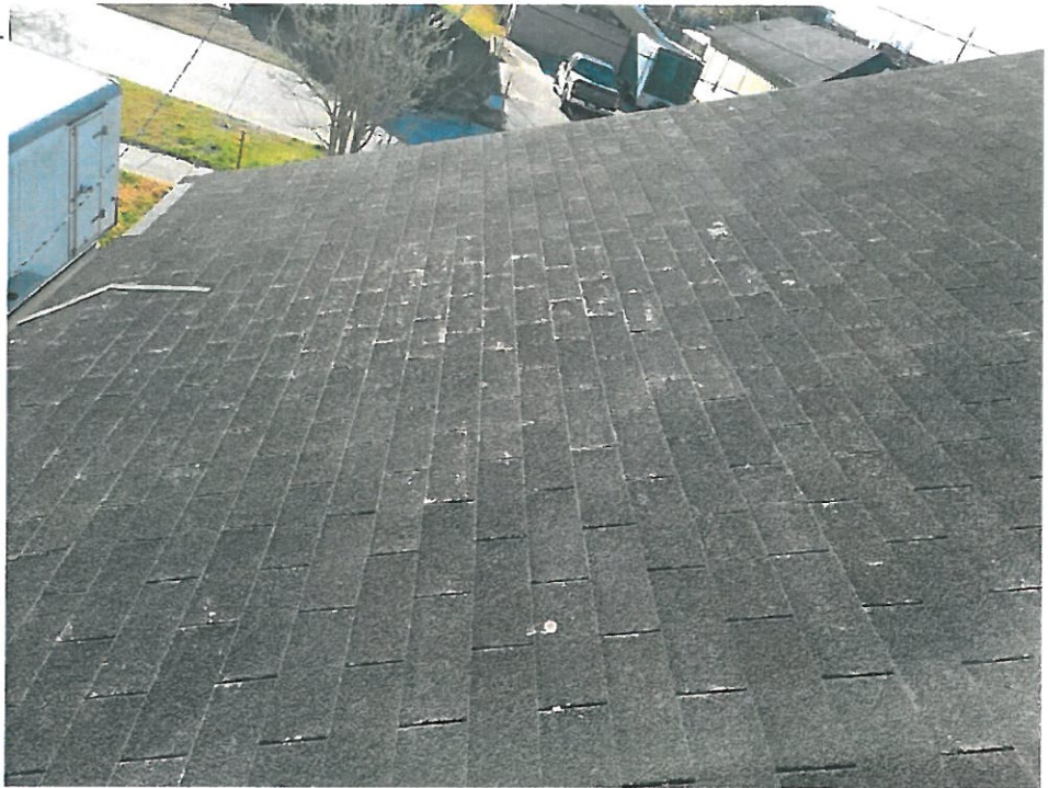
23 Roof/Roof - 75-75-Jan 31 2022 03_51pm-qfVk Date Taken: 1/31/2022
