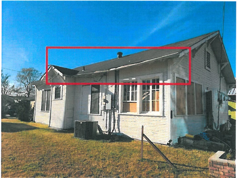
76 Dwelling Exterior/Rear Elevation - 44-44-Jan 31 2022 03_46pm- hpJW Date Taken: 1/31/2022
