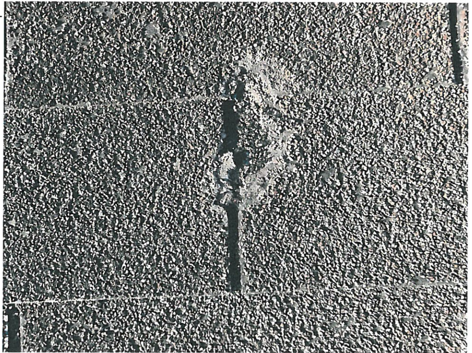
24 Roof/Roof - 76-76-Jan 31 2022 03_51pm-zAgK Date Taken: 1/31/2022
