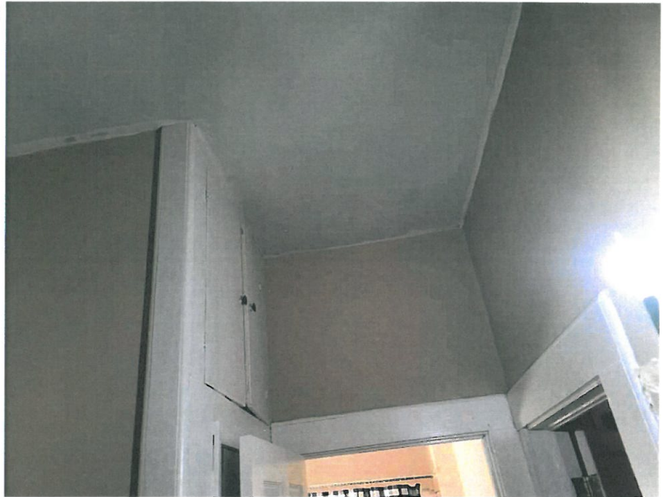
143 Main Level/Hallway - 208-208-Jan 31 2022 04_24pm-osMQ Date Taken: 1/31/2022
