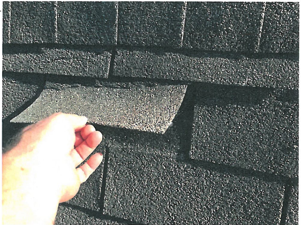
11 Roof/Roof - 63-63-Jan 31 2022 03_ 50pm-BrWC Date Taken: 1/31/2022
