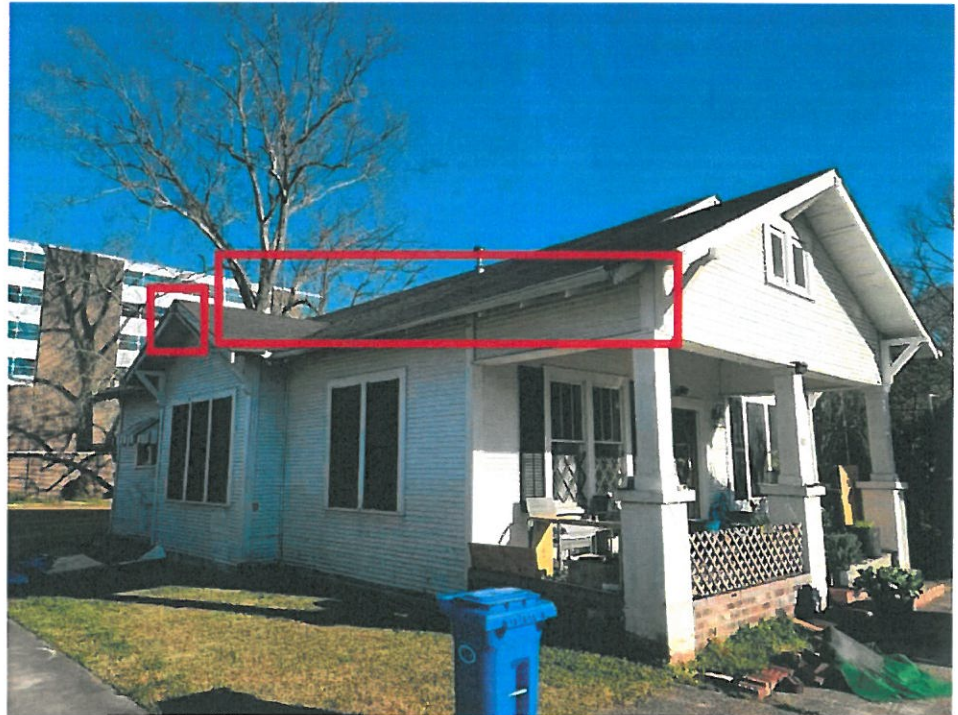
56 Dwelling Exterior/Left Elevation - 24-24-Jan 31 2022 03_43pm- K9iQ Date Taken: 1/31/2022
