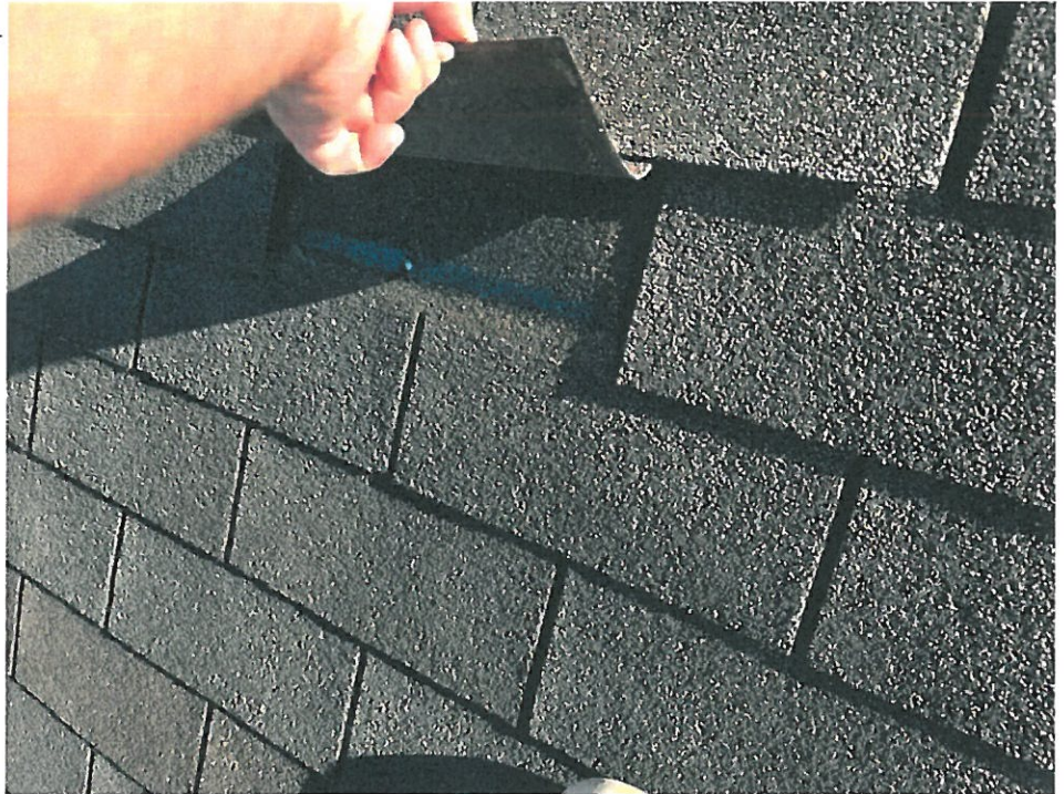
13 Roof/Roof - 65-65-Jan 31 2022 03_ 50pm-EV6m Date Taken: 1/31/2022
