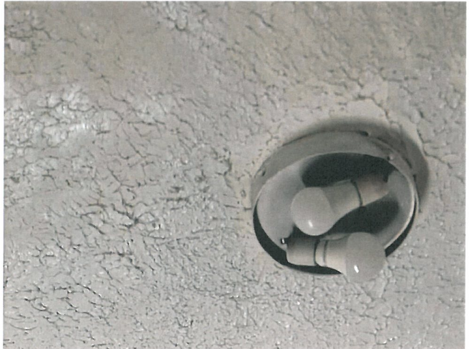
190 Main Level/Bathroom - 168-168- Jan 31 2022 04_21pm-GQZR Date Taken: 1/31/2022
