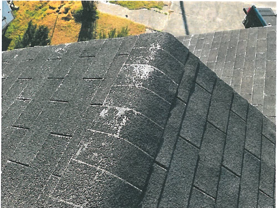
15 Roof/Roof - 67-67-Jan 31 2022 03_ 50pm-Ubp6 Date Taken: 1/31/2022
