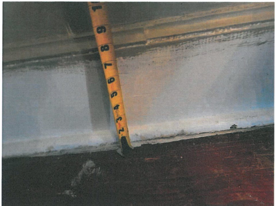
109 Main Level/Living Room - 113- 113-Jan 31 2022 04_14pm-4bvy Date Taken: 1/31/2022
