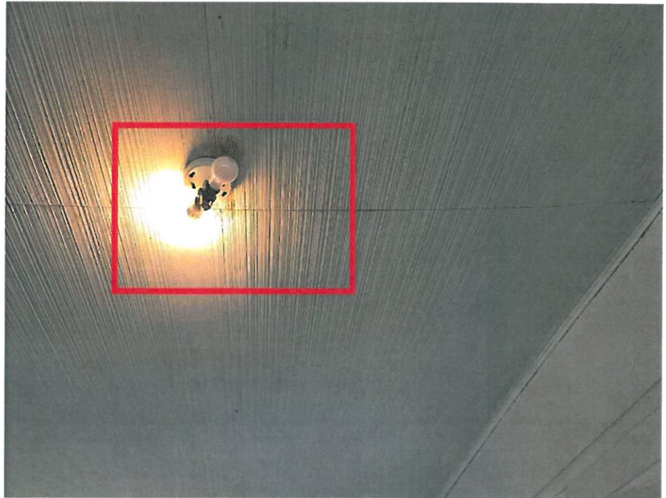
244 Main Level/Sun room - 227-227- Jan 31 2022 04_25pm-ENbe Date Taken: 1/31/2022
