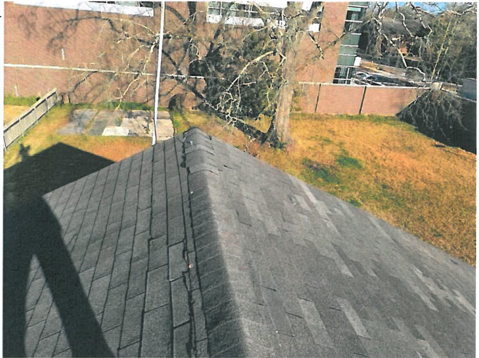
32 Roof/Roof - 84-84-Jan 31 2022 03_52pm-Ux3R Date Taken: 1/31/2022
