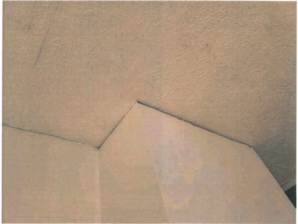
99 Main Level/Den - 103-103-Jan 31 2022 04_13pm-1Ep9 Date Taken: 1/31/2022
