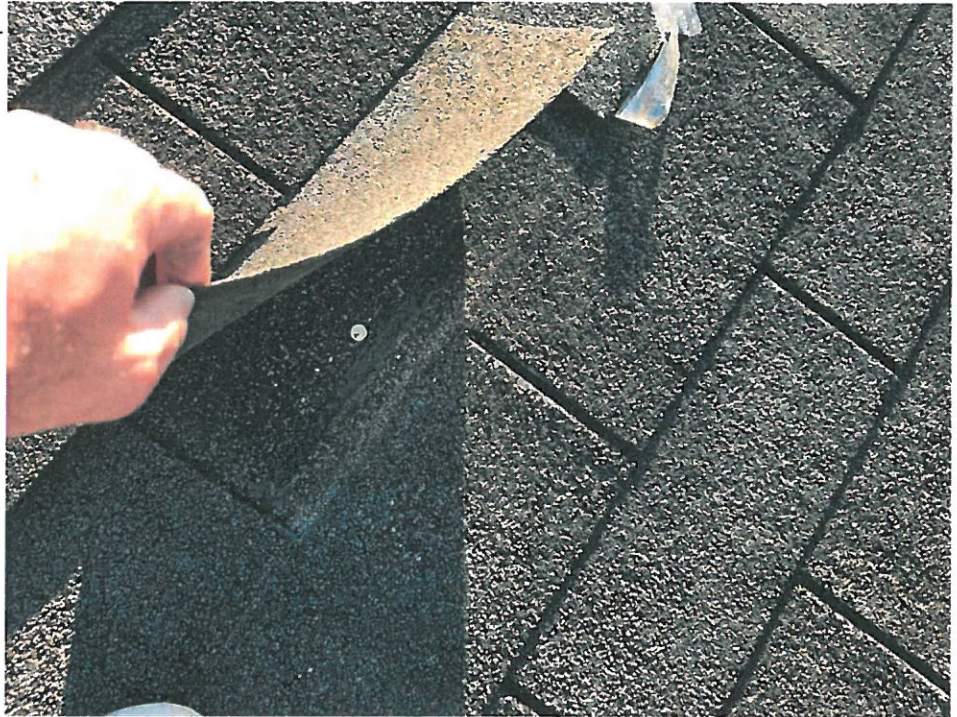
35 Roof/Roof - 87-87-Jan 31 2022 03_52pm-16FN Date Taken: 1/31/2022
