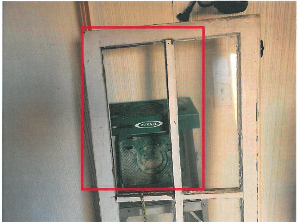
234 Main Level/Sun room - 217-217- Jan 31 2022 04_25pm-hdpc Date Taken: 1/31/2022
