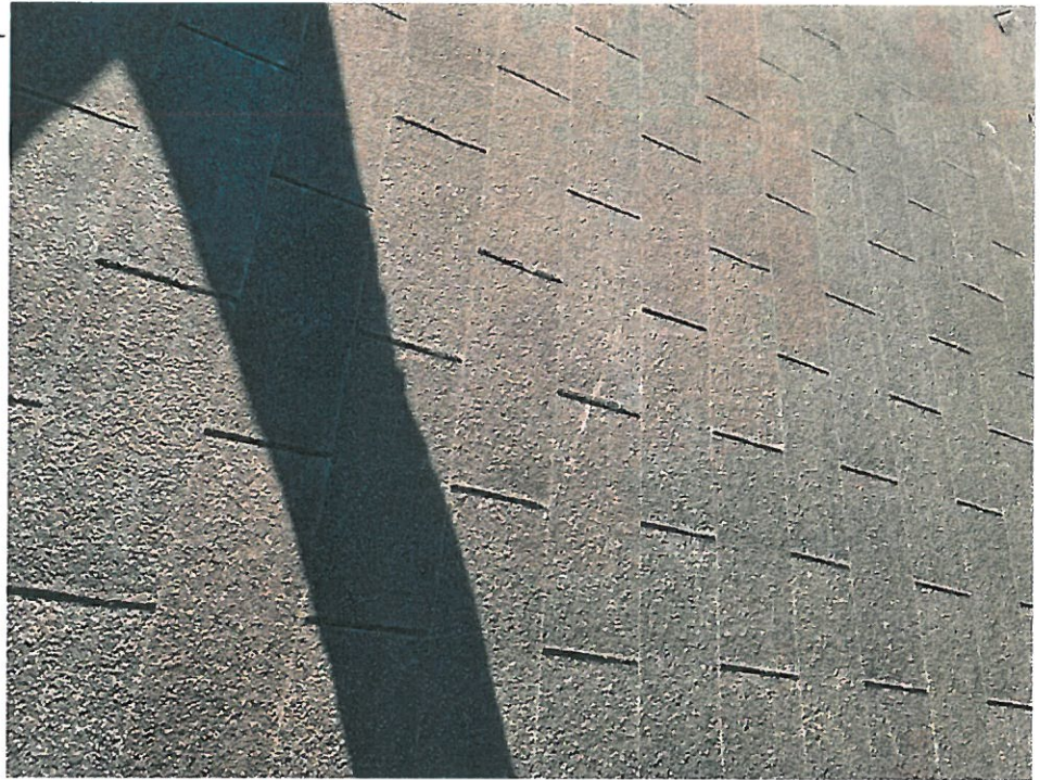
27 Roof/Roof - 79-79-Jan 31 2022 03_52pm-HubE Date Taken: 1/31/2022
