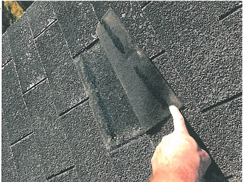
17 Roof/Roof - 69-69-Jan 31 2022 03_51pm-KvLw Date Taken: 1/31/2022
