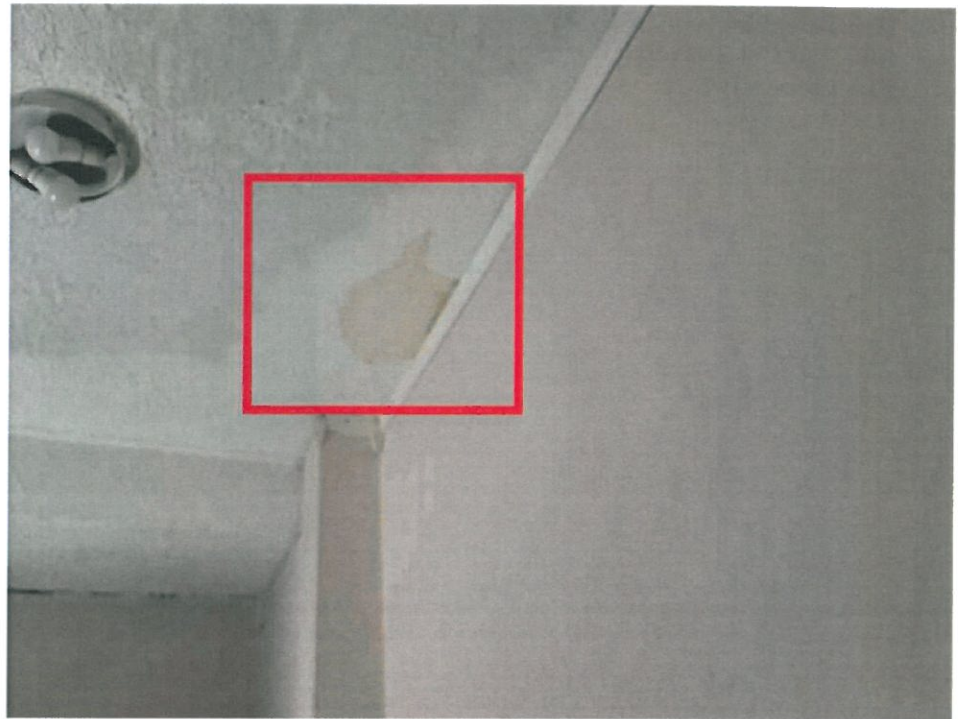
188 Main Level/Bathroom - 166-166- Jan 31 2022 04_21pm-16Vj Date Taken: 1/31/2022
