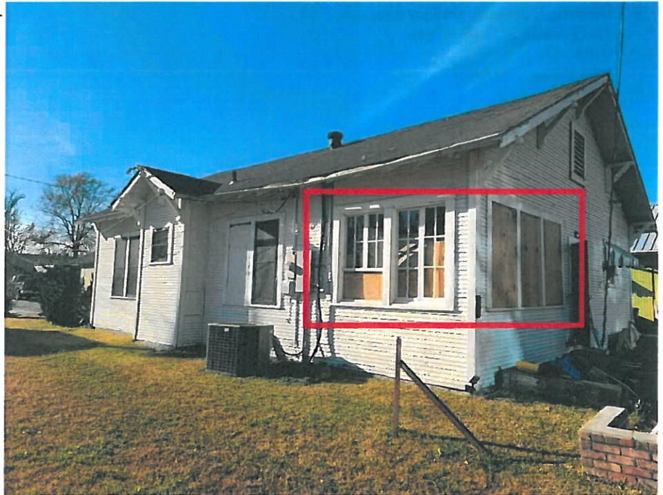
77 Dwelling Exterior/Right Elevation - 45-45-Jan 31 2022 03_46pm- YoRi Date Taken: 1/31/2022
