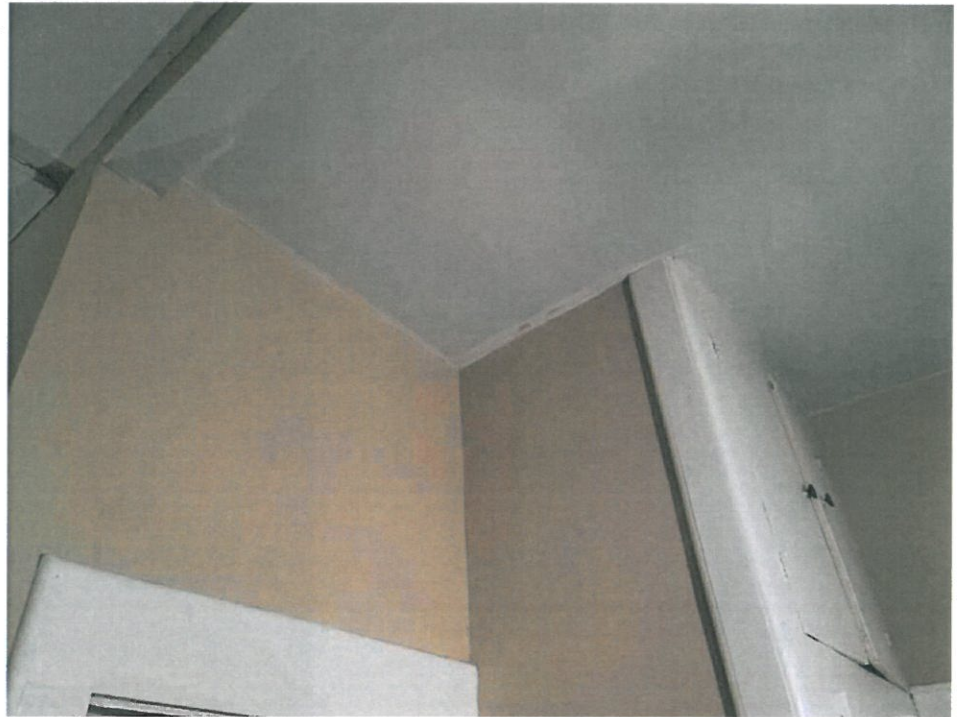
144 Main Level/Hallway - 209-209-Jan 31 2022 04_24pm-9J2t Date Taken: 1/31/2022
