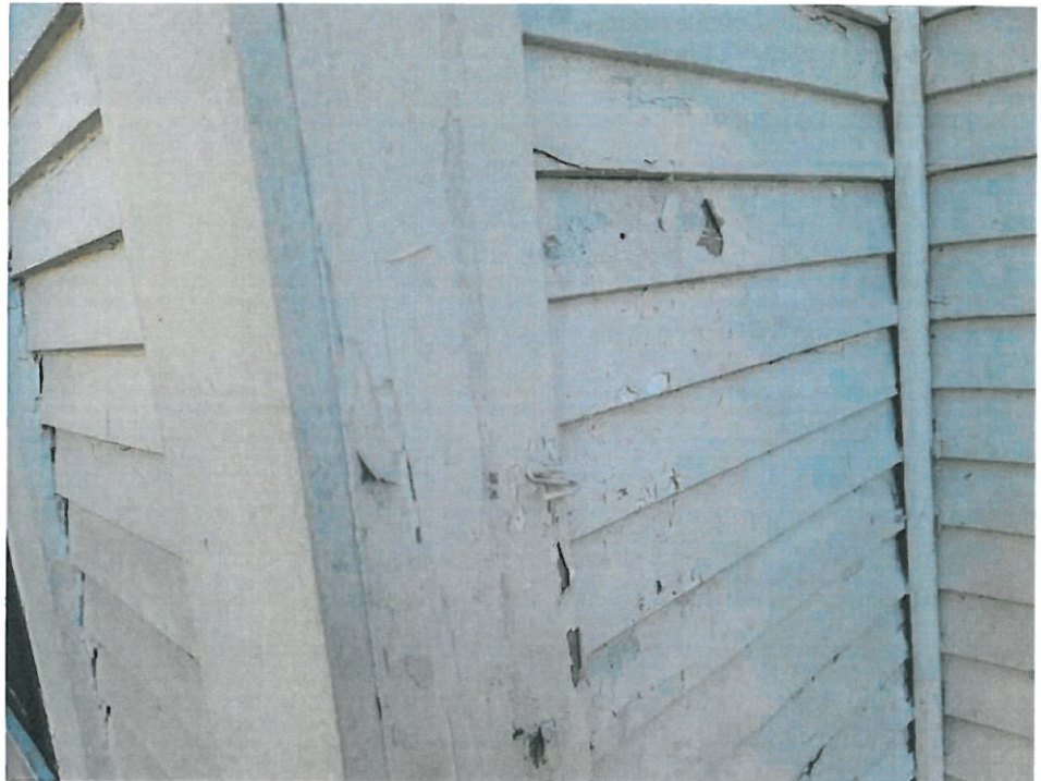
59 Dwelling Exterior/Left Elevation - 27-27-Jan 31 2022 03_43pm-9uFn Date Taken: 1/31/2022
