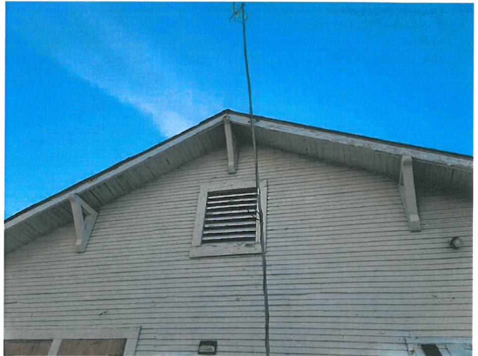
72 Dwelling Exterior/Rear Elevation - 40-40-Jan 31 2022 03_46pm- gUMA Date Taken: 1/31/2022
