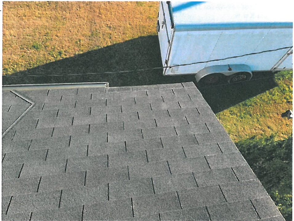
19 Roof/Roof - 71-71-Jan 31 2022 03_51pm-vH5R Date Taken: 1/31/2022
