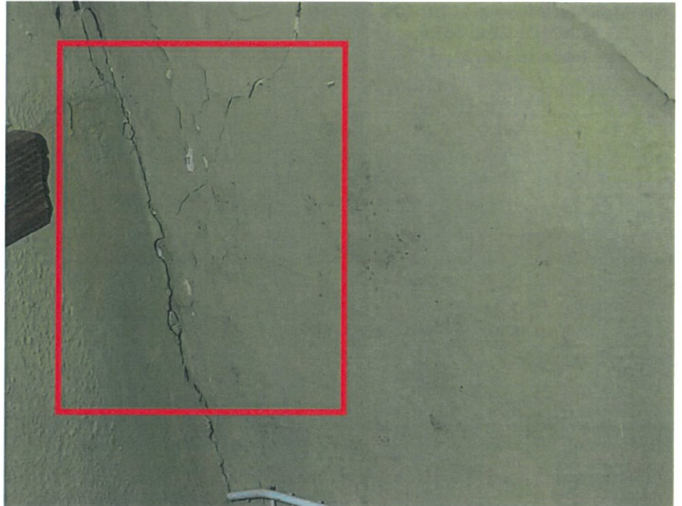
206 Main Level/Bedroom 2 - 203-203- Jan 31 2022 04_24pm-6u6v Date Taken: 1/31/2022
