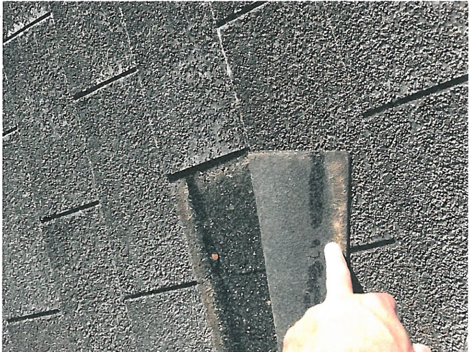
18 Roof/Roof - 70-70-Jan 31 2022 03_51pm-4Nrm Date Taken: 1/31/2022
