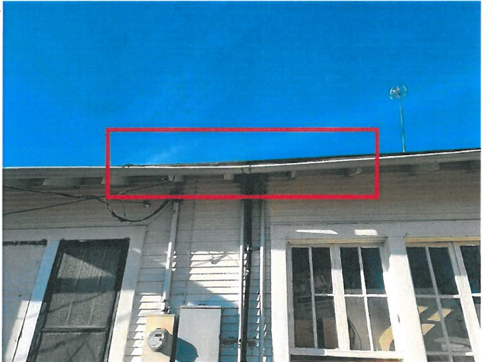
78 Dwelling Exterior/Right Elevation - 46-46-Jan 31 2022 03_46pm-tdiT Date Taken: 1/31/2022
