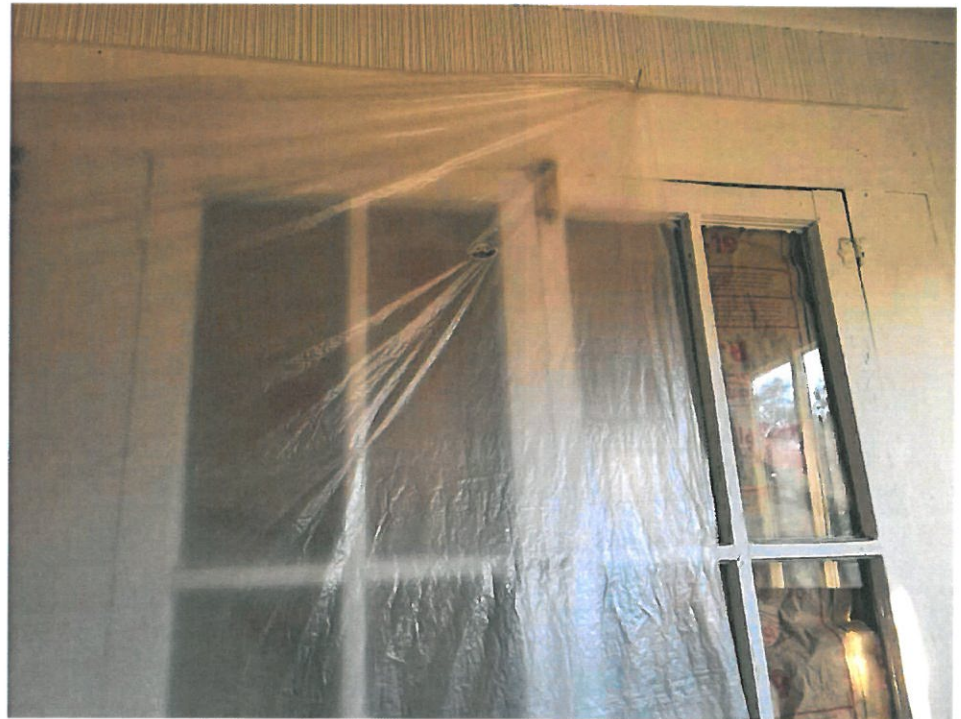
240 Main Level/Sun room - 223-223- Jan 31 2022 04_25pm-WbRt Date Taken: 1/31/2022
