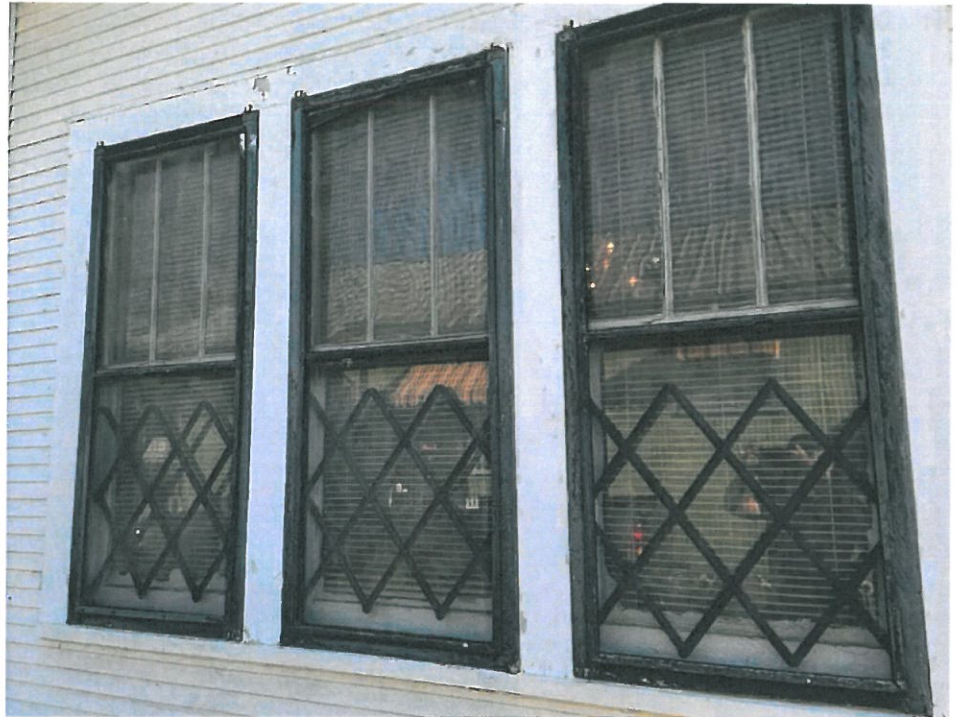
63 Dwelling Exterior/Left Elevation - 31-31-Jan 31 2022 03_44pm- 2Wso Date Taken: 1/31/2022
