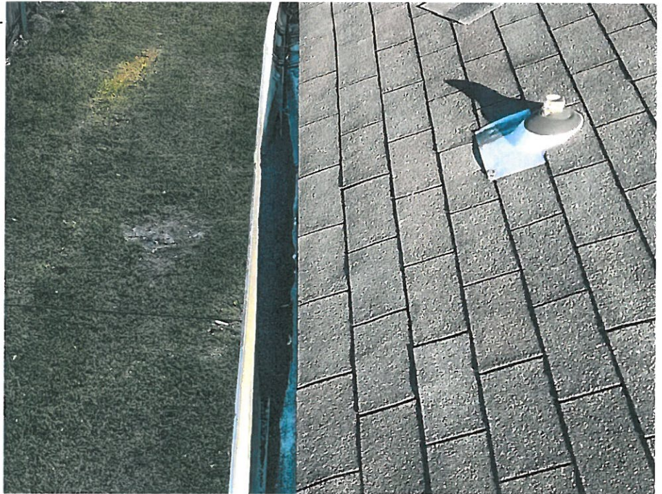
40 Roof/Roof - 92-92-Jan 31 2022 03_ 53pm-ZNSm Date Taken: 1/31/2022
