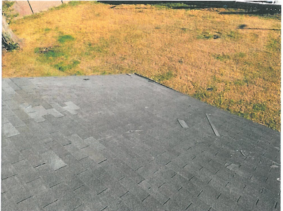
29 Roof/Roof - 81-81-Jan 31 2022 03_52pm-5ZhW Date Taken: 1/31/2022
