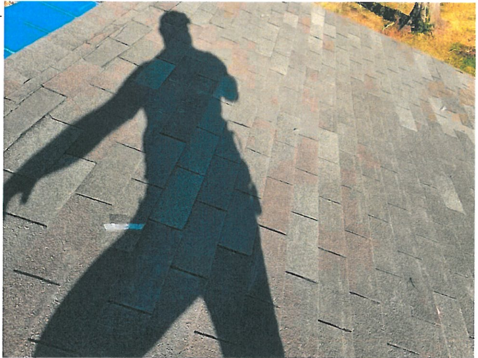
28 Roof/Roof - 80-80-Jan 31 2022 03_52pm-5bcL Date Taken: 1/31/2022
