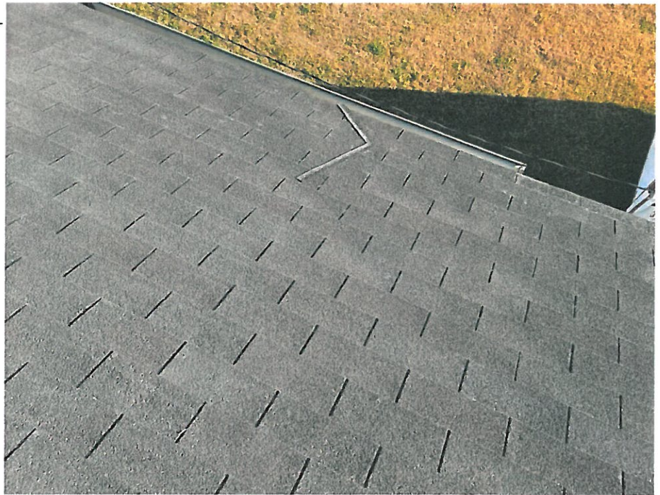
20 Roof/Roof - 72-72-Jan 31 2022 03_51pm-GgCJ Date Taken: 1/31/2022
