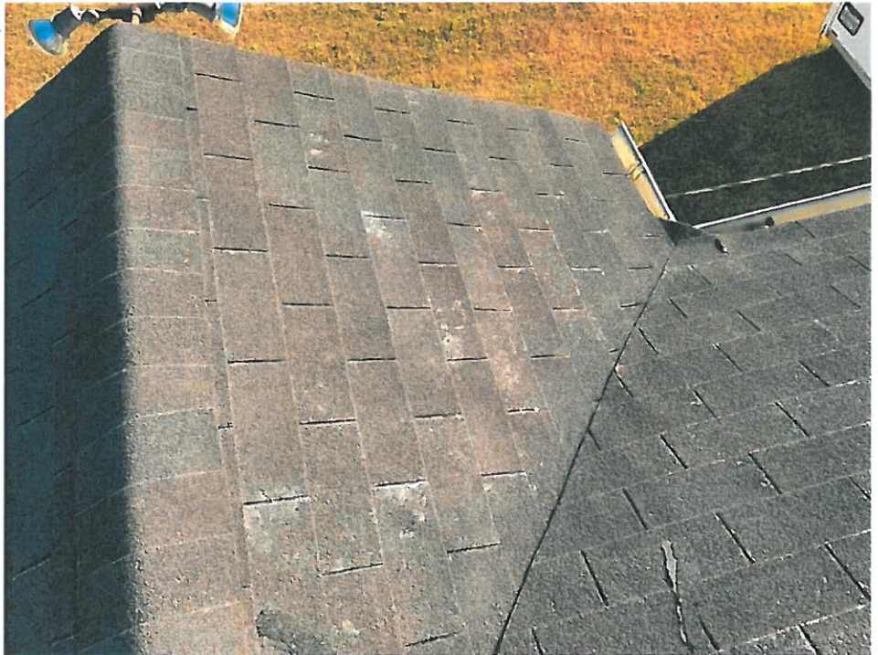
22 Roof/Roof - 74-74-Jan 31 2022 03_51pm-M3rr Date Taken: 1/31/2022
