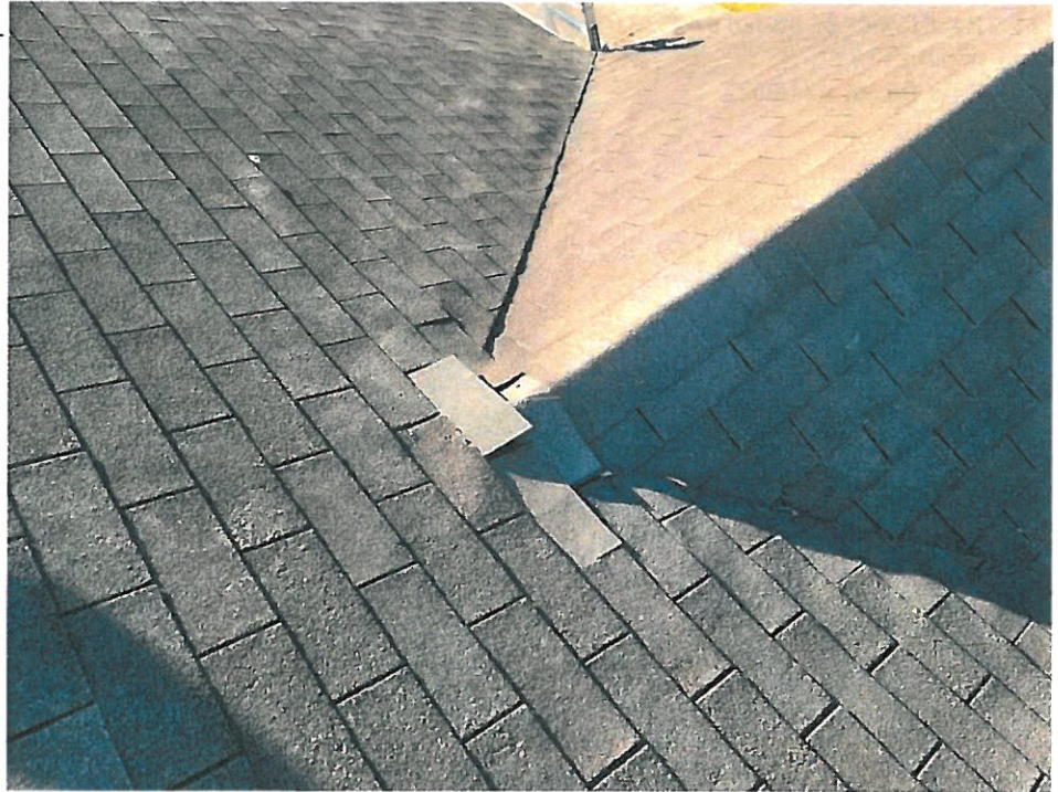
36 Roof/Roof - 88-88-Jan 31 2022 03_52pm-aQGx Date Taken: 1/31/2022
