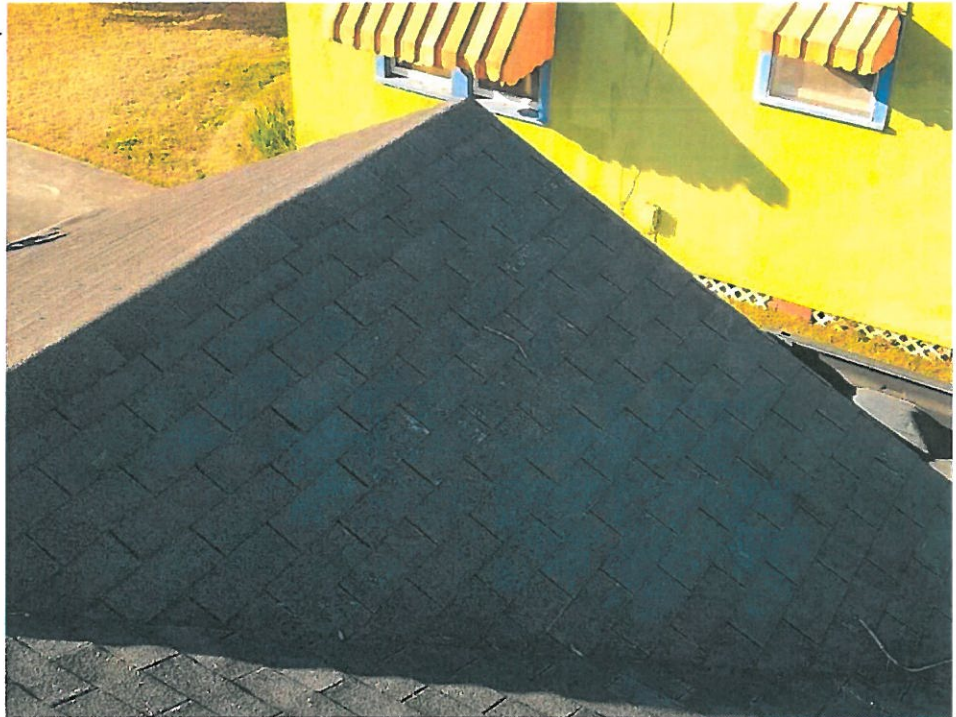
33 Roof/Roof - 85-85-Jan 31 2022 03_52pm-sjEo Date Taken: 1/31/2022
