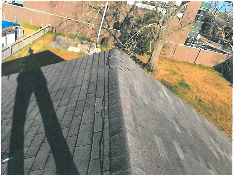
31 Roof/Roof - 83-83-Jan 31 2022 03_52pm-fmjw Date Taken: 1/31/2022
