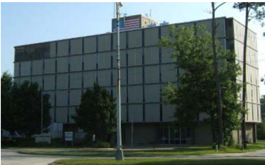
St Tammany Parish Admin Complex Katrina Storm Damage
