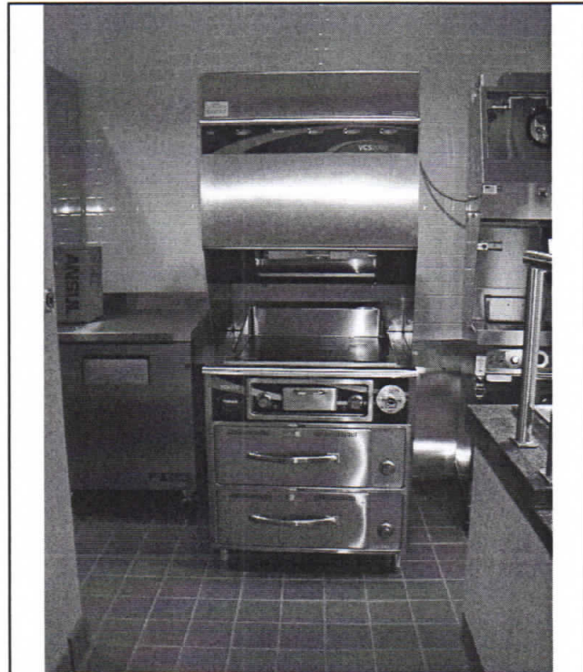
Figure 507.1(3) ELECTRIC GRIDDLE WITH RECIRCULATING HOOD
