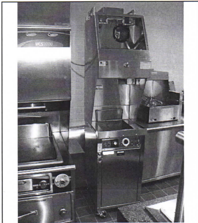
Figure 507.1(2) ELECTRIC DEEP FAT FRYER WITH RECIRCULATING HOOD
