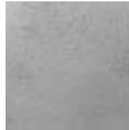
Sand-aggregated float finish
