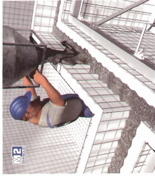
Concrete cast inside double panels braced with light prop.
