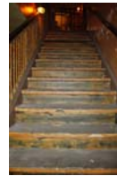
94-BALCONY ACCESS STAIRS (3)
