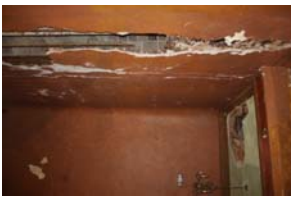
96-BALCONY ACCESS STAIRS (6)
