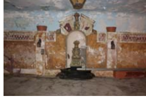
123-BASEMENT LOBBY AND LOUNGES (3)
