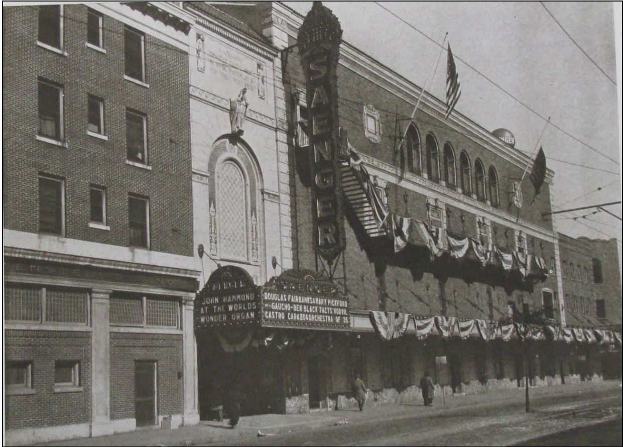
Figure 5: Photograph of Saenger Theatre, Rampart Street entrance (ca. 1927) Illustrations of Selected Work of Emile Weil, Architect, New Orleans 1900-1928 Collection 82, Emile Weil Office Records, Folder 14 Southeastern Architecture Archives, Tulane University
