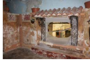
124-BASEMENT LOBBY AND LOUNGES (5)
