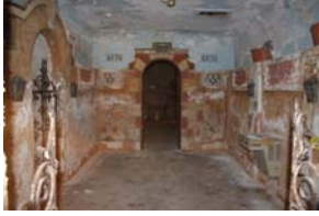
126-BASEMENT LOBBY AND LOUNGES (6)
