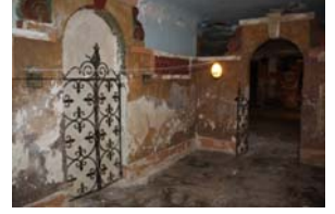
125-BASEMENT LOBBY AND LOUNGES (1)
