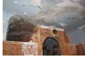
129-BASEMENT LOBBY AND LOUNGES (7)
