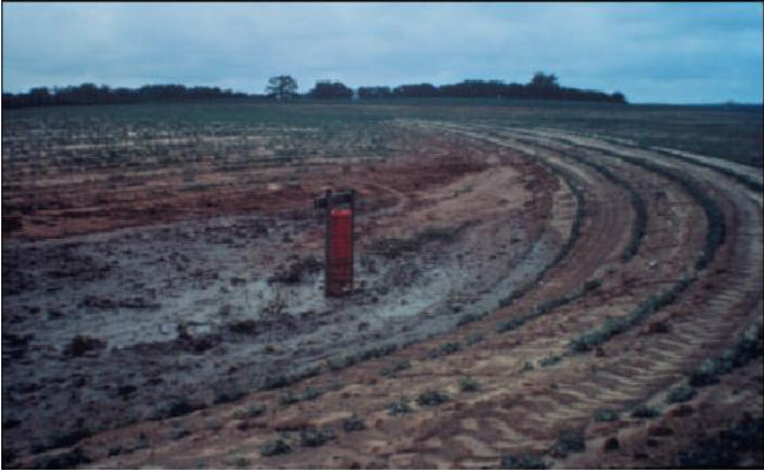
Figure 10. Water and sediment control basin (USDA Natural Resources Conservation Service).
