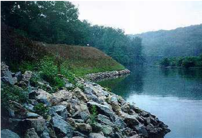
Figure 8. Riprap bank armoring for channel stabilization, Little Miami River, Ohio.
