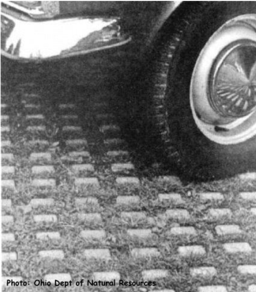
Figure 2. Example of a concrete grid pavement used in an overflow parking area (ODNR 1992).
