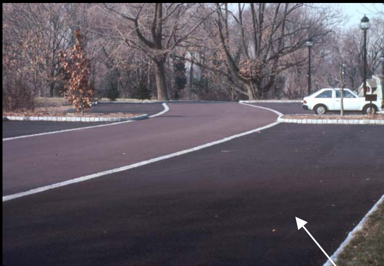
Porous asphalt pavement
