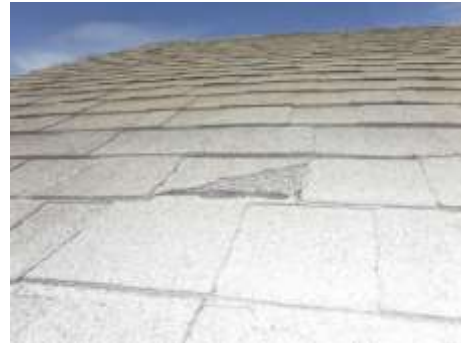
Figure 14 Broken shingles.
