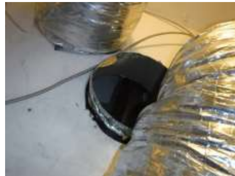
Figure 52 Connect the return air duct.
