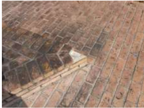
Figure 19 Missing bricks.
