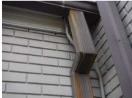
Figure 7 Gutters leak.
