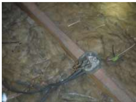
Figure 41 Remove all useless wiring.
