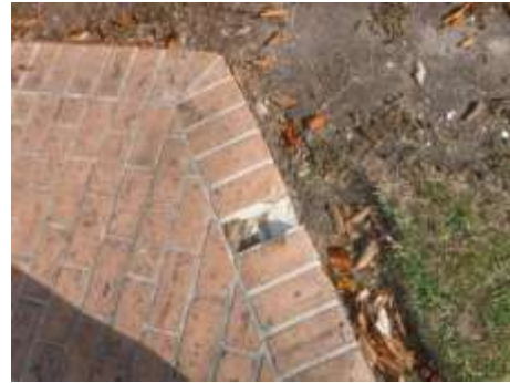
Figure 20 Missing bricks.
