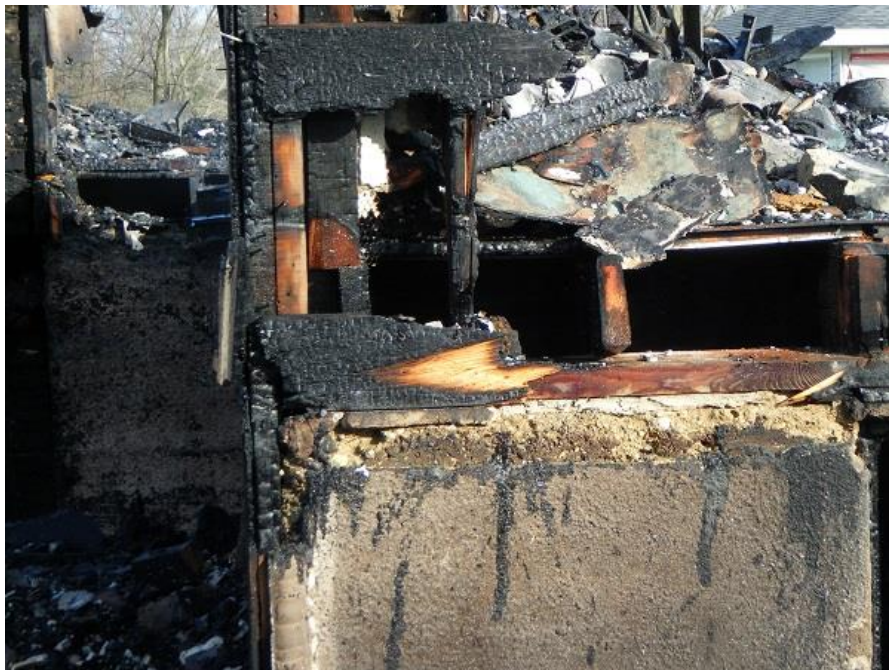
Photo 3 shows part of a load-bearing wood joist (unplanned dimensional lumber) from a residential structure fire. Although the surface was deeply charred, the joist failed anyway, probably because the char removed so much of the strength from the wood that it was no longer able to carry its load.
