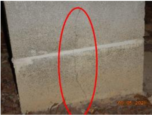
Photo 1: Rebuild Piers.
