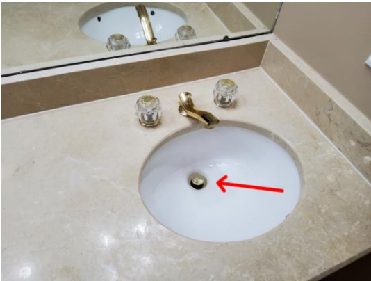
Photo 46: Drain Stopper Adjust.
