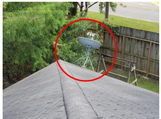
Photo 7: Dish Installed on Roof.
