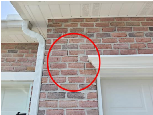
Photo 13: Cracks Typical.
