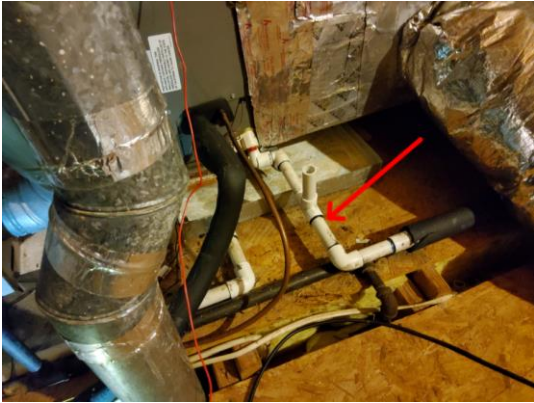
Photo 31: Insulate Condensate Drain Line.
