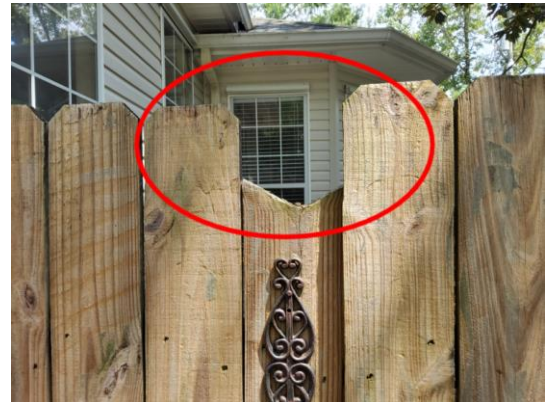
Photo 18: Fair Condition, Minor Repairs.
