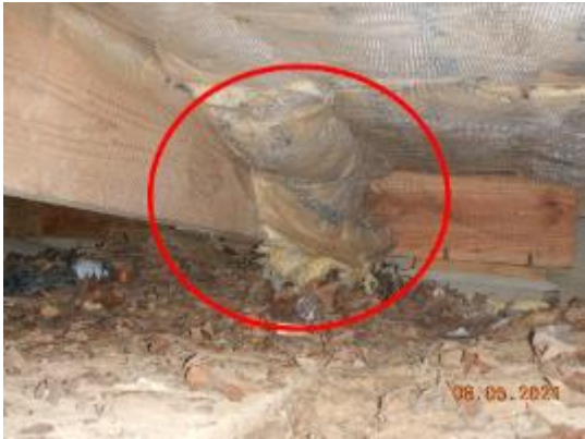
Photo 37: Loose/Damaged Insulation.
