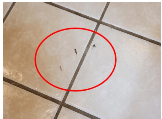
Photo 58: Tile Cracked.
