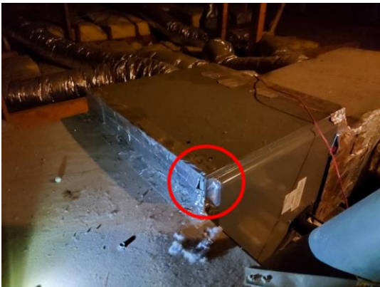
Photo 33: Seal Duct Openings.
