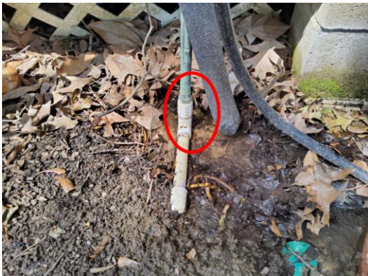
Photo 41: Pipe Leak.
