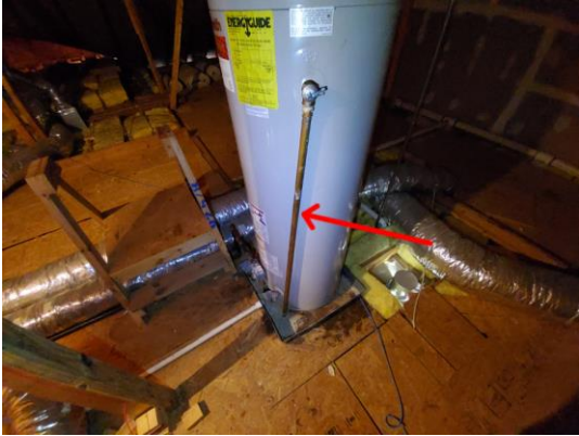
Photo 44: Add Discharge Piping for TPR.
