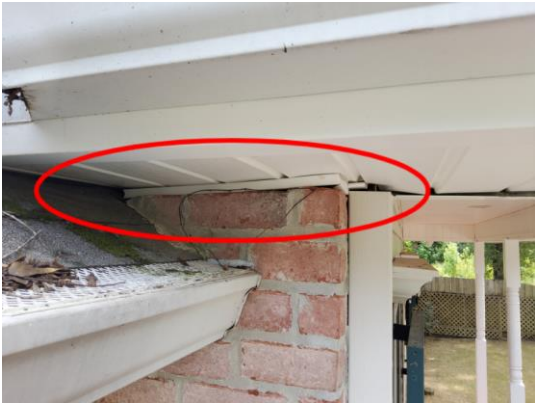
Photo 11: Seal Openings.
