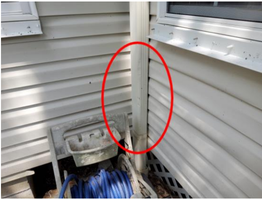
Photo 4: Downspout Damaged.
