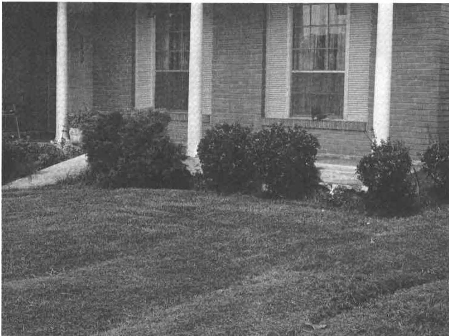
Figure 3.—Buried logs and stumps resulted in uneven subsidence. The soil is Westwego clay. It is poorly suited to use as homesites.
