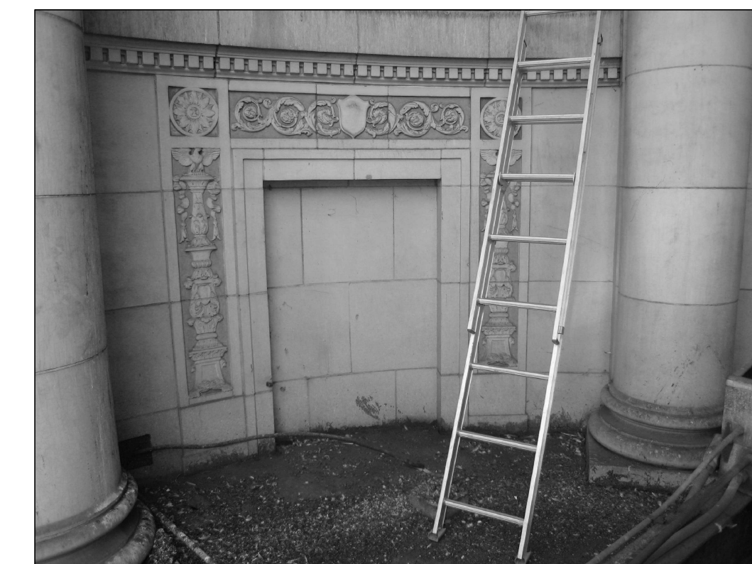
H PHOTO 2080 BLIND NICHE IN ALCOVE; CLEAN ALL ROOFING MATERIAL OFF TERRA COTTA
