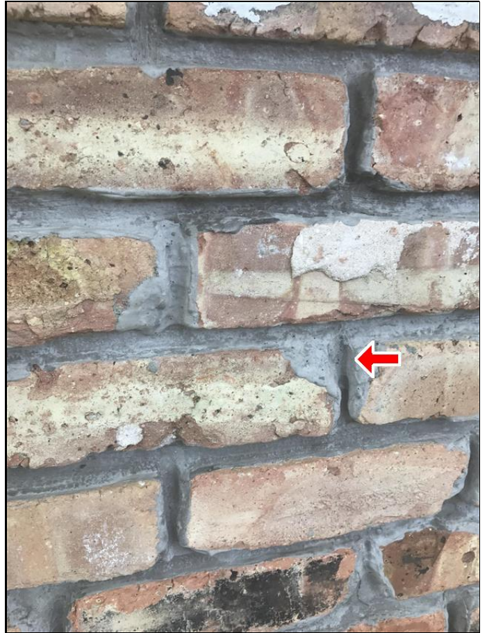
2.0 Item 4(Picture) weather coating over mortar
