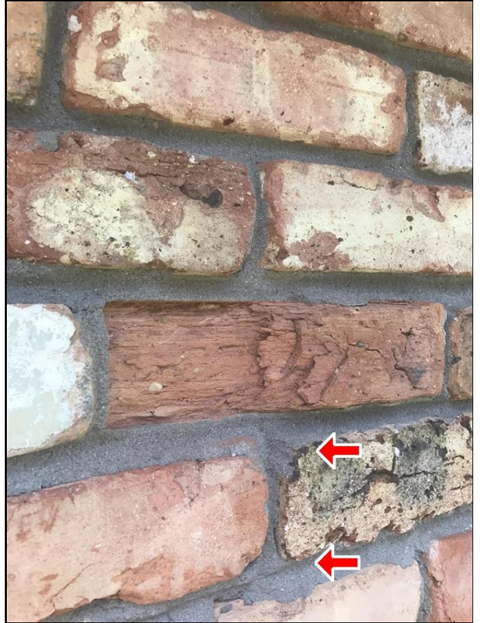
2.0 Item 2(Picture) mortar has weather proofing on mortar
