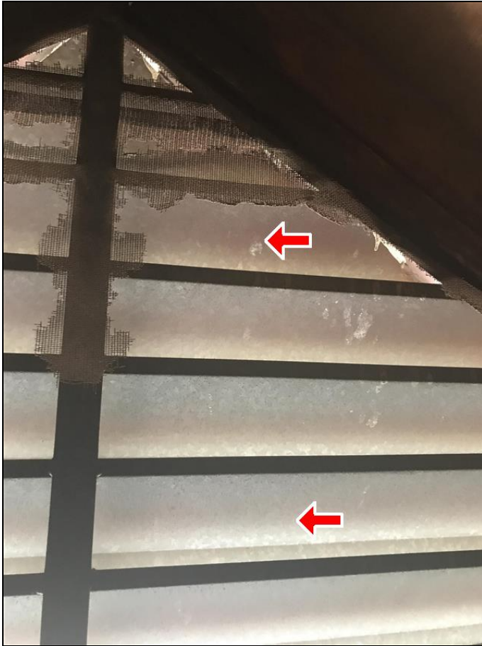
9.3 Item 1(Picture) re-screen gable vents
