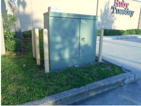
19. Pad-mounted transformer
