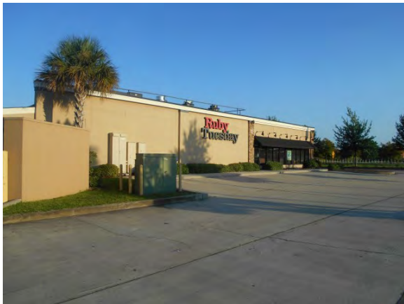
9. East side of the building
