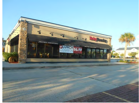
8. North side of the building
