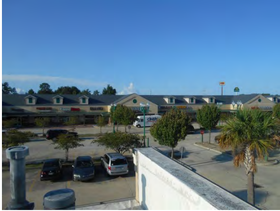
31. Adjacent to the south
