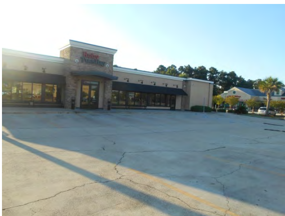
11. West side of the building
