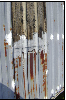
DAMAGED OVERLAPPING PANELS N.T.S.
