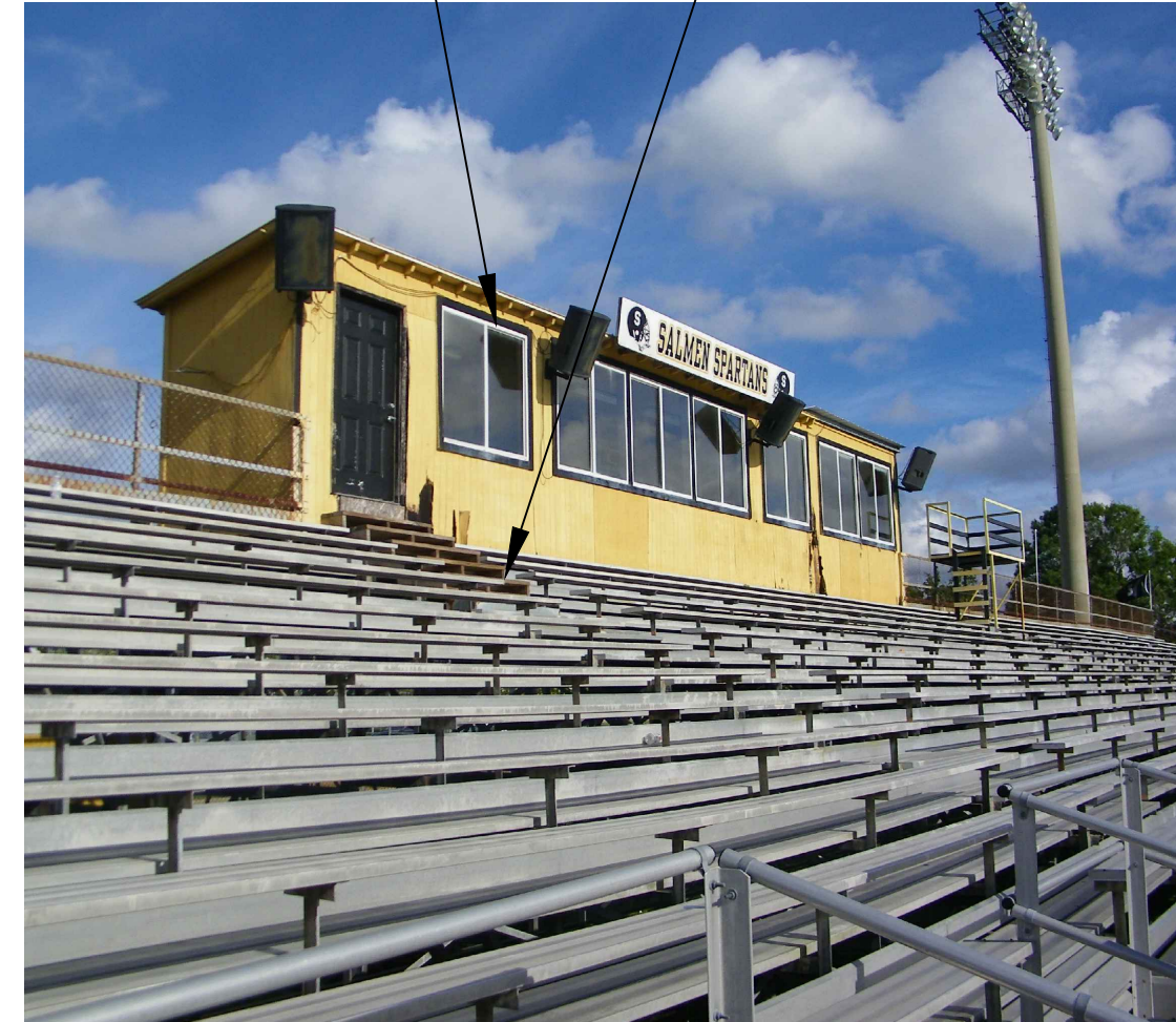
REMOVE ALL FIBER OPTIC AND PHONE COMMUNICATIONS AND SAVE FOR REINSTALLATION IN NEW PRESS BOX.
