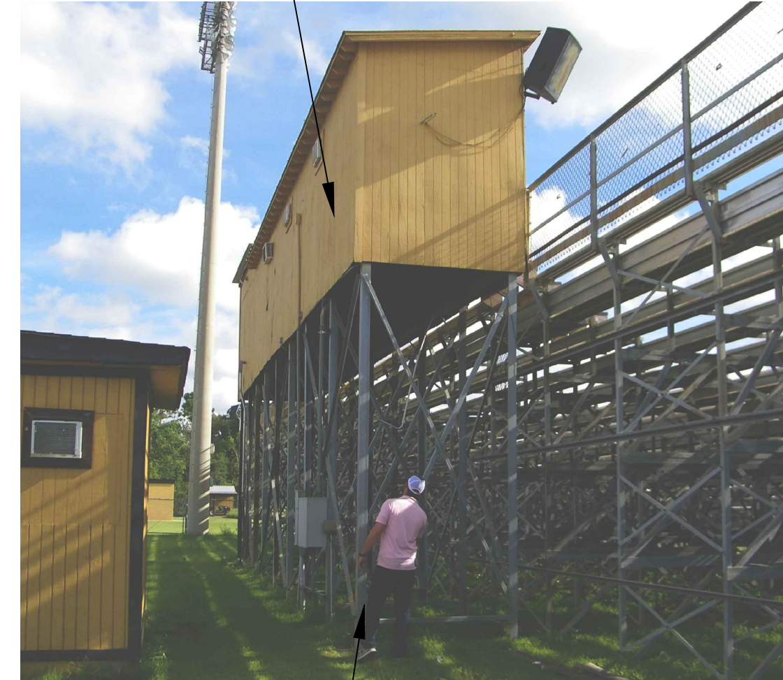
REMOVE ALL STEEL SUPPORTS AND CONCRETE FOOTINGS
