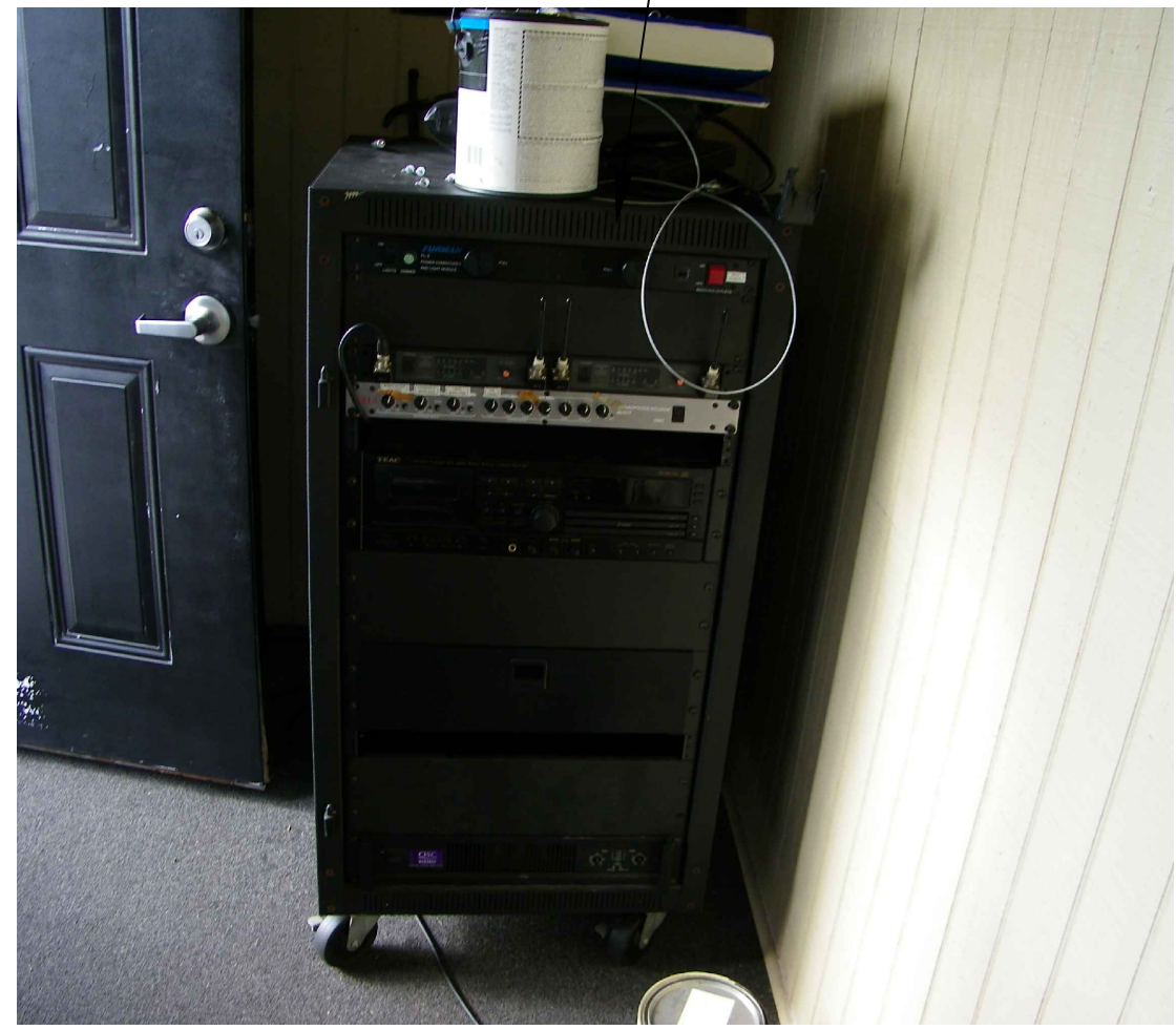
REMOVE PA SYSTEM AND SAVE FOR REINSTALL IN NEW PRESS BOX.
