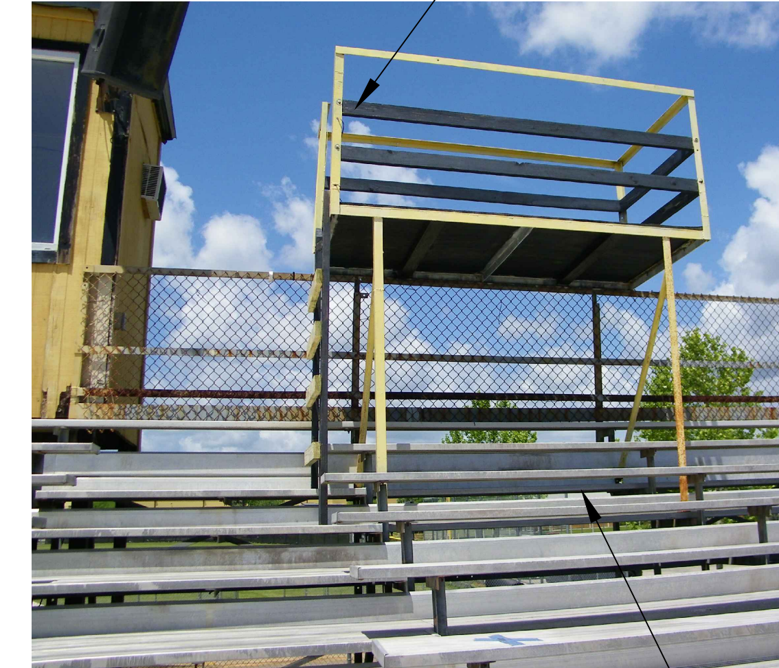
REPAIR BLEACHERS WHERE FRAMING WAS REMOVED.
