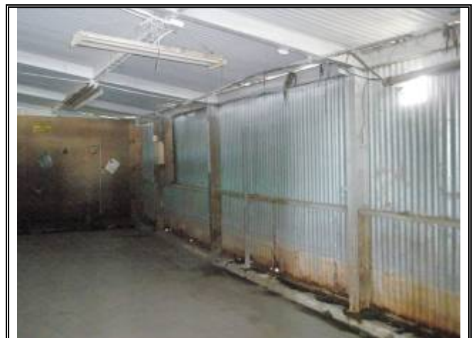
Photograph No. 030: inside storage shed of bldg 2
