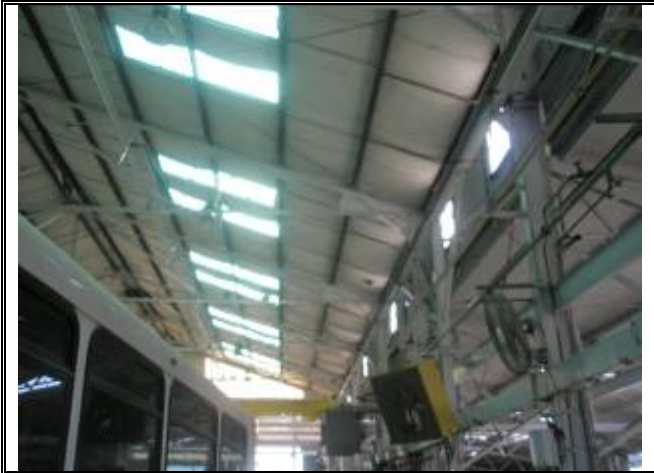
Photograph No. 019: inside of bldg 2
