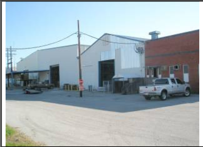
Photograph No. 001: overall facility
