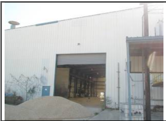
Photograph No. 032: west side of bldg 3
