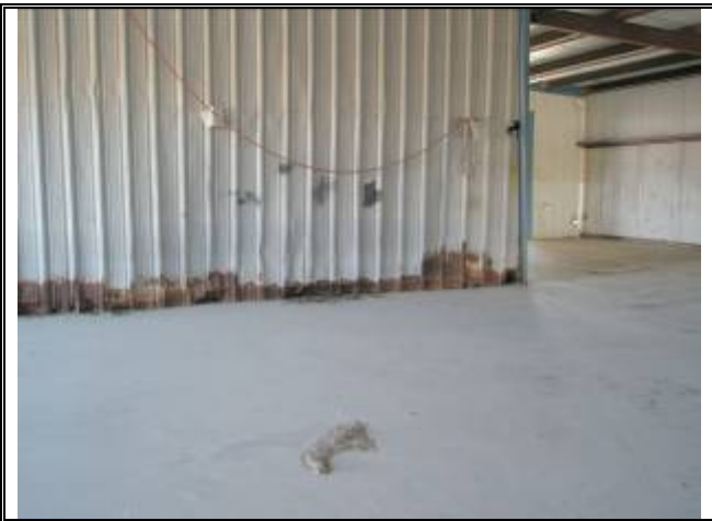
Photograph No. 068: inside of bldg 5
