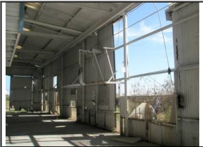
Photograph No. 026: inside of bldg 2
