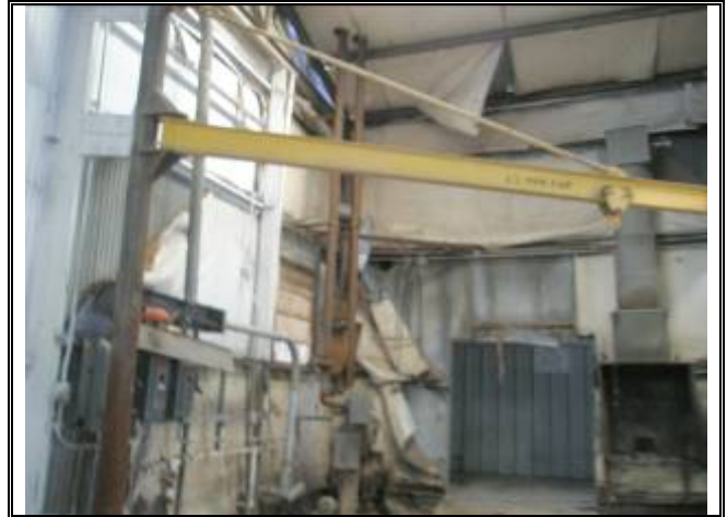
Photograph No. 052: inside of bldg 4
