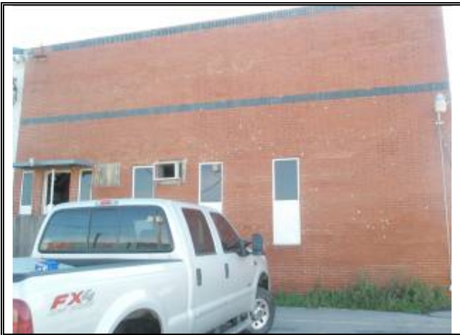
Photograph No. 002: west side of bldg 1
