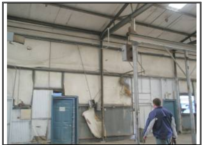
Photograph No. 054: inside of bldg 4
