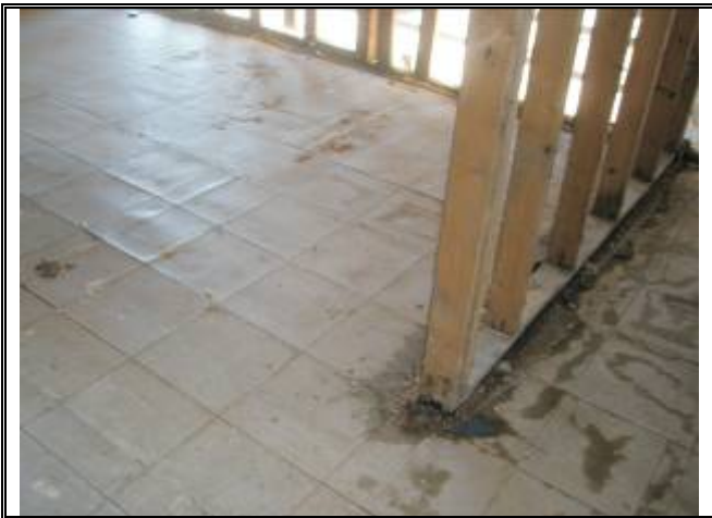
Photograph No. 008: inside downstairs of bldg 1
