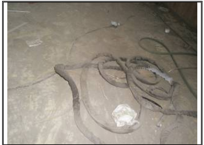
Photograph No. 023: inside upstairs offices of bldg 2
