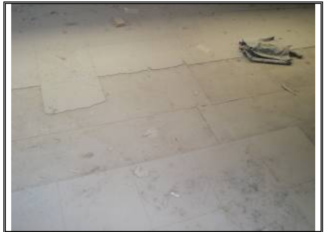
Photograph No. 047: inside upstairs office of bldg 3
