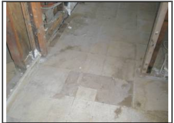
Photograph No. 005: inside downstairs of bldg 1
