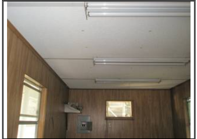
Photograph No. 022: inside upstairs offices of bldg 2
