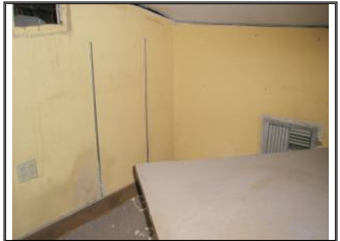
Photograph No. 011: inside upstairs of bldg 1
