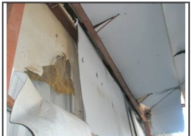
Photograph No. 066: inside of bldg 5
