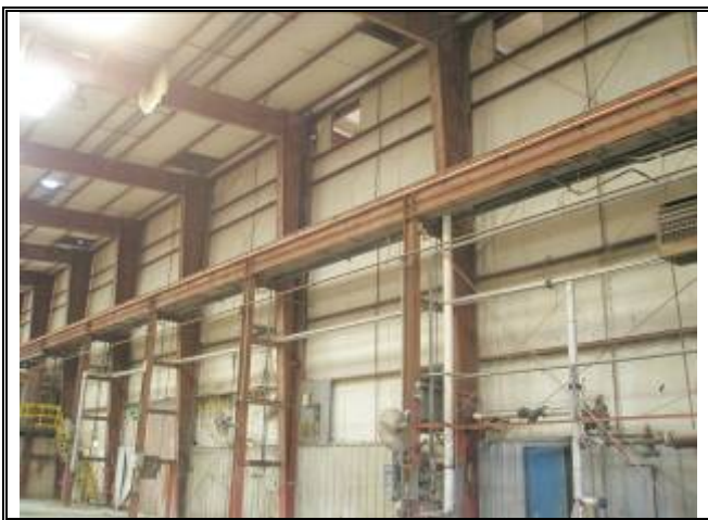
Photograph No. 039: inside of bldg 3
