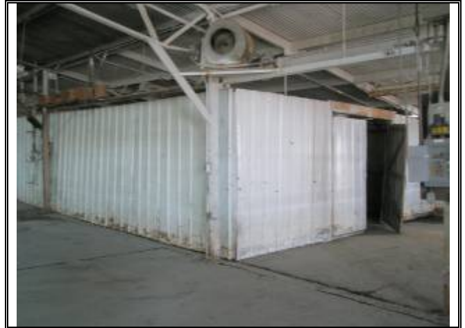
Photograph No. 028: inside of bldg 2
