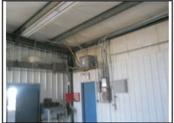
Photograph No. 064: inside of bldg 5
