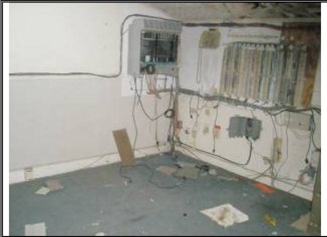
Photograph No. 013: inside upstairs of bldg 1
