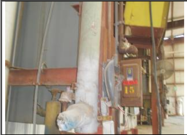
Photograph No. 043: inside of bldg 3
