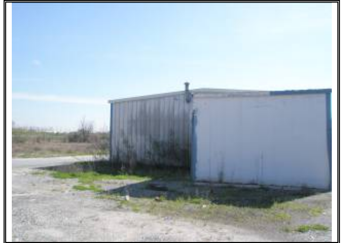
Photograph No. 058: west side of bldg 5
