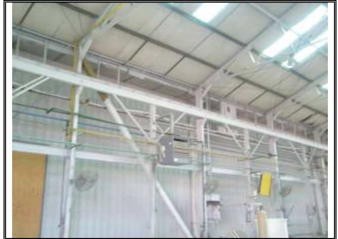
Photograph No. 016: inside of bldg 2
