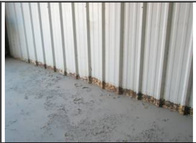
Photograph No. 062: inside of bldg 5
