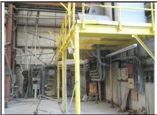
Photograph No. 038: inside of bldg 3
