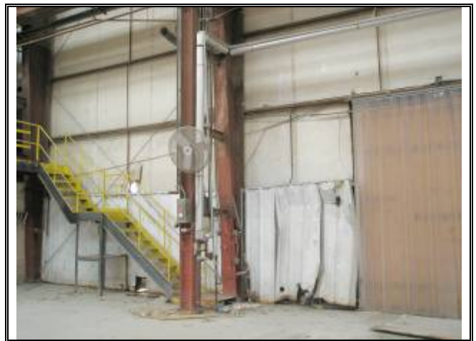
Photograph No. 041: inside of bldg 3
