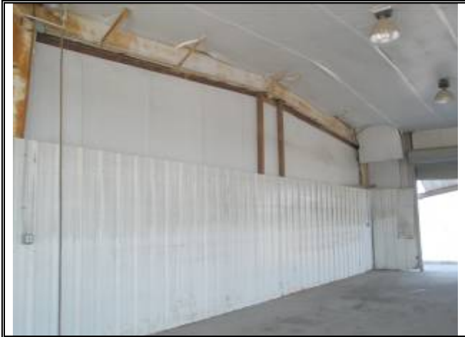
Photograph No. 073: inside of bldg 5
