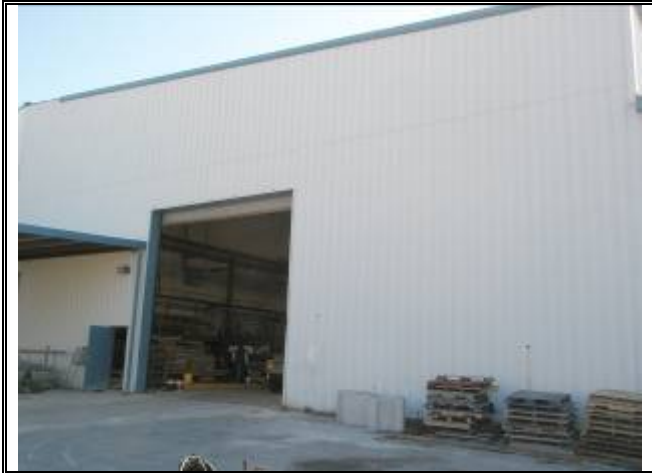
Photograph No. 031: west side of bldg 3
