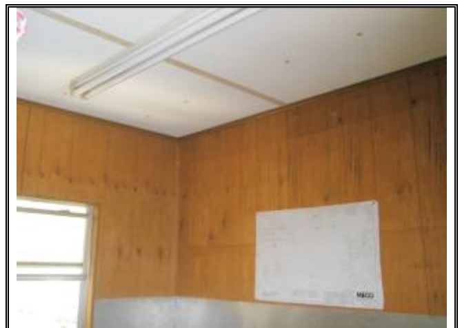
Photograph No. 024: inside upstairs offices of bldg 2
