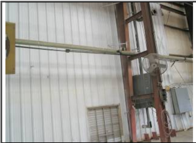
Photograph No. 044: inside of bldg 3
