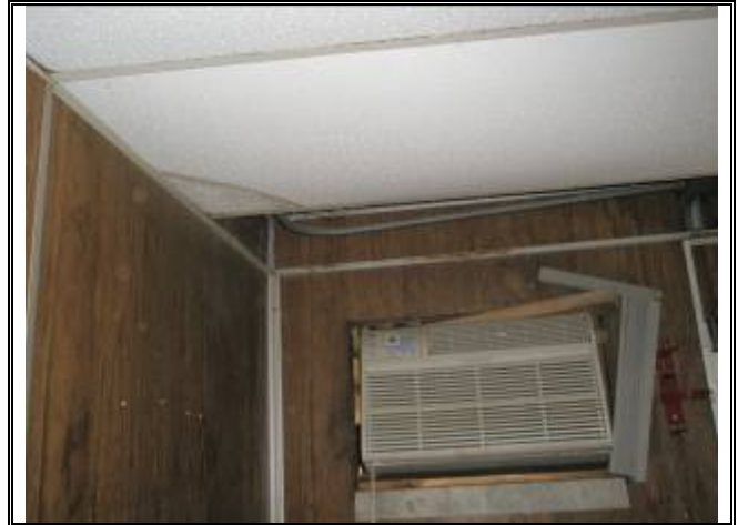
Photograph No. 046: inside upstairs office of bldg 3
