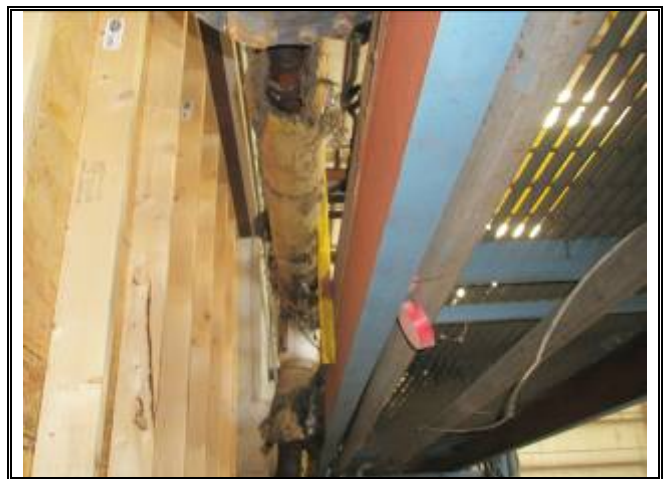
Photograph No. 036: inside of bldg 3
