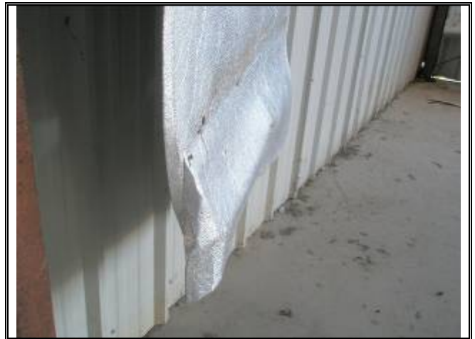
Photograph No. 065: inside of bldg 5
