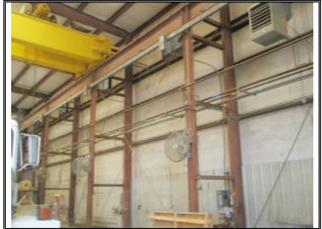
Photograph No. 034: inside of bldg 3
