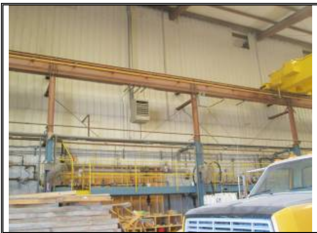
Photograph No. 033: inside of bldg 3
