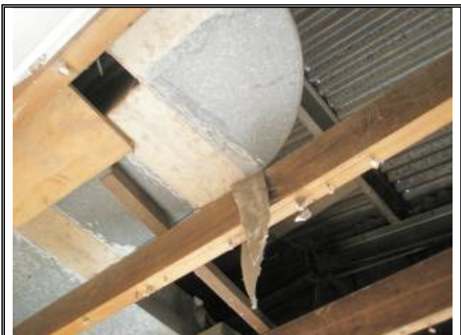
Photograph No. 009: inside downstairs of bldg 1
