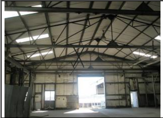
Photograph No. 055: inside of bldg 4
