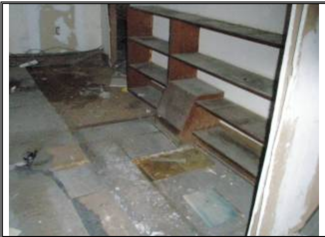
Photograph No. 014: inside upstairs of bldg 1
