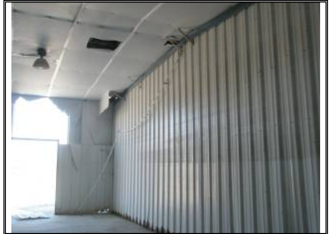
Photograph No. 070: inside of bldg 5
