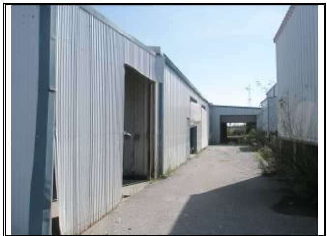
Photograph No. 060: south side of bldg 5
