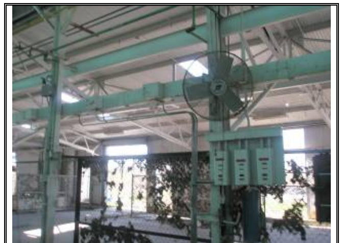
Photograph No. 018: inside of bldg 2
