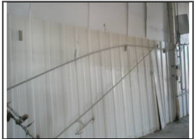
Photograph No. 071: inside of bldg 5
