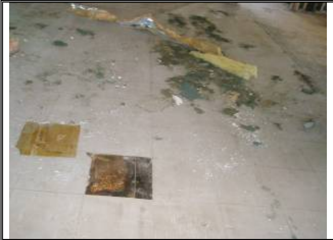
Photograph No. 007: inside downstairs of bldg 1
