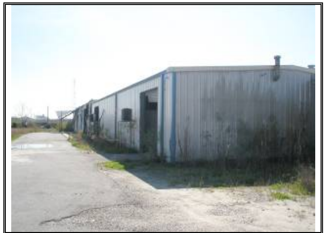
Photograph No. 059: north side of bldg 5
