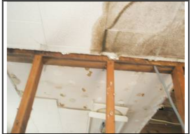
Photograph No. 010: inside downstairs of bldg 1
