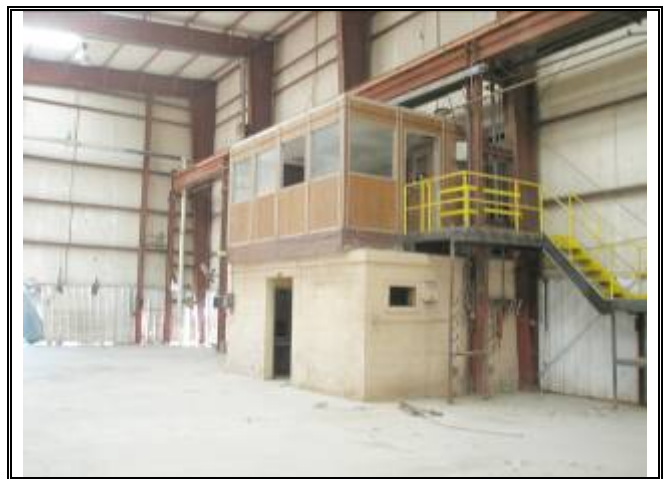
Photograph No. 042: inside of bldg 3
