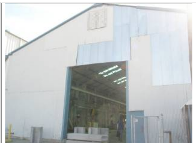
Photograph No. 015: west side of bldg 2
