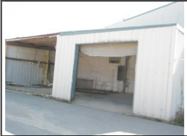
Photograph No. 049: west side of bldg 4
