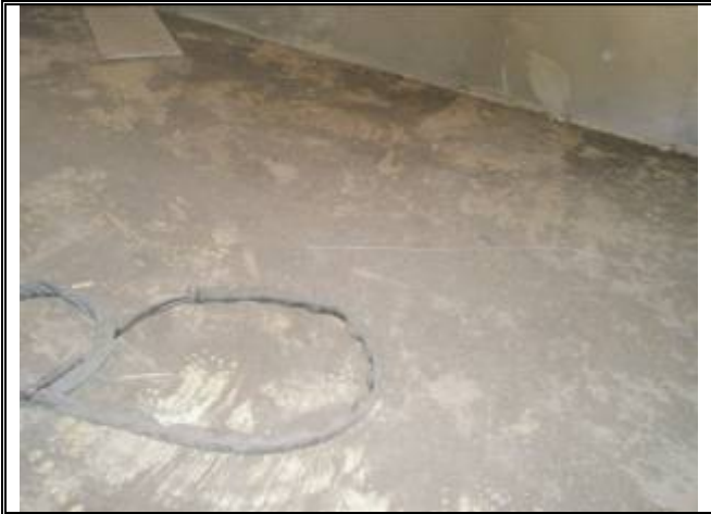
Photograph No. 025: inside upstairs offices of bldg 2
