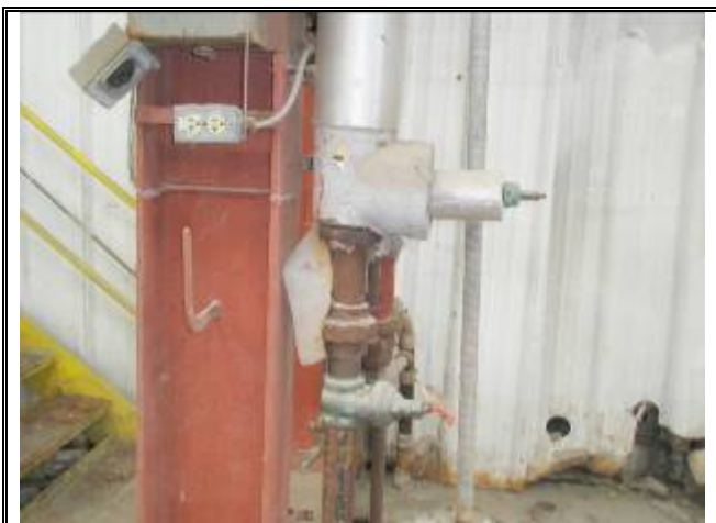
Photograph No. 045: inside of bldg 3
