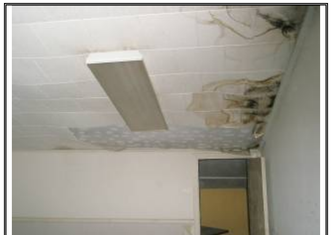
Photograph No. 012: inside upstairs of bldg 1
