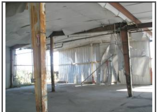
Photograph No. 072: inside of bldg 5
