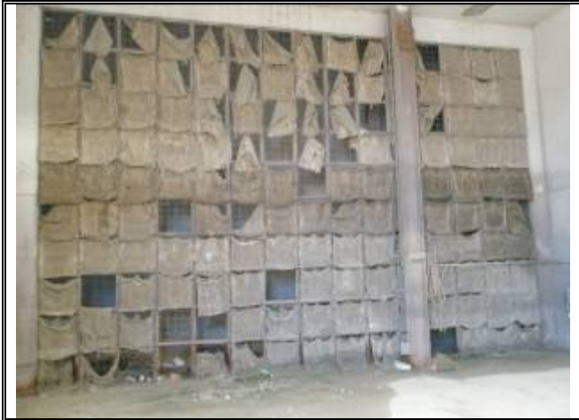
Photograph No. 037: inside of bldg 3
