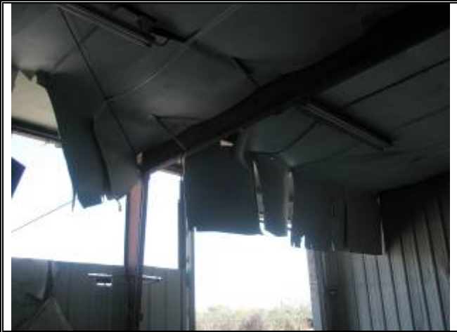
Photograph No. 067: inside of bldg 5
