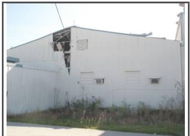
Photograph No. 048: west side of bldg 4
