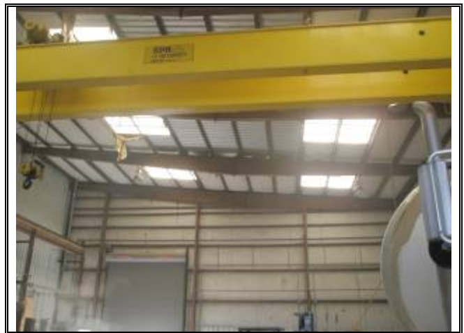
Photograph No. 035: inside of bldg 3
