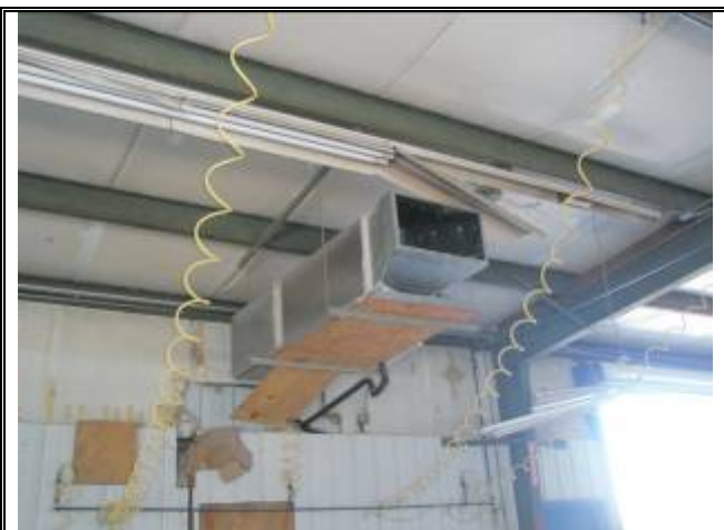
Photograph No. 063: inside of bldg 5
