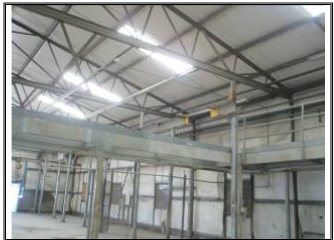
Photograph No. 053: inside of bldg 4
