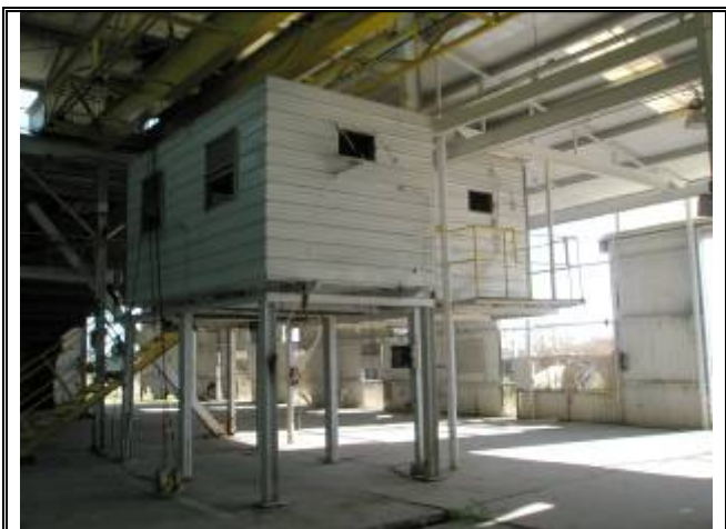
Photograph No. 021: inside of bldg 2
