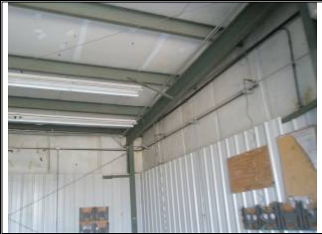
Photograph No. 061: inside of bldg 5
