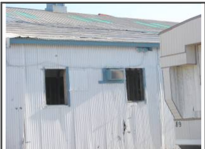
Photograph No. 003: south side of bldg 1
