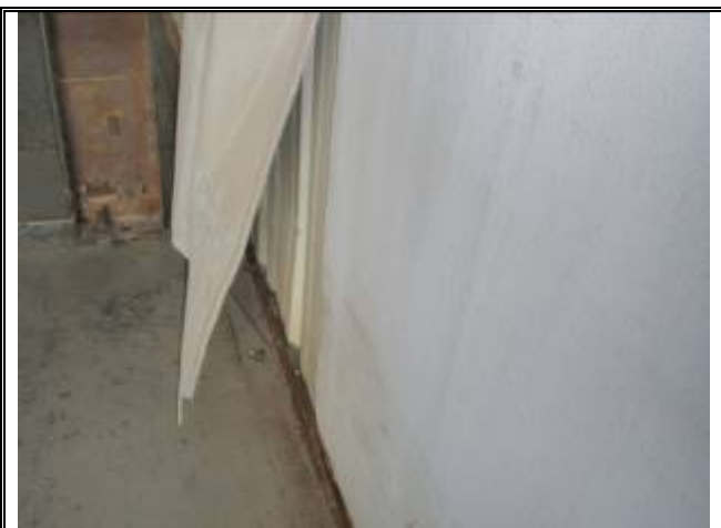
Photograph No. 069: inside of bldg 5
