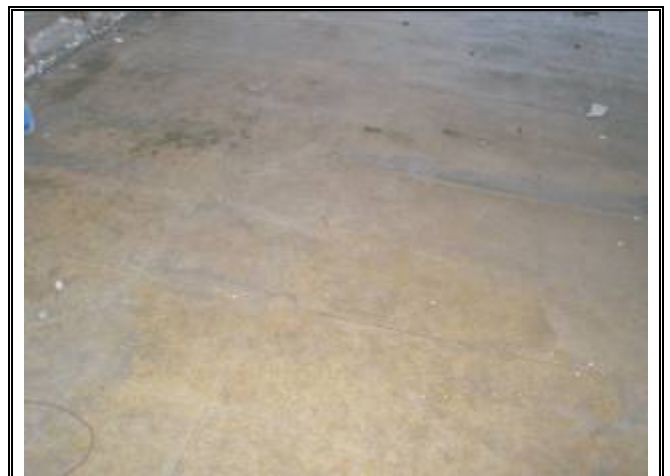
Photograph No. 006: inside downstairs of bldg 1
