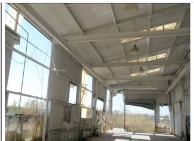
Photograph No. 027: inside of bldg 2
