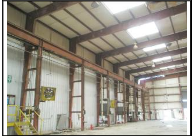
Photograph No. 040: inside of bldg 3
