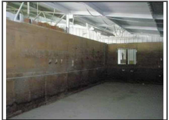
Photograph No. 029: inside storage shed of bldg 2
