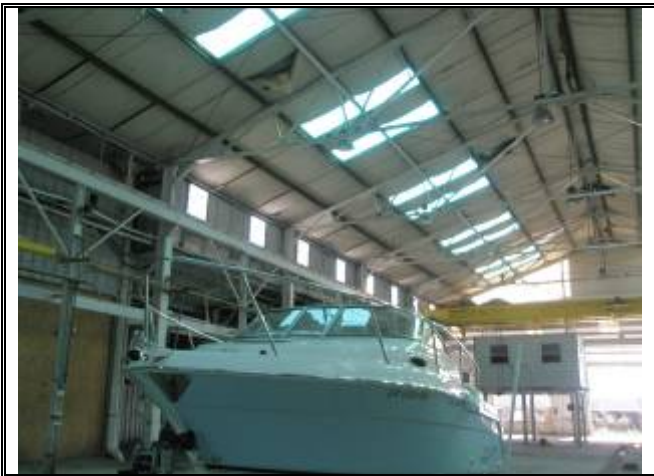
Photograph No. 020: inside of bldg 2
