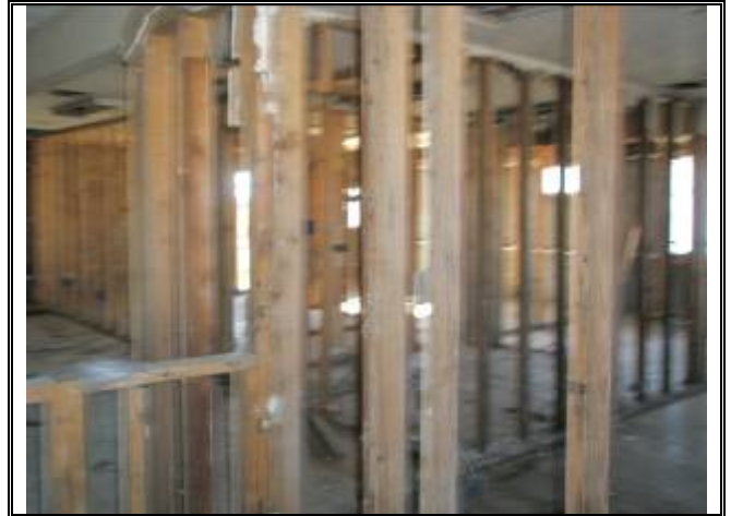
Photograph No. 004: inside downstairs of bldg 1
