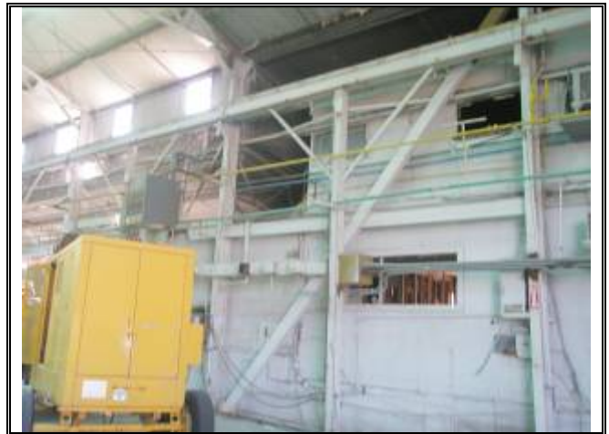
Photograph No. 017: inside of bldg 2
