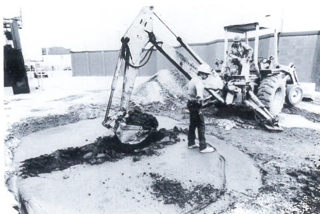
Fig. 4.1—Excavating CLSM with backhoe.
