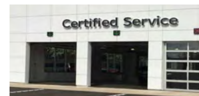
3 EXTERIOR LOT PAVEMENT MARKINGS AND EXTERIOR DIRECTIONAL LANE LIGHTS
