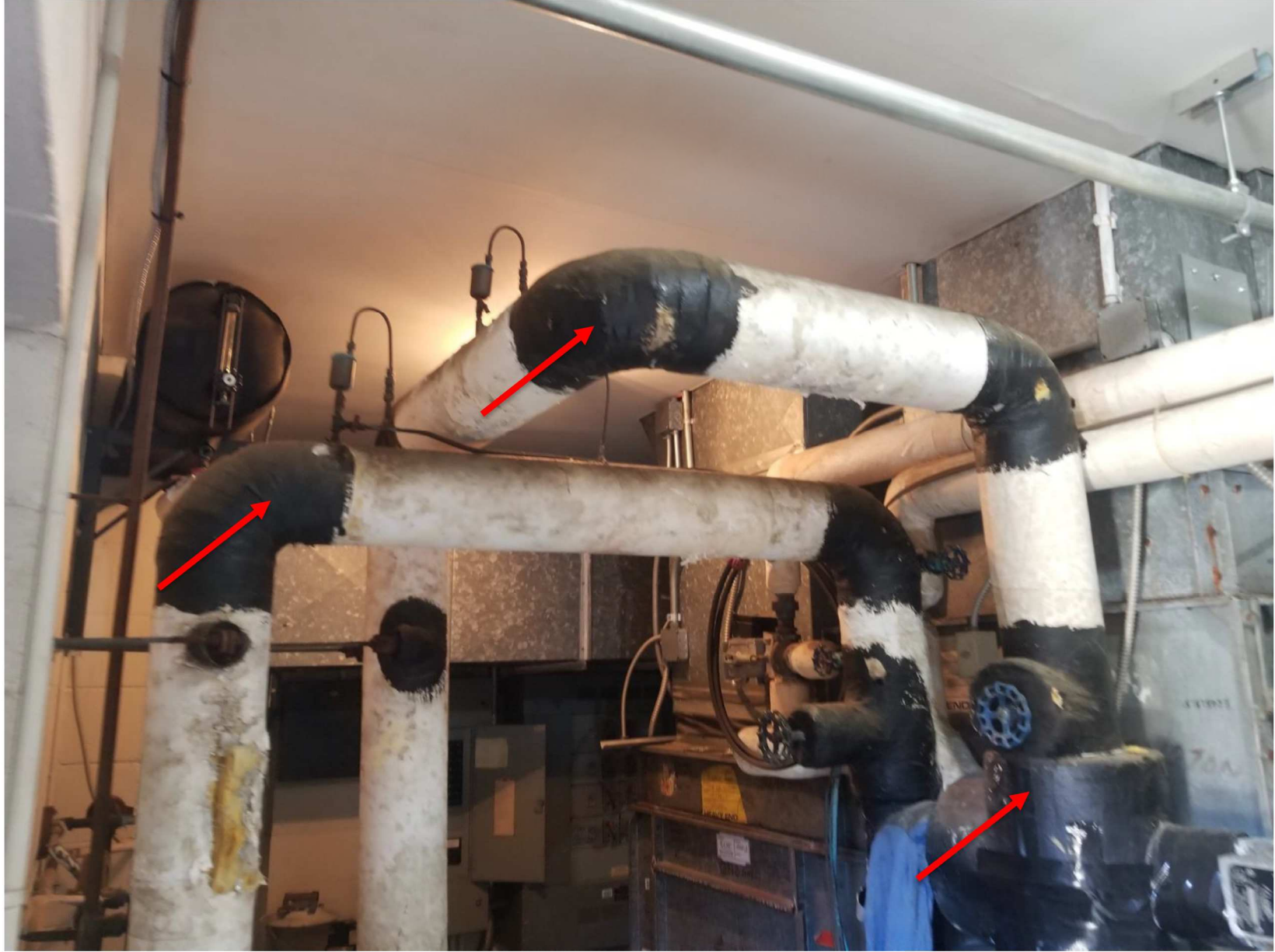
View of HA-05: Black, tar like pipe/pipe insulation covering.
