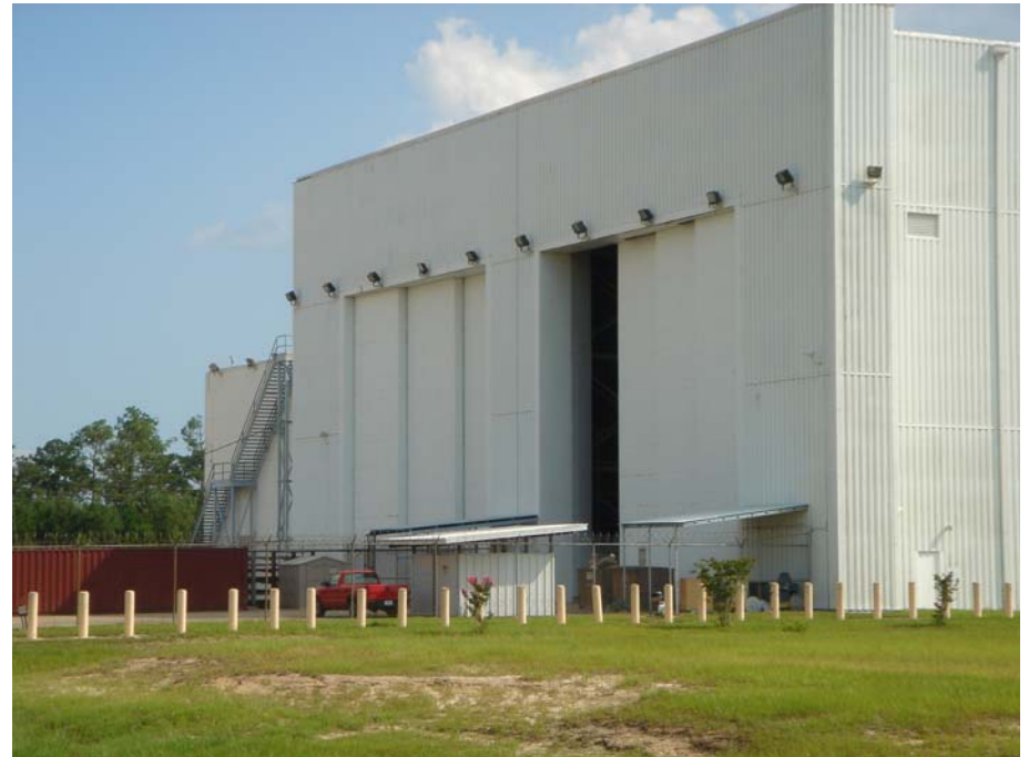
The north/east elevation of Building 3202 which shows the bay doors to the buoy maintenance area. This entrance will be adjacent to the blast and paint booth. See Part 6 - Attachments for booth data.
