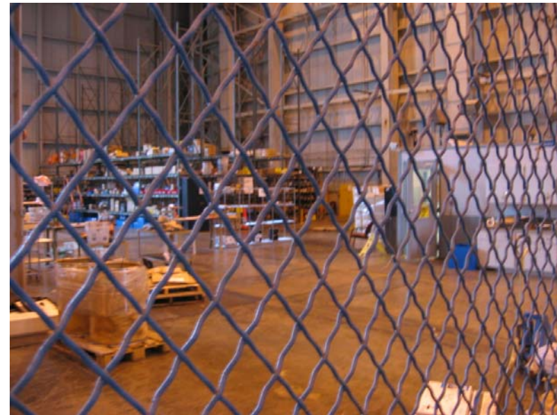
Existing racks along North/West Wall
