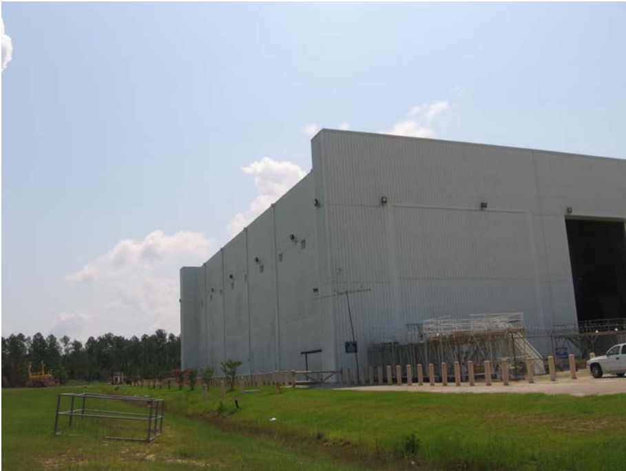
The north/west elevation of Building 3202 where the 10,714 square feet addition will be added.
