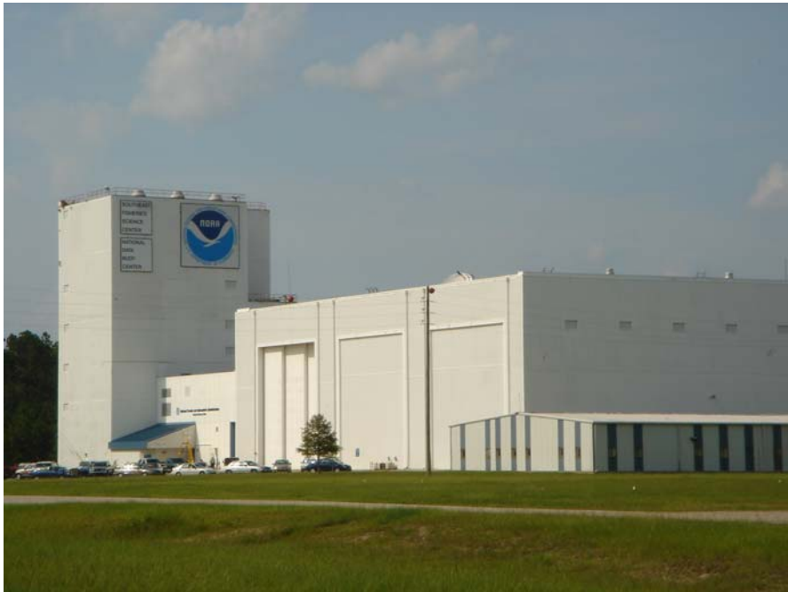
Building B3203 – West side
