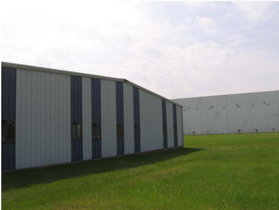
Existing west elevation. NOTE: Building 3202 in the background
