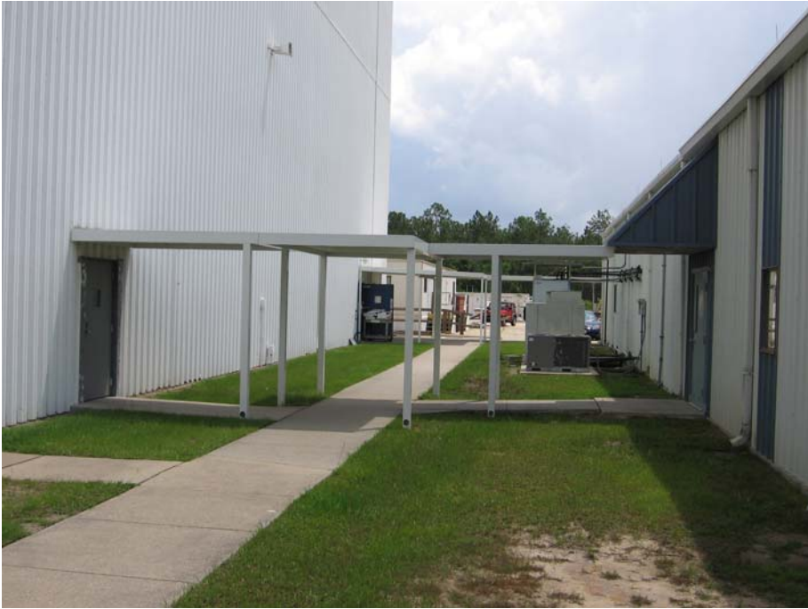
Walkway between Building 3205 and Building 3203
