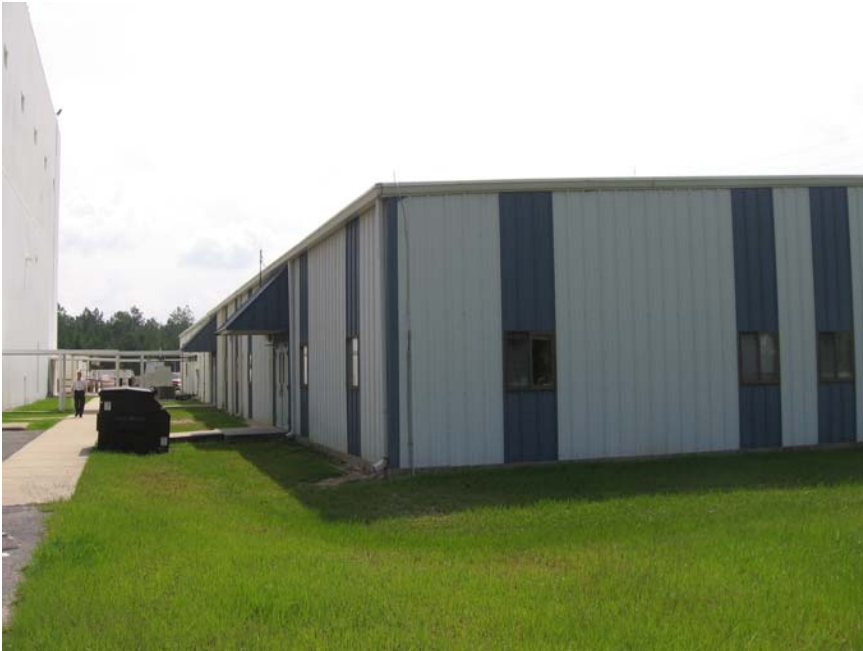
Building 3205 – North and West side
