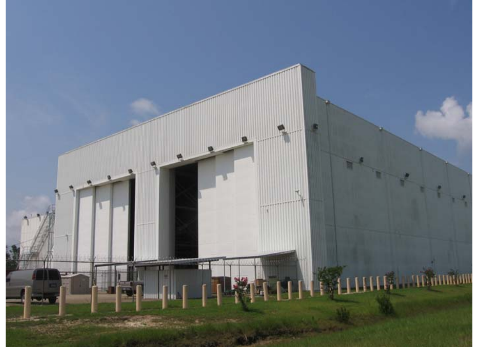
Building 3202 – North and East side
