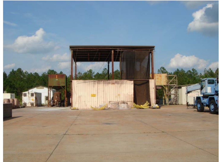
Building B3209 – West side
