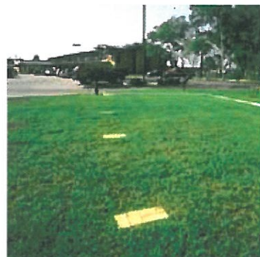
Bricks are embedded inside the Grasspave2 system to delineate spaces in this parking lot.
