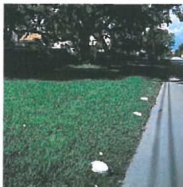
Reflective raised pavement markers delineate the parking spots in this Grasspave2 roadside parking lot.
