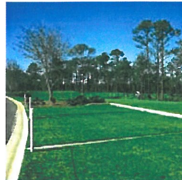
A concrete curb identifies the Grasspave2 access road on this golf course. A chain gate (left) prevents unauthorized travel over the reinforced grass road.
