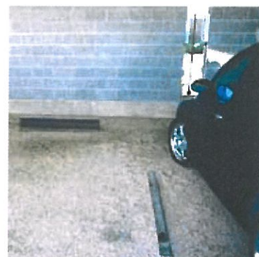
Metal markers are used in this Gravelpave2 parking lot to identify parking bays.
