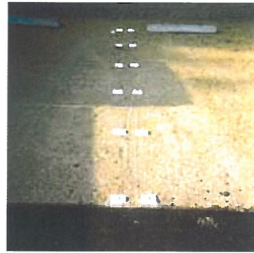
A combination of reflecting raised pavement markers and bumper stops line this Gravelpave2 parking lot. Asphalt drive aisle is shown in the foreground.
