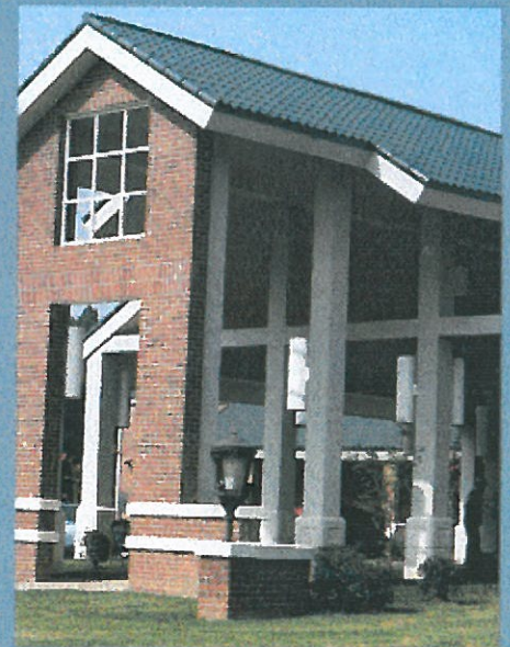
Slate Gray Met-Tile roofing was selected for a trio of Veterans homes.
