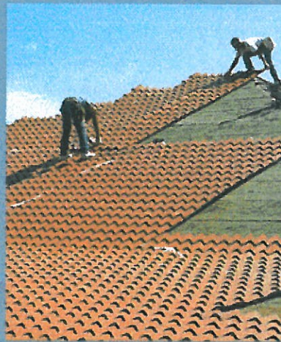
Met-Tile's long-length, cut-to-order tile panels install quickly and easily, with no truss reinforcement or batten grids required.
