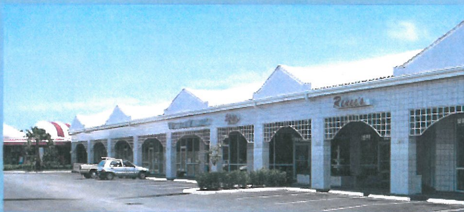
Met-Tile's high reflectivity makes it an energy-efficient choice. Panels in Cotillion White offer maximum energy and wind performance to this tropical shopping center.
