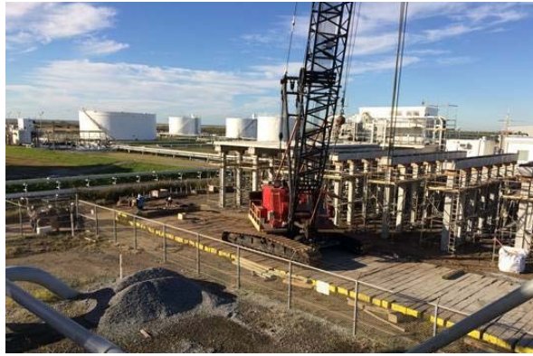
Figure 8-1: Example of a Waskey concrete deck.
