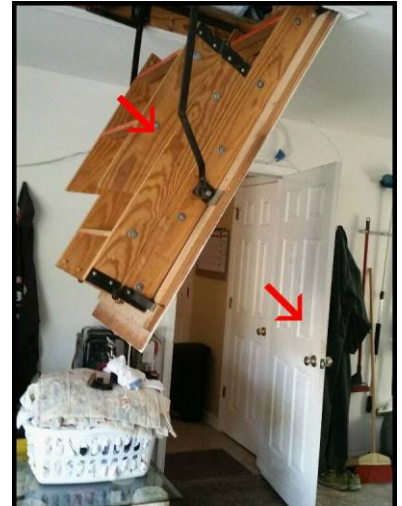
Not fire-rated: attic & house entry door
