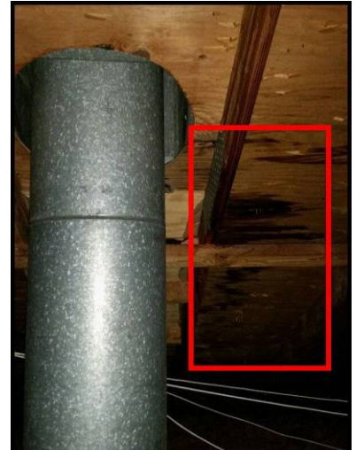
Evidence of past/present water stains
