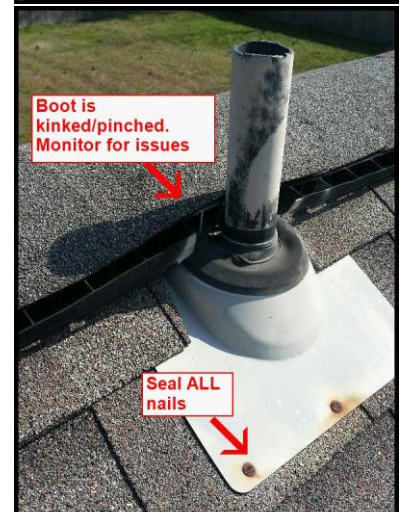
ridge vent presses on rubber boot. Monitor
