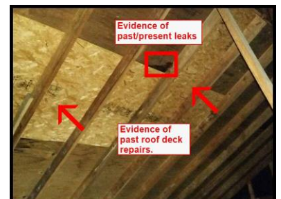
Main house attic
