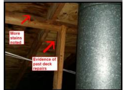
Evidence of past/present water stains
