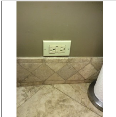
Repair: Outlet loose in the kitchen.
