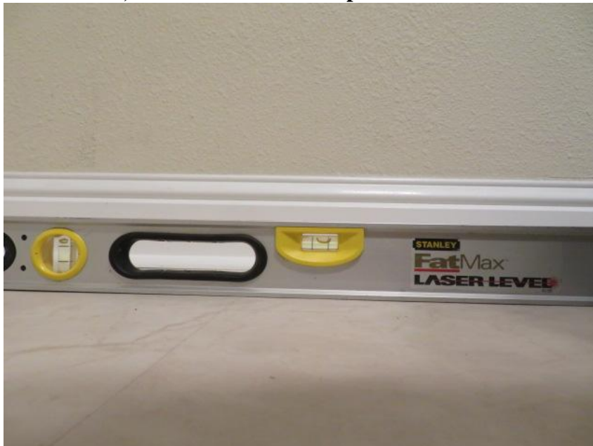
Picture #12, bathroom bubble - sloped toward exterior wall
