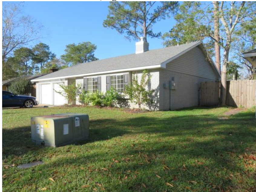
Picture #2, right front - affect area
