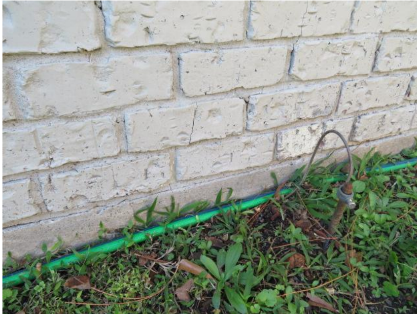
Picture #7, slab view - no cracks found
