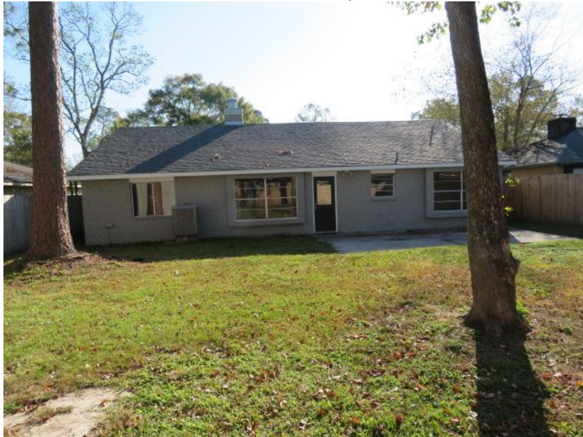
Picture #4, rear yard
