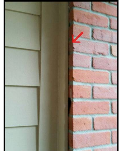
Caulk between all dissimilar material
