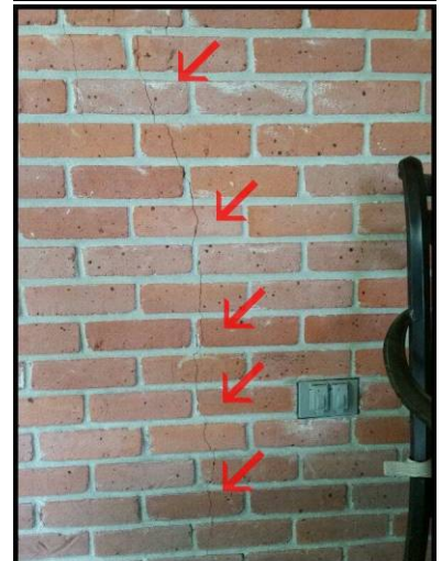
Side wall below patio
