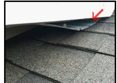
Zoomed in pic of loose soffit
