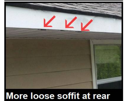
Zoomed in pic of loose soffit
