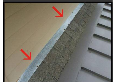
Seal ALL exposed nails
