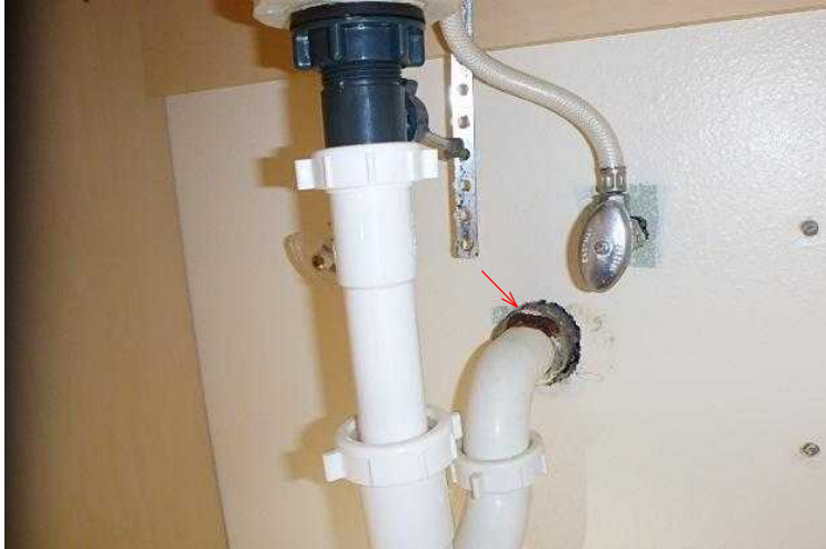
#97 Galvanized drain pipe in the wall.
