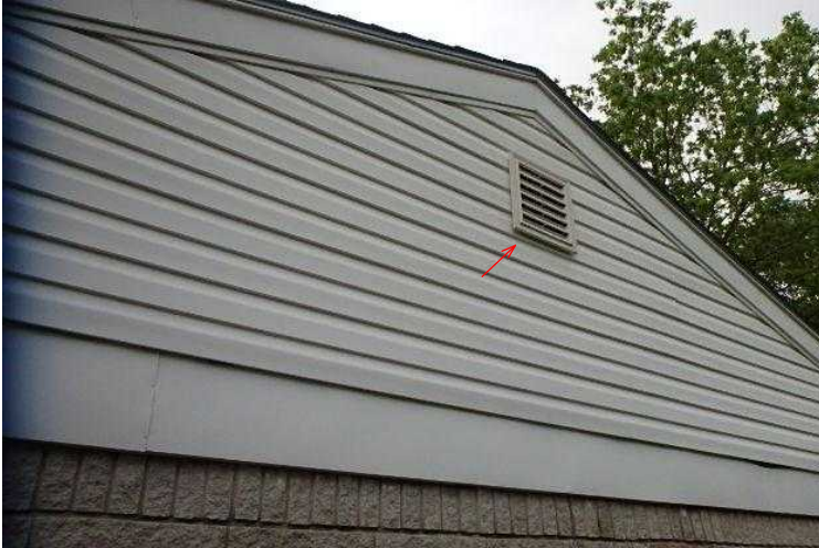
#13 Gable vents on each side.
