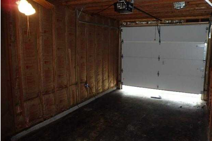
#53 Garage. Drywall removed and walls were insulated.
