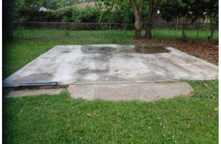
#18 Large slab on right rear.
