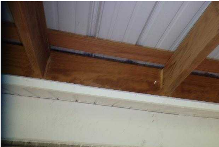
#51 Patio roof framing.
