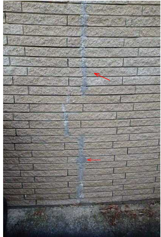
#14 Brick crack on the right side was filled with mortar.
