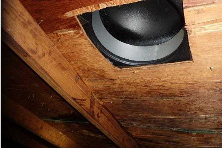
#113 Open vent over kitchen.
