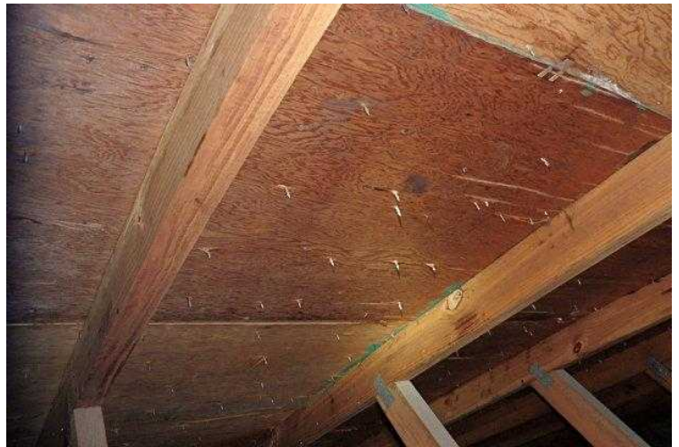
#108 Roof framing and sheathing.
