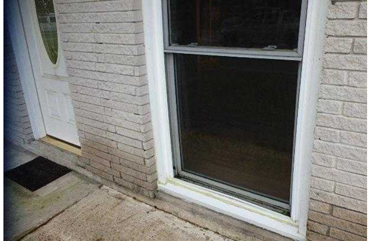
#10 Large window on the right front. Wood framing was probably removed.
