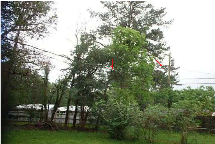
#19 Electrical service wires enter from the rear.
