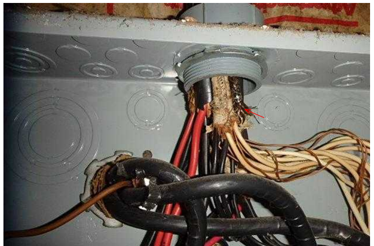
#64 Older cloth wrapped wiring.
