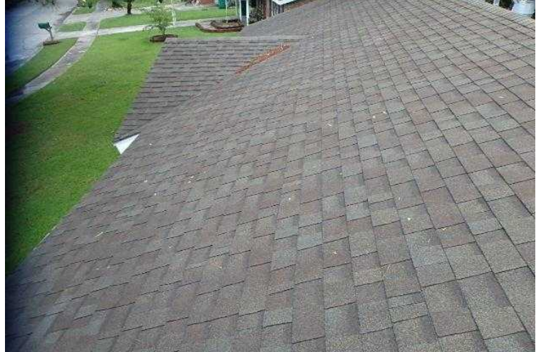
#38 Front roof view with center gable.
