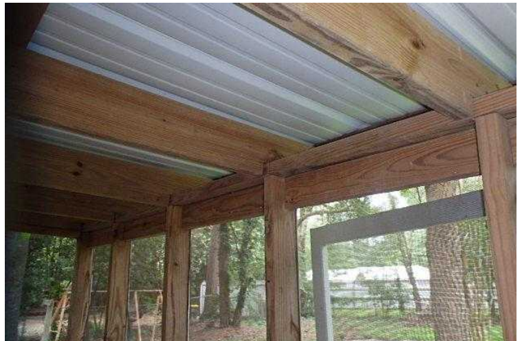
#52 Rafters rest on single top plate.
