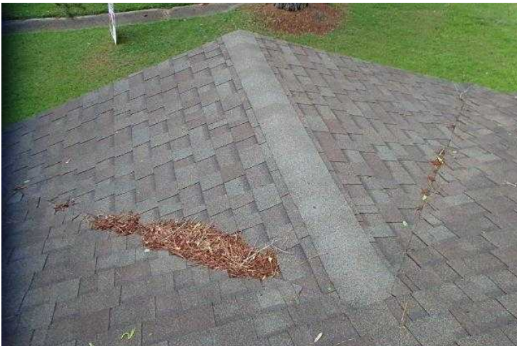
#39 Front gable and valleys.
