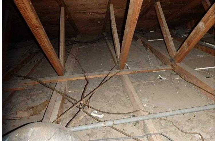
#106 Garage attic. 2x4 roof trusses. The walls in the garage are insulated but not the ceiling.
