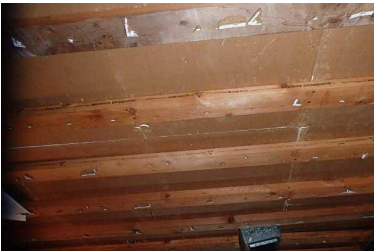
#55 Ceiling drywall removed.
