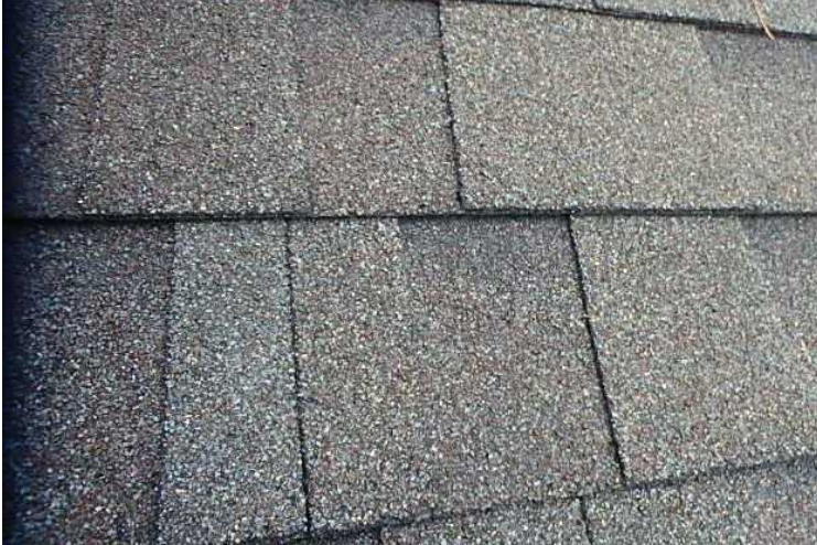
#37 Roof shingles. No granule loss noted.
