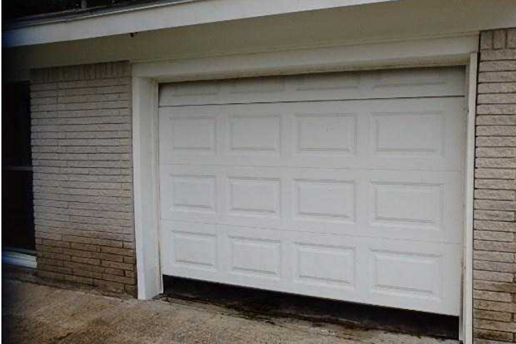
#9 Right front garage door.
