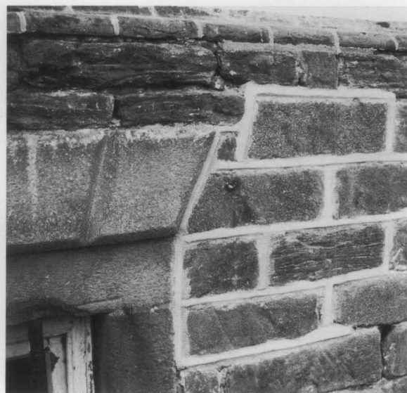
Figure 4. (left) The poor quality of this repointing—it appears to have been “tooled” with the mason’s finger—does not match the delicacy of the original beaded joint on this 19th-century brick wall. (right) It is obvious that the repointing on this “test patch” is not an appropriate replacement mortar joint for this early-19th century stone foundation. Photos: Lee H. Nelson, FAIA.
