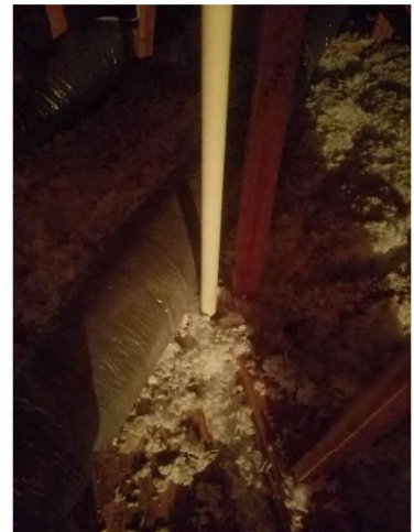
This roof support is supported by the end of the Island Wall
