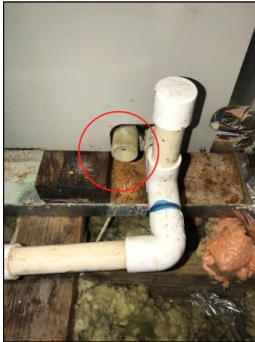
64. Poor termination
