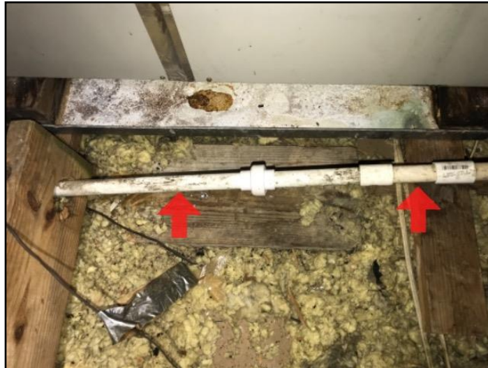
67. Missing insulation
