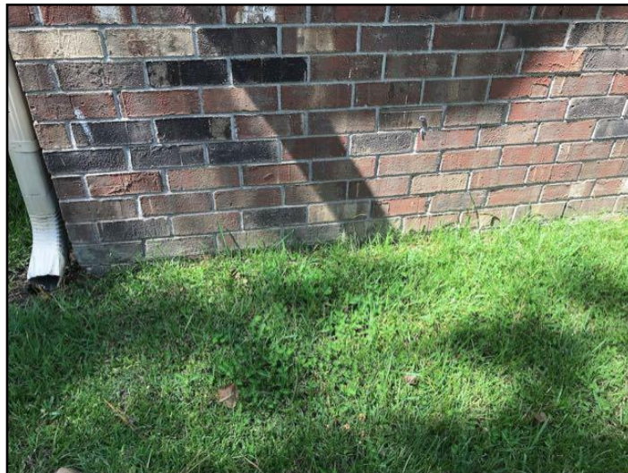
34. High soil at slab
