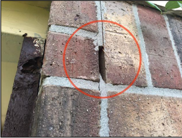
26. Mortar deterioration
