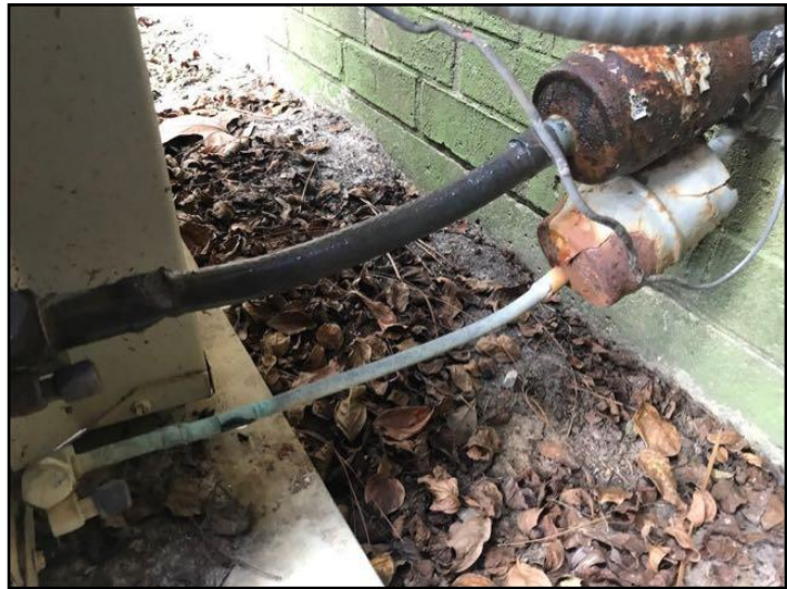
69. Insulation - missing
