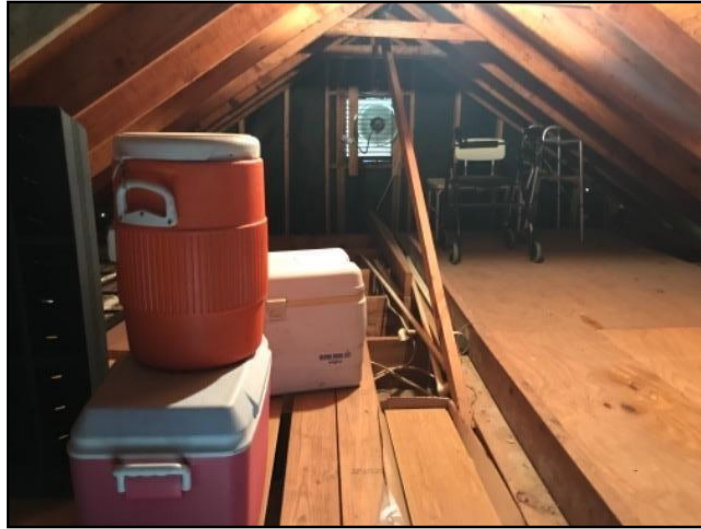
35. Storage in attic
