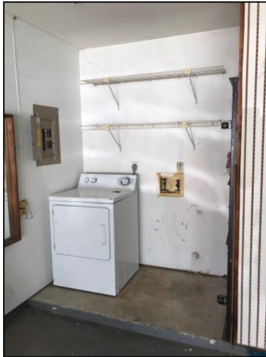
91. Located at garage
