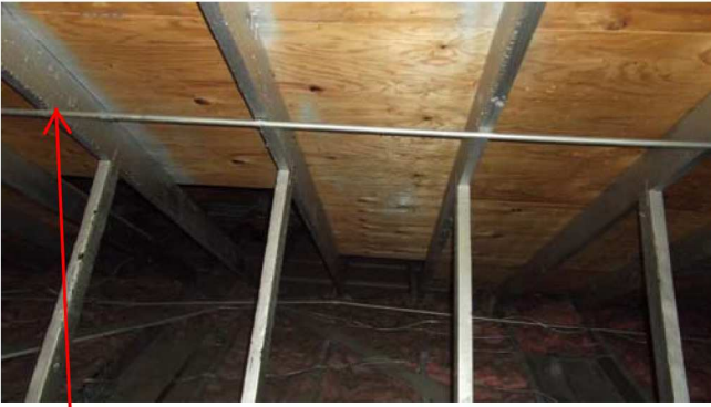
Roof framing members that have been painted.
