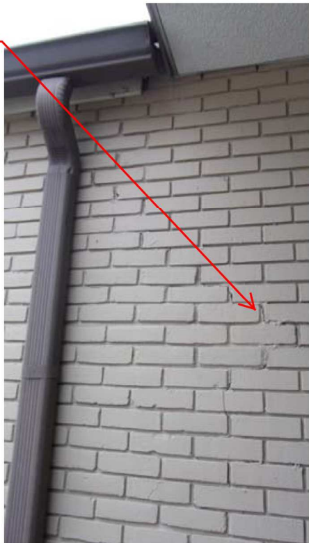
Crack in brick veneer.
