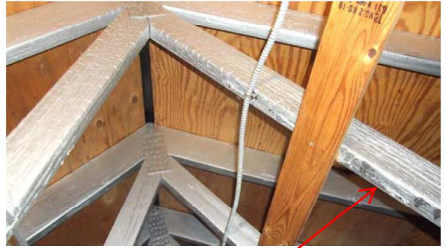
Roof framing members that have been painted.
