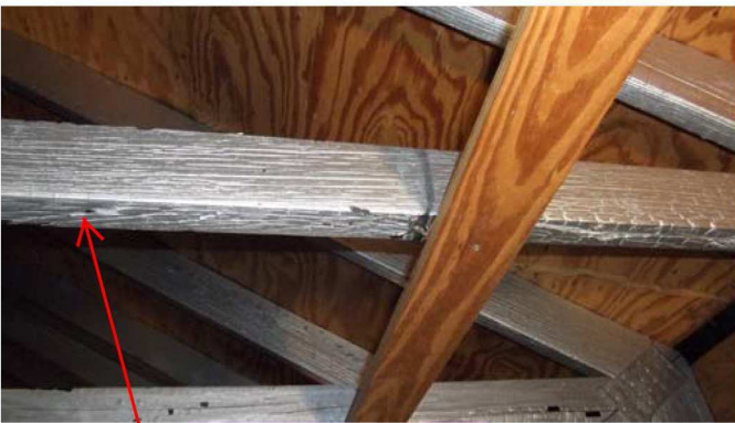
Roof framing member that has been painted.
