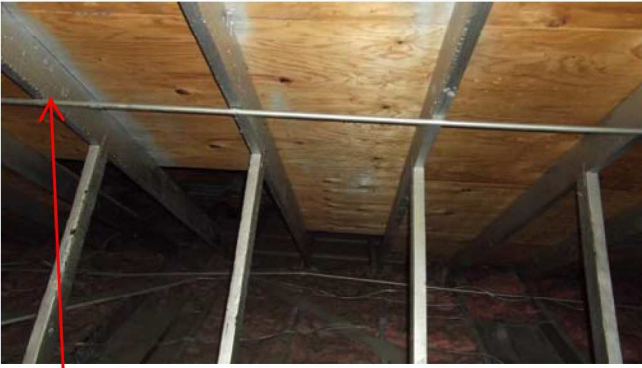
Roof framing members that have been painted.
