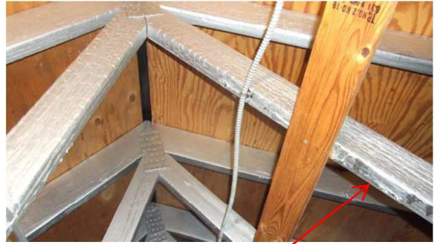
Roof framing members that have been painted.
