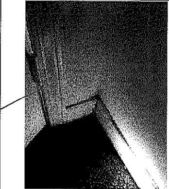
Repair: Master closet wall water damaged.
