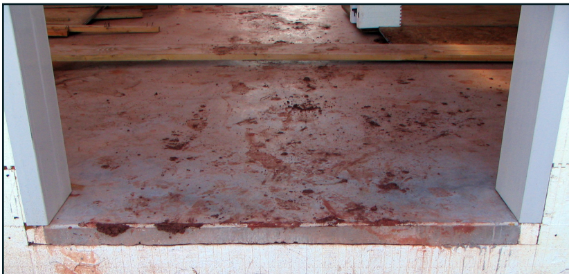
Note the concrete threshold poured to the outside wall edge.
