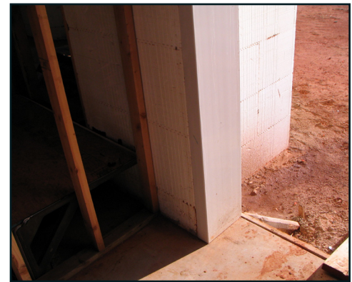
Note the concrete threshold poured to the outside wall edge.
