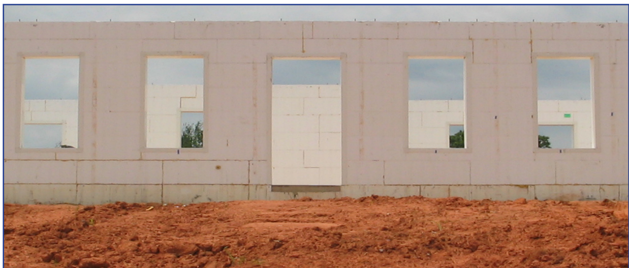
Clean and neat window and door openings.
