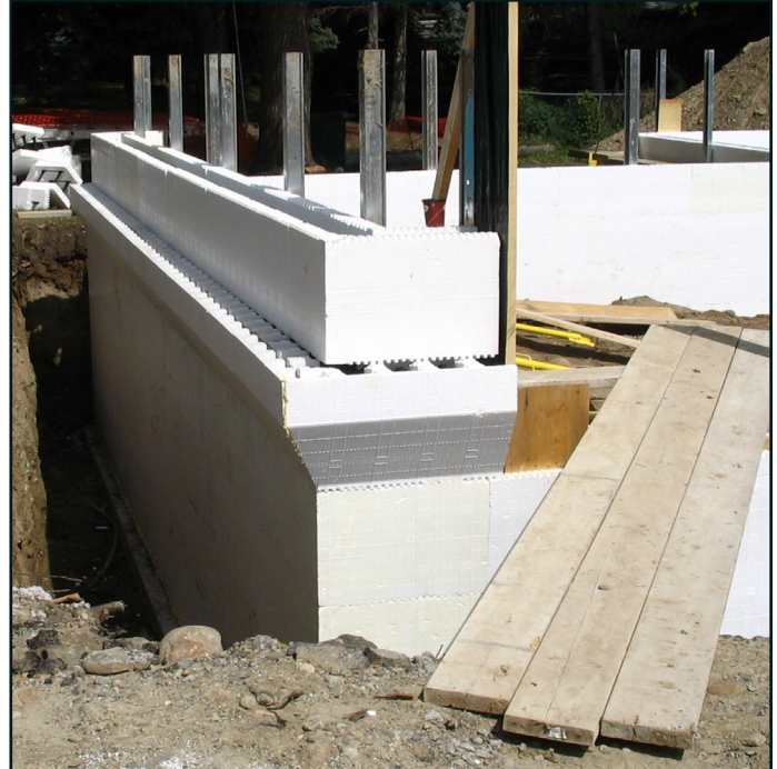
6" Buildblock Form Placed Over the Brick Ledge Form
