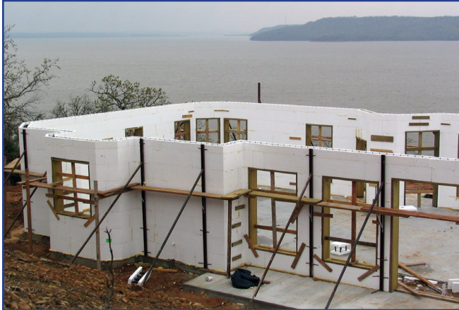
Minimal Outer Bracing
