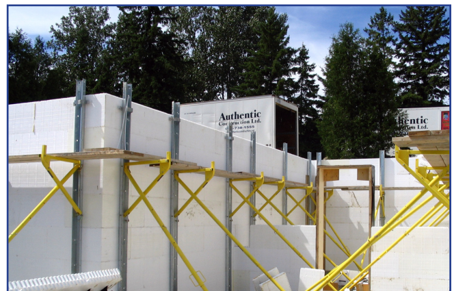
More Secure Inner Bracing w/ Walk Board
