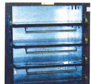
Adjustable Dampers at each deck
