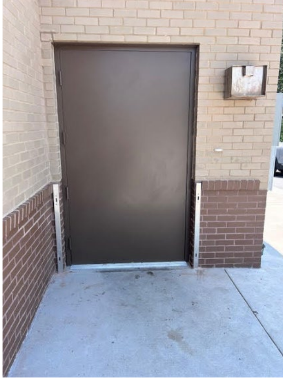
Door 3 Rear Service without Flood Barrier August 09/2024
