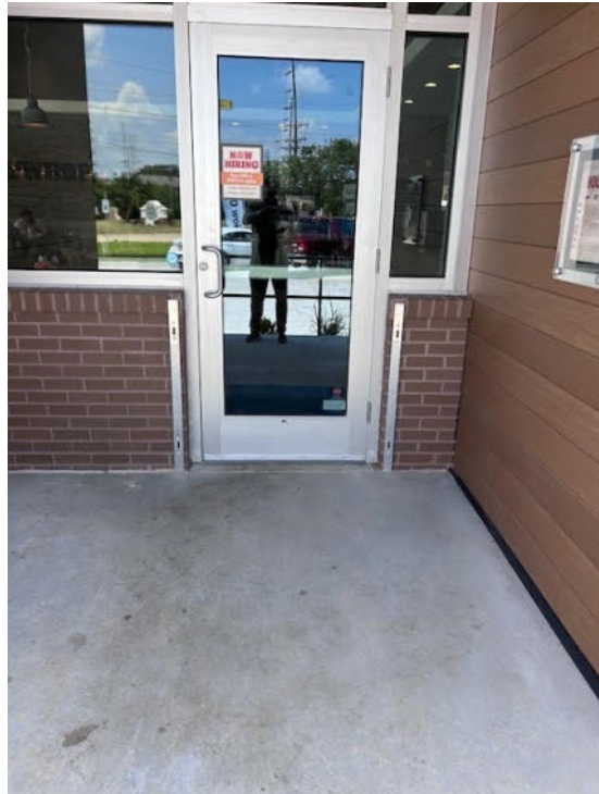
Door 1 Side Main Entry without Flood Barrier August 09/2024
