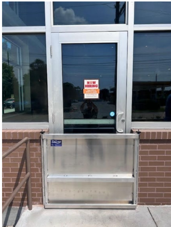
Door 2 Front Entry with Flood Barrier August 09/2024
