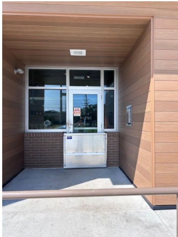
Door 1 Side Main Entry with Flood Barrier August 09/2024
