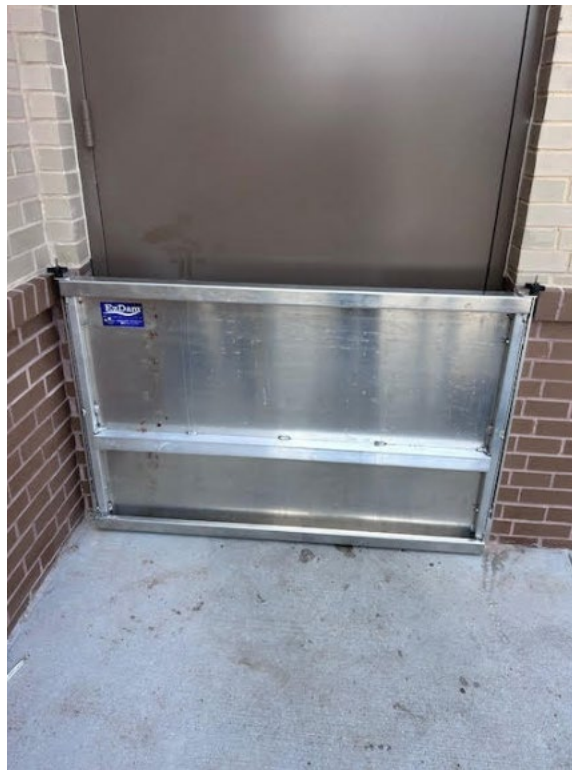
Door 3 Rear Service with Flood Barrier August 09/2024
