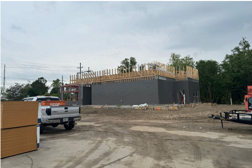
Main Side Entry / Rear Elevation April 8/2024
