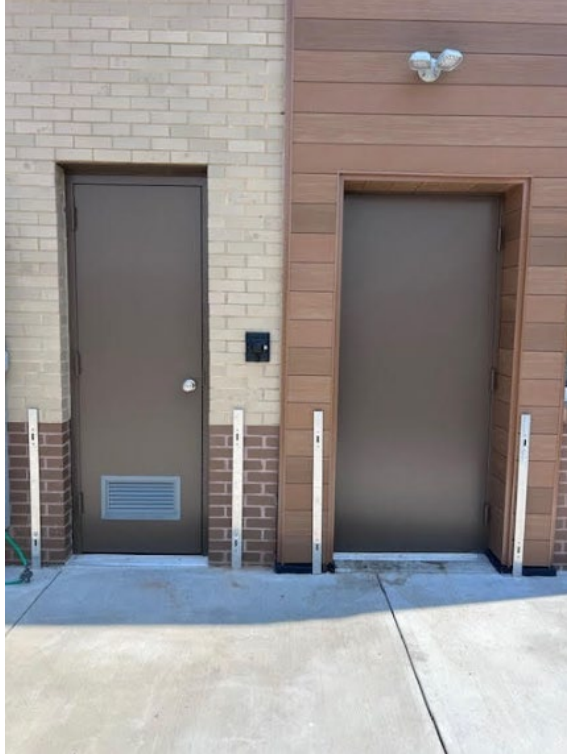
Door 4 Bulk CO2 Room Rear Elevation without Flood Barrier August 09/2024
