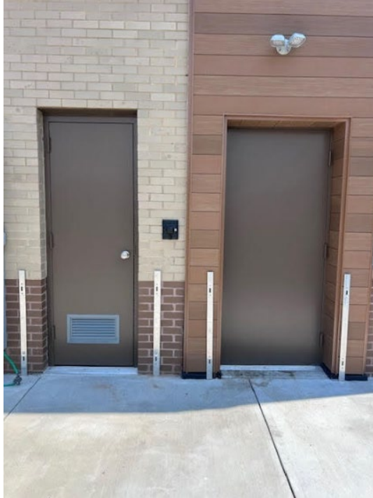
Door 5 Drive Thru Pay Rear Elevation without Flood Barrier August 09/2024
