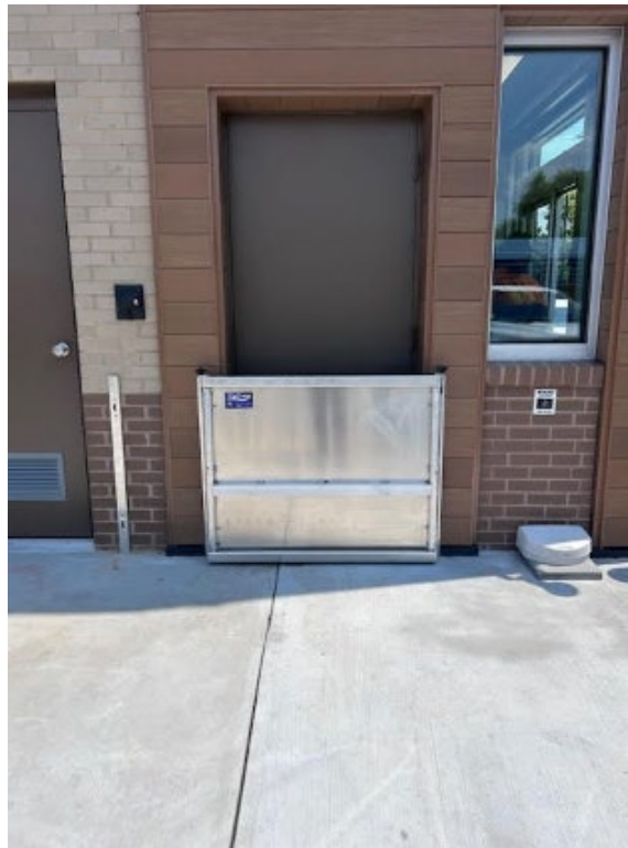
Door 5 Drive Thru Pay Rear Elevation with Flood Barrier August 09/2024
